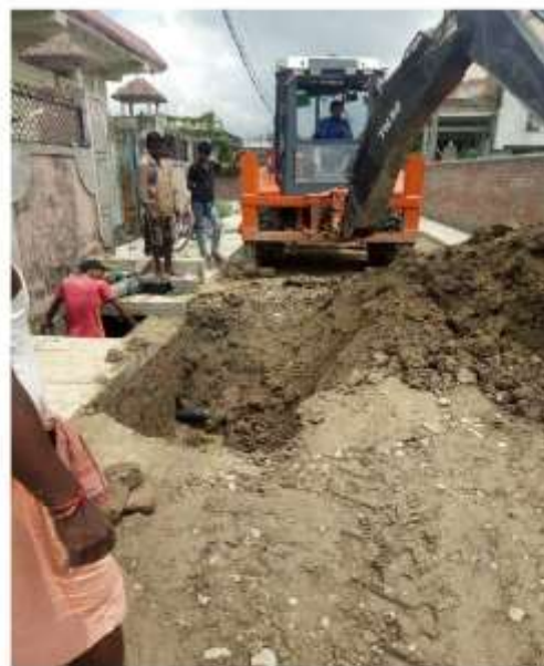
Excavation for house connection
