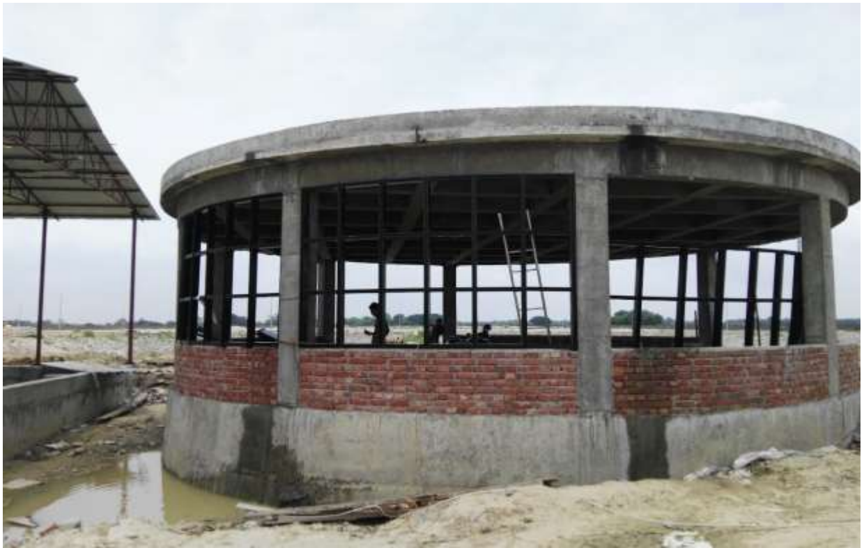
A view of sump well
