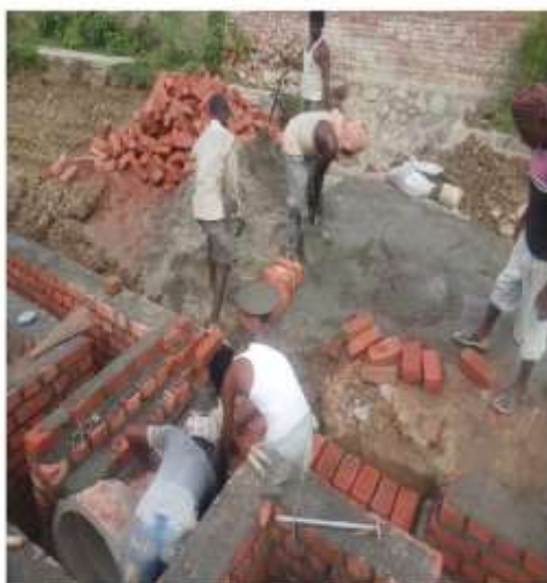
Catchpit Construction in WWTP
