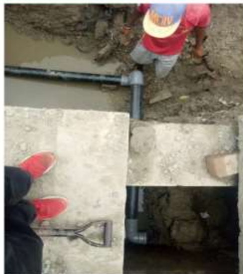
House connection at Dharambad Road
