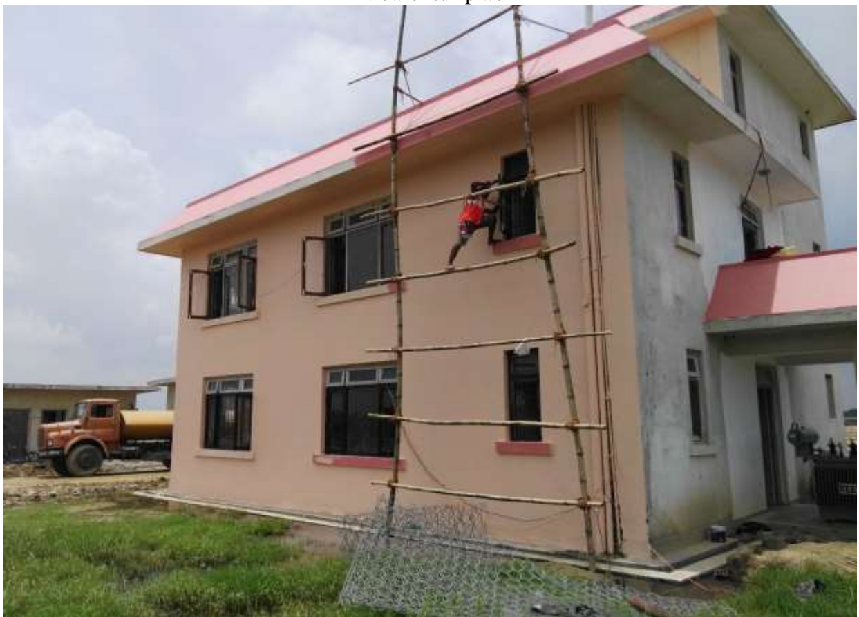
Painting work is progressing at Lab building, WWTP, Jatuwa
