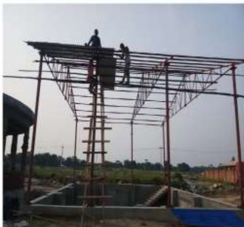
Placing of panels above the Bar Screen Chamber
