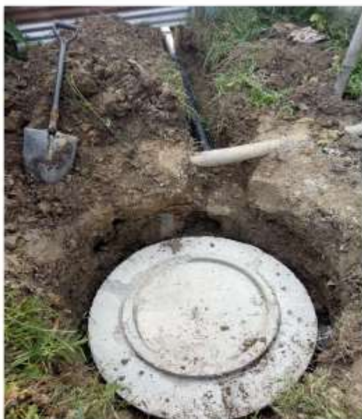
Placing of Sewer Inlet
