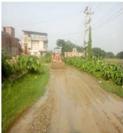
Road Maintenance at R-4
