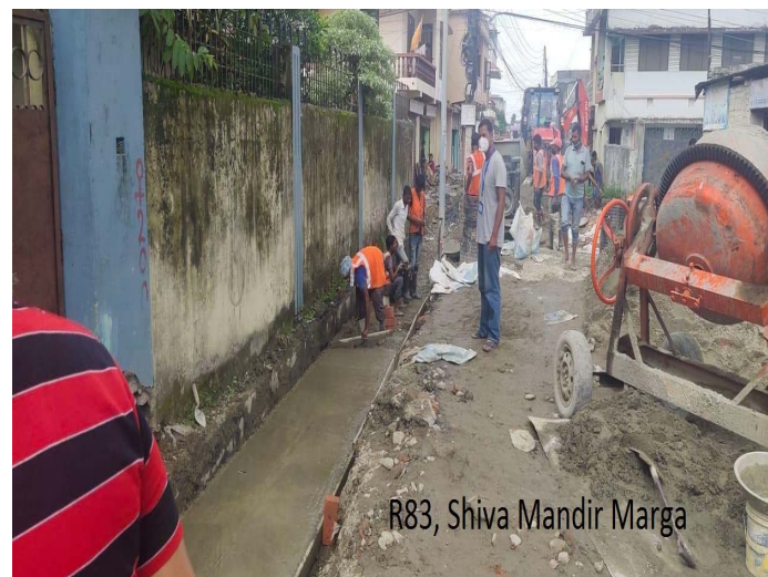
Drain foundation PCC work at shiv mandir marga
