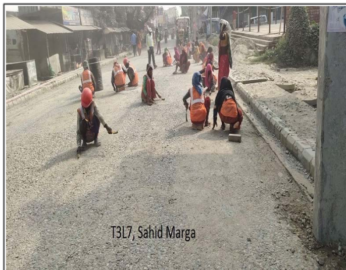
Road cleaning for to spread Asphalt in Sahid marga
