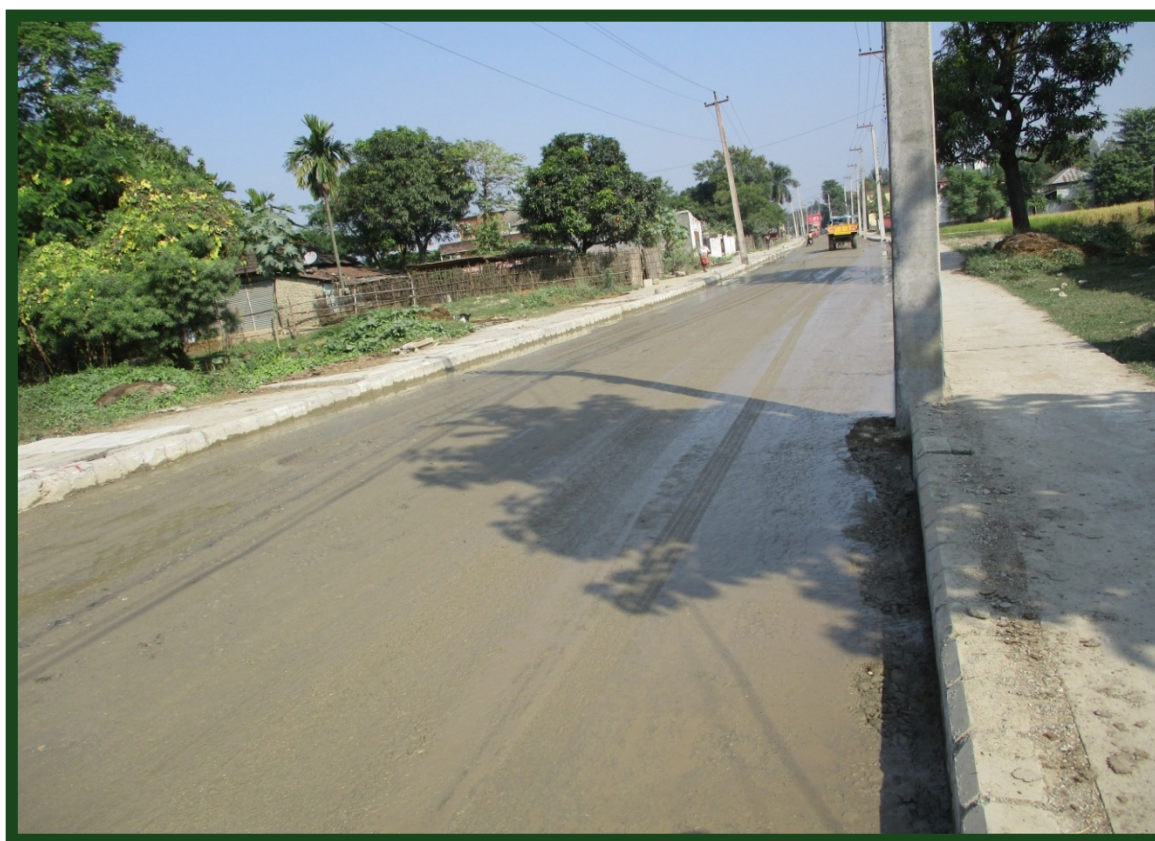
Subbase final works at R3
