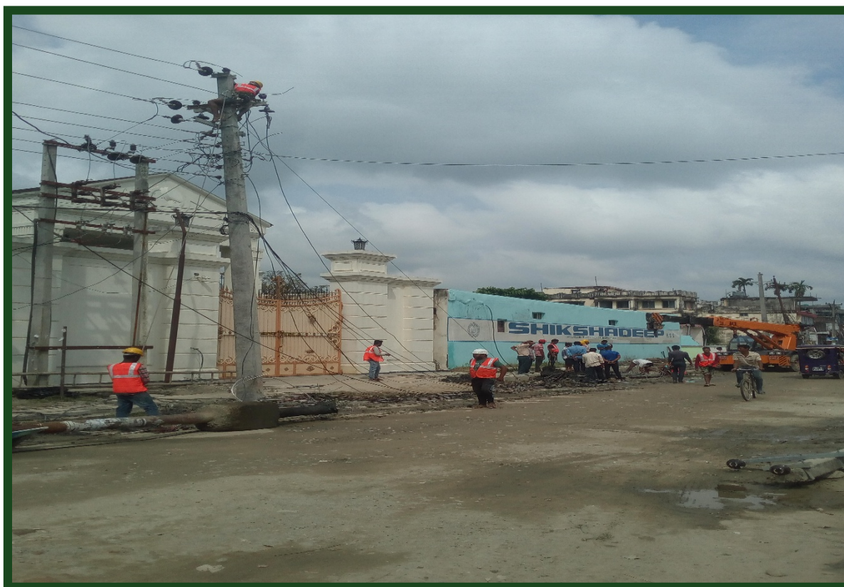
Relocation of Electric poles at R2
