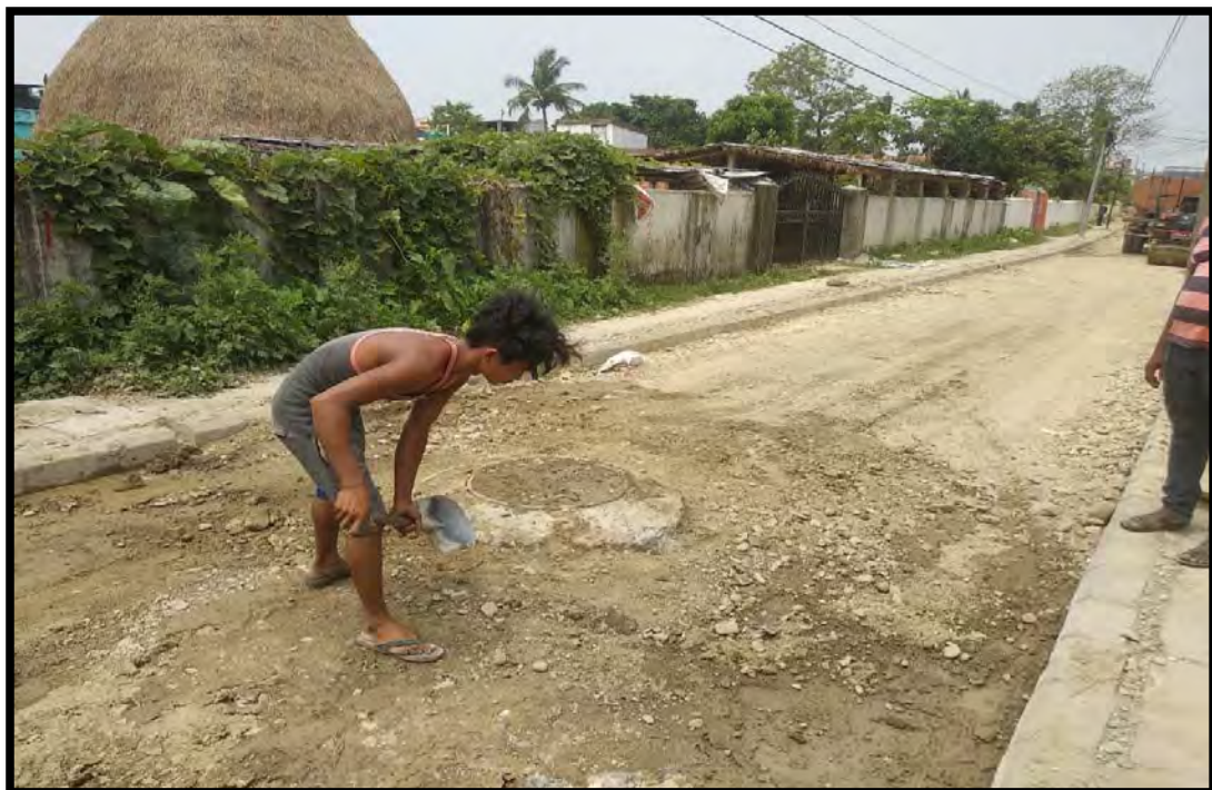
Re adjustment of Sewer manhole wrt the required gradient
