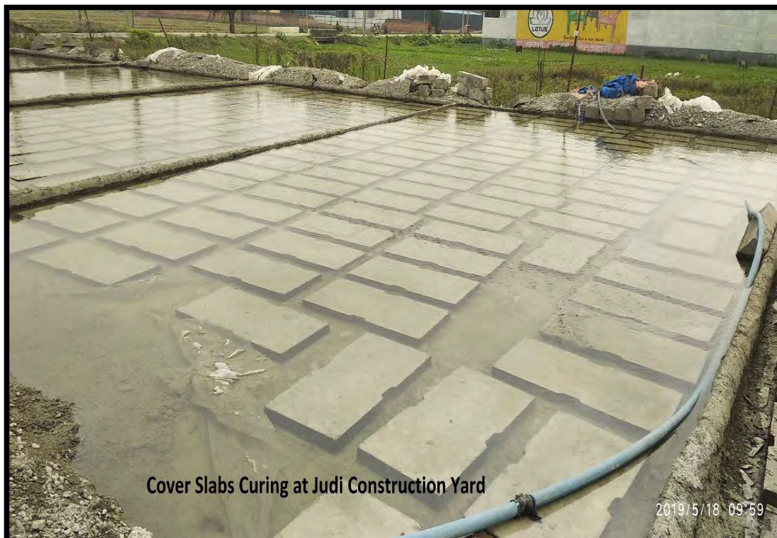
Curing of precast elements at Contractor's yard
