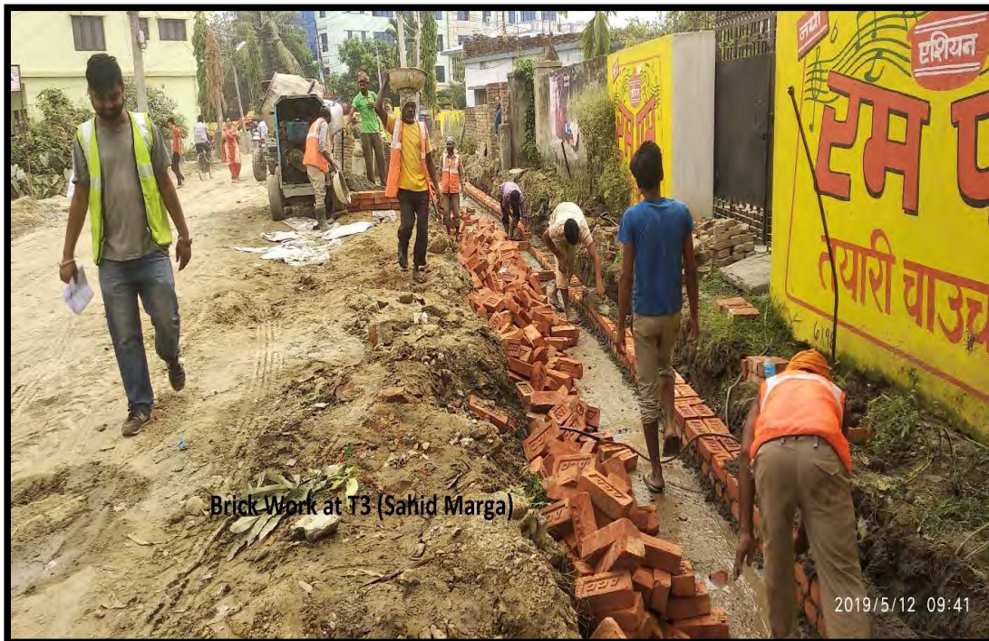
Brick work for road side drain at T3 Trunk (Sanihaat to Tapariya eye Hospital)
