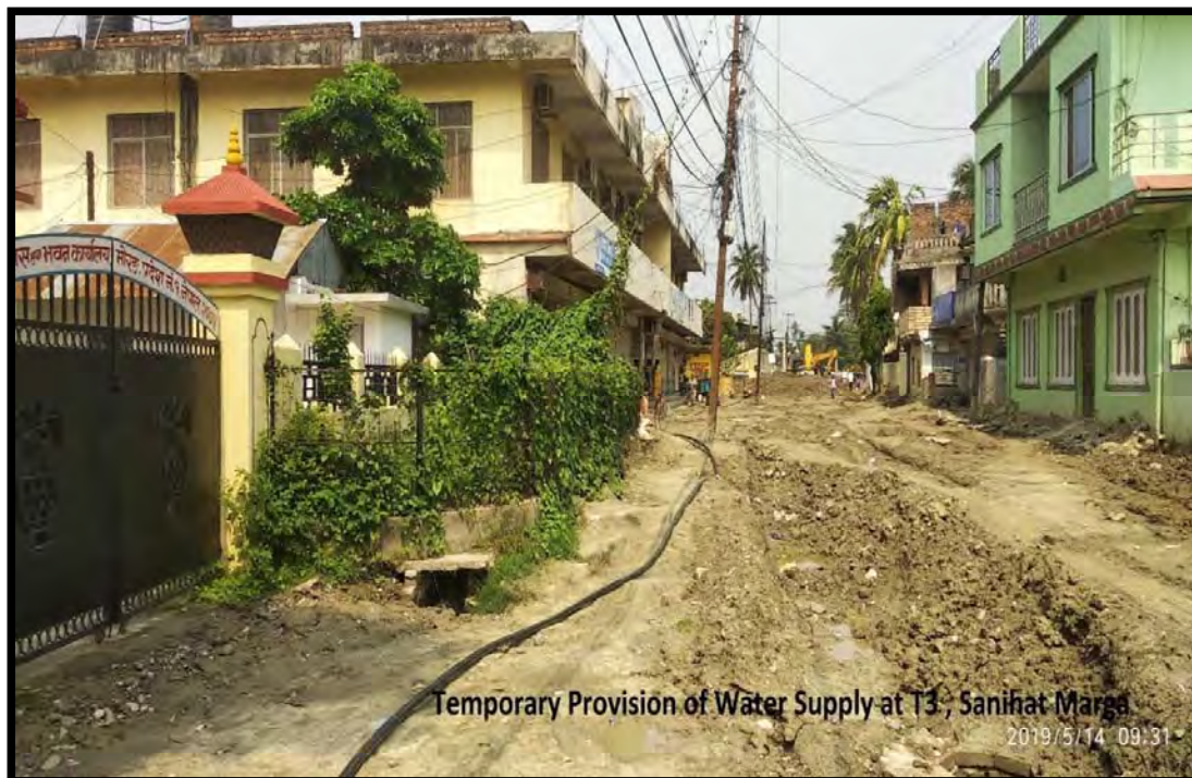
Temporary water supply HDPE 40mm pipes
