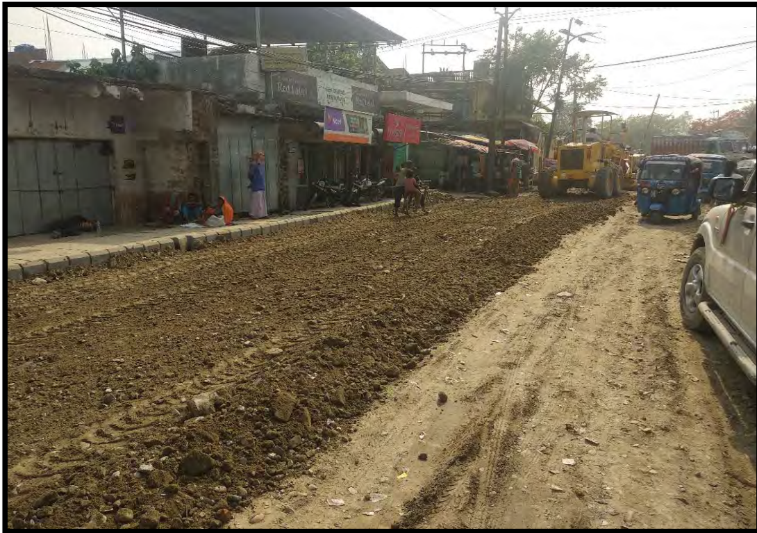
Laying of Base in T3 Trunk
