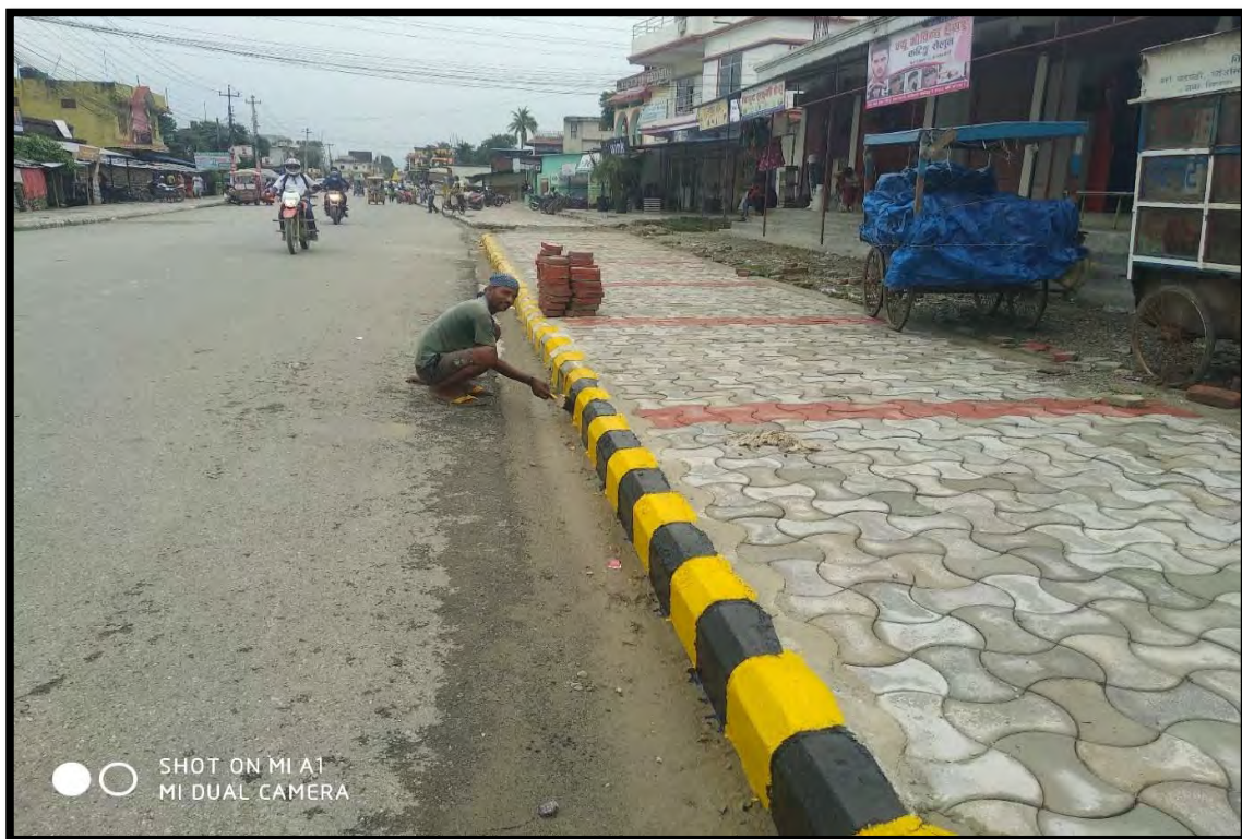
Interlocking work on footpath – B1
