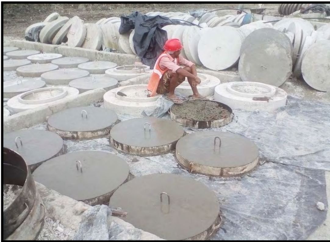
Pre cast top cover slab for HCC at Madhumara Yard
