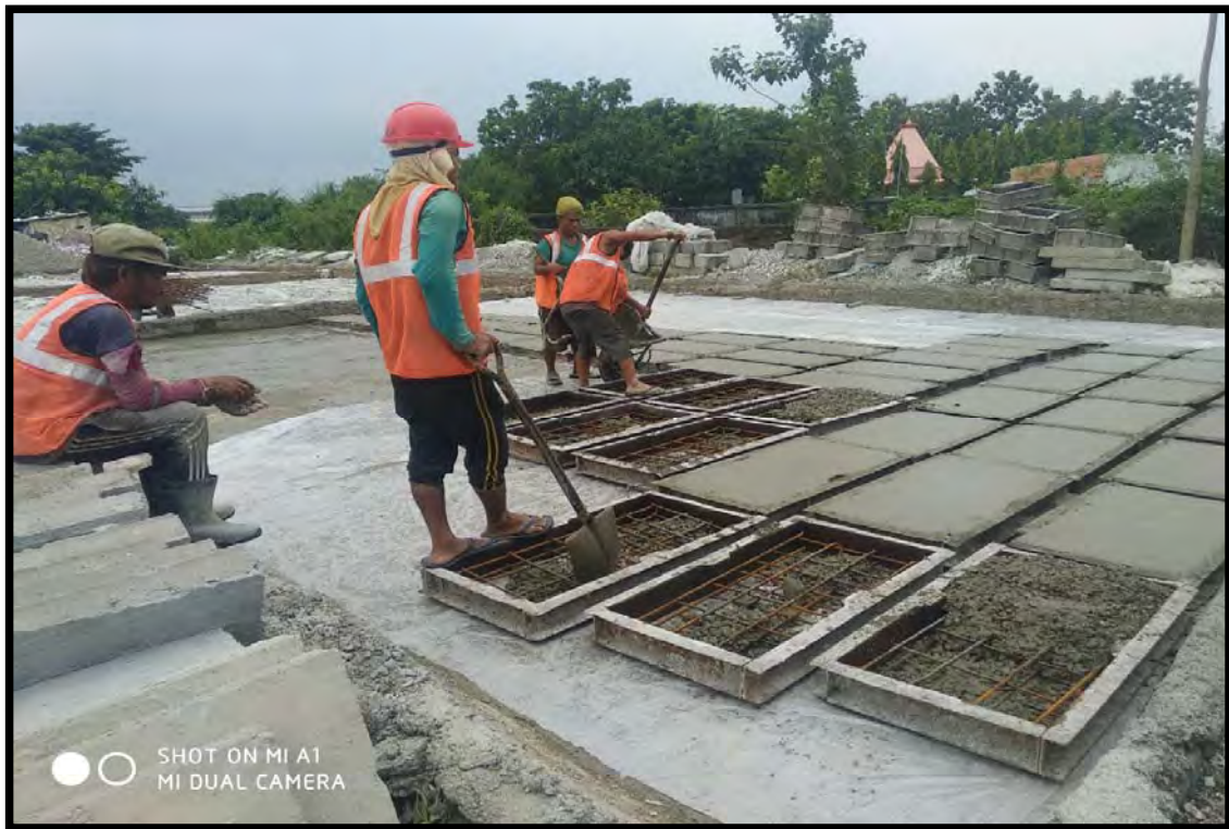
Pre cast slab casting at Madhumara Yard
