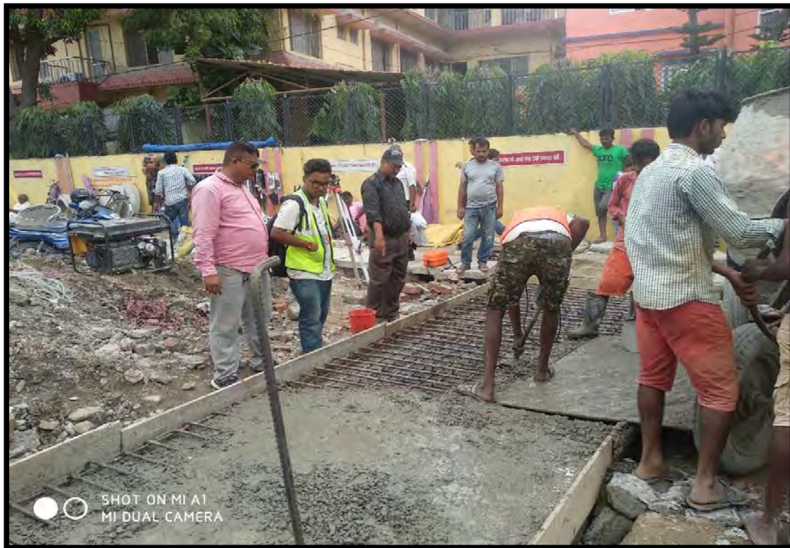
Laying of concrete for crossing slab at R2 – Main road
