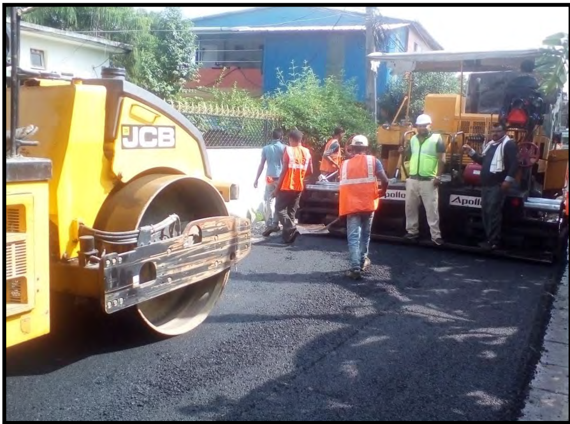
Asphalt work at T2L19Q
