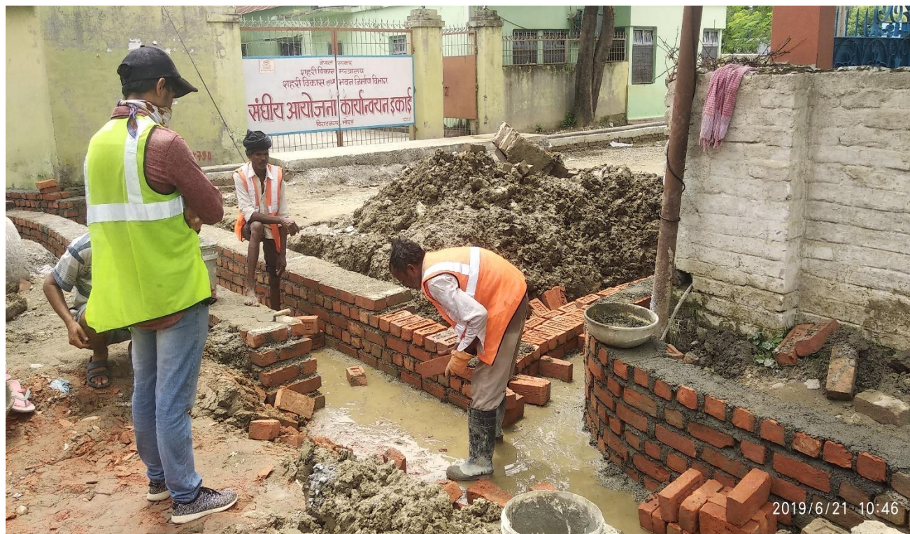
Road side Drain work at T3 Trunk – DUDBC Office, Biratnagar
