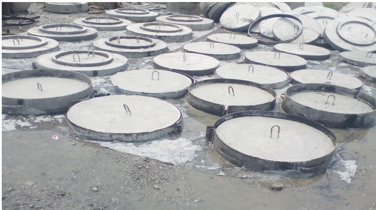
Curing of precast elements at Contractor's yard
