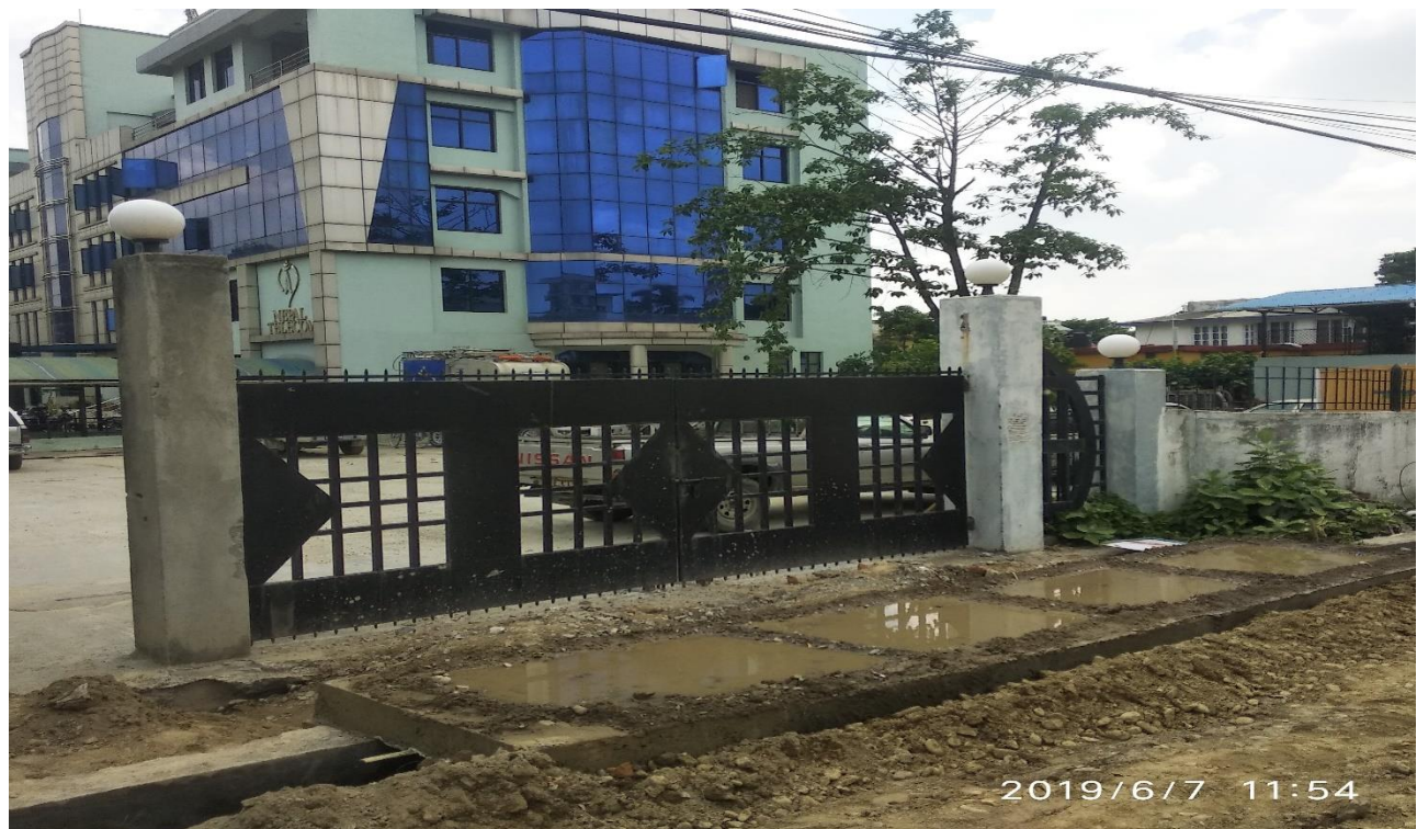
Dewatering work at T3 Trunk – Road side drain & crossing
