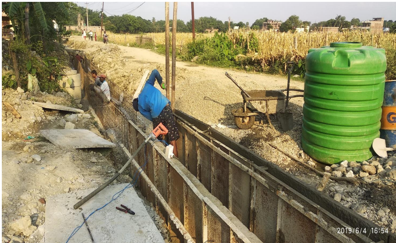
RCC Road side Drain at R4
