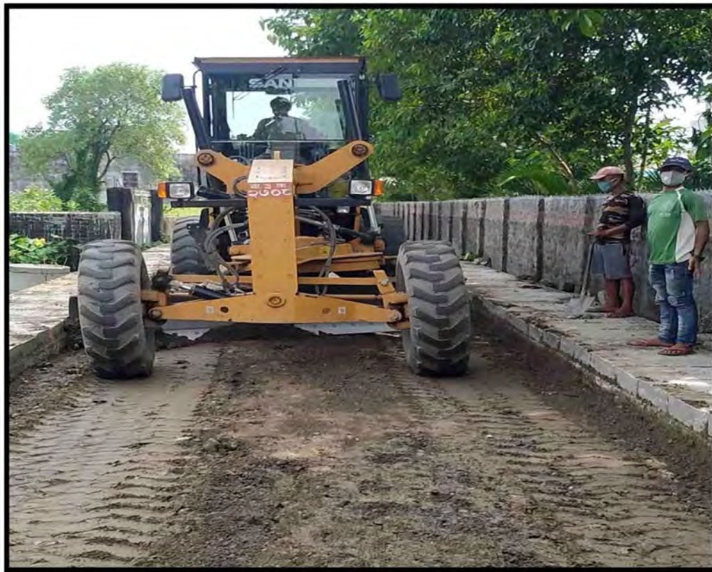
Subgrade preparation work at T2Line19K (Sudhaar Marga)
