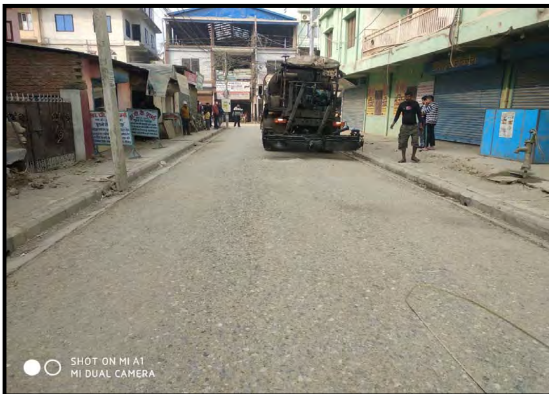
Road Surface prepared for prime coat application at T3L10C
