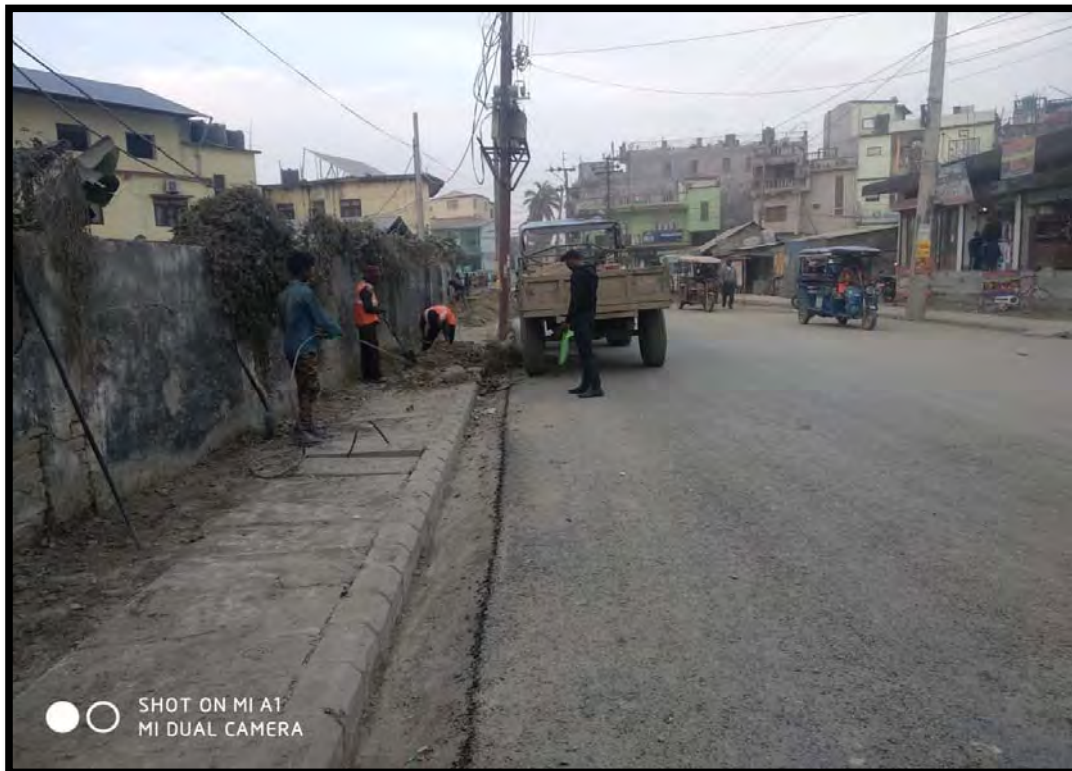
Backfilling work for footpath at R44
