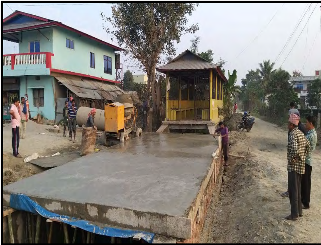
Completion of road crossing slab concreting at S13
