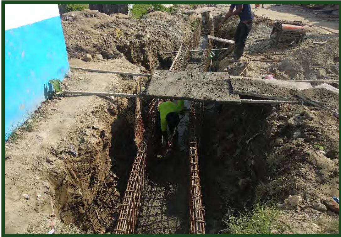
RCC Drain works at R6
