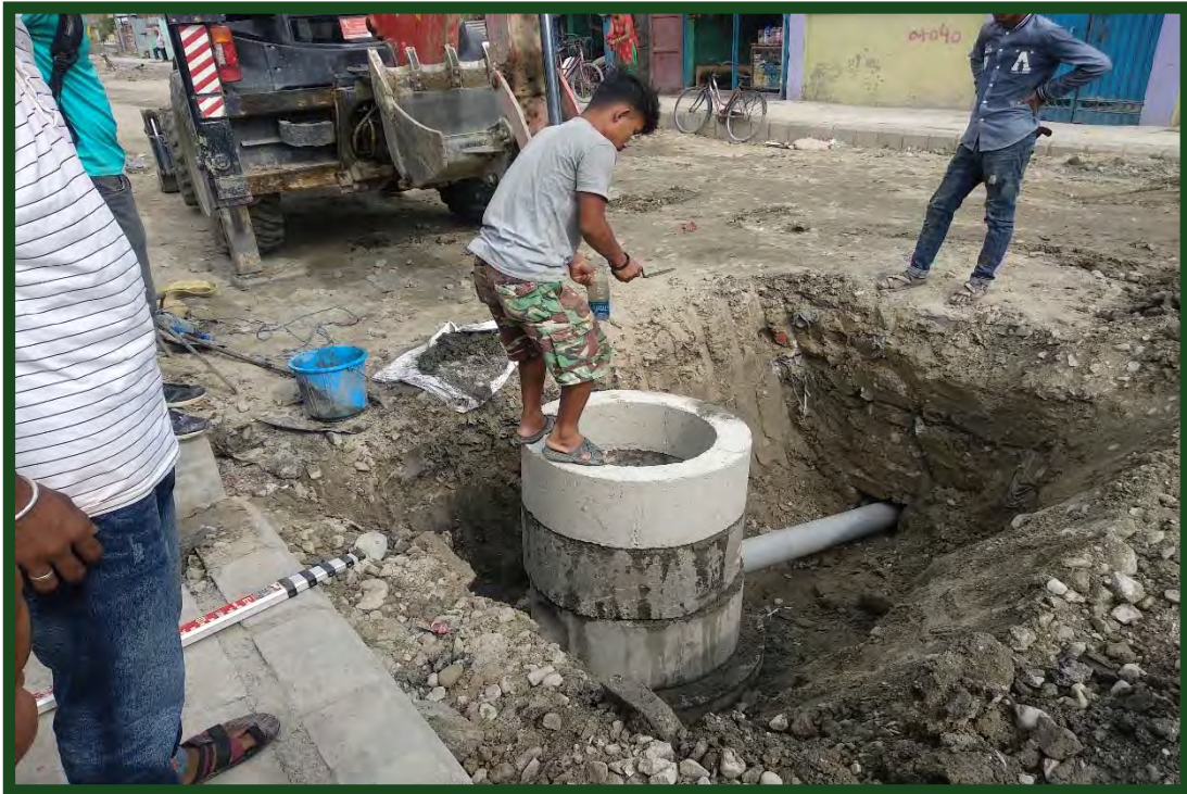
Sewer inlet works at R63 (DSP Road)
