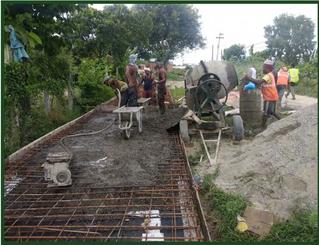
Concreting of Top Slab at Chyangbari Nala
