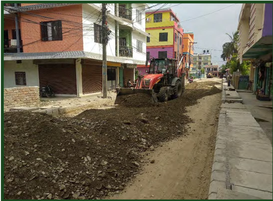
Sub base work at T1L16B (Xenial Front)
