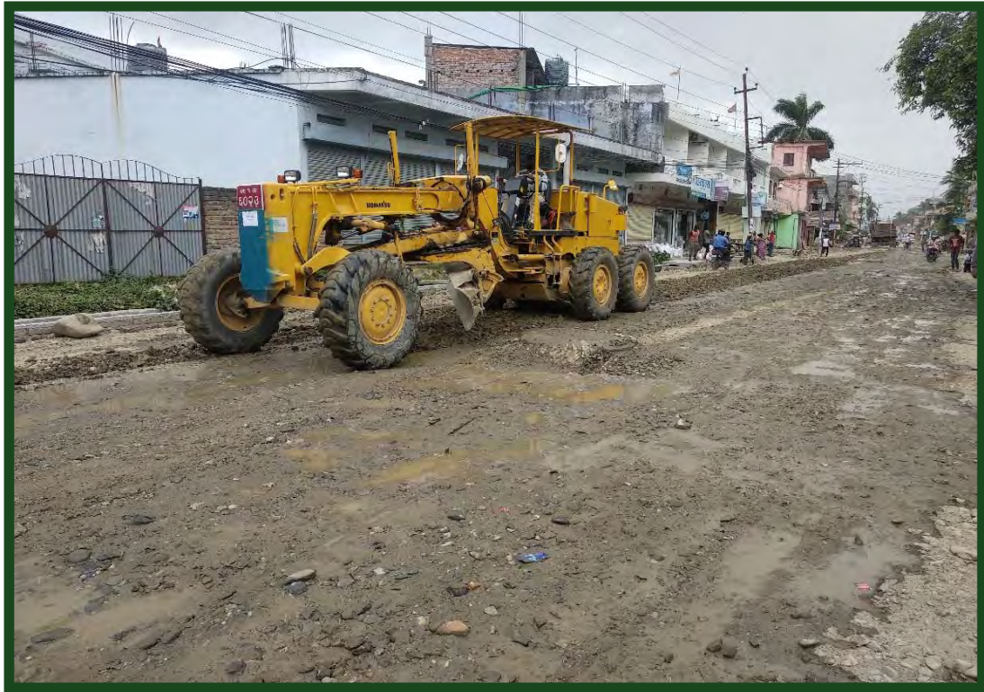
Subbase work at R2
