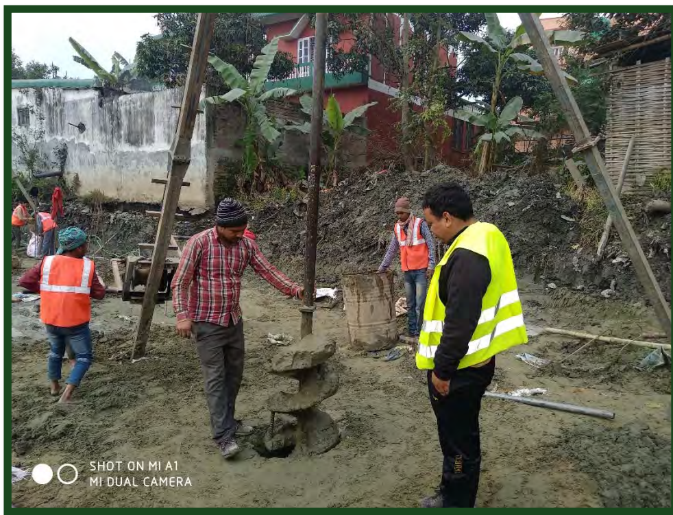
Pile Foundation works at Chyangbari Nala (CN3-CN2)
