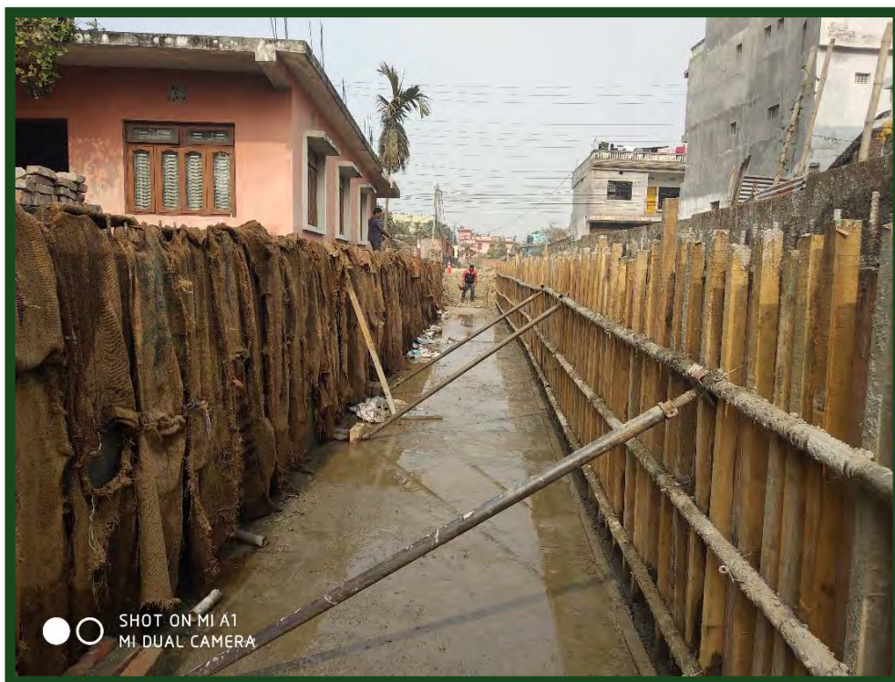
Shear Wall Construction (Chyangbari Nala)
