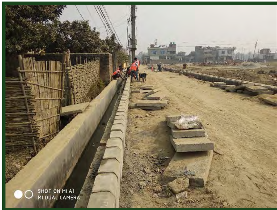
Kerb stone laying works at R29
