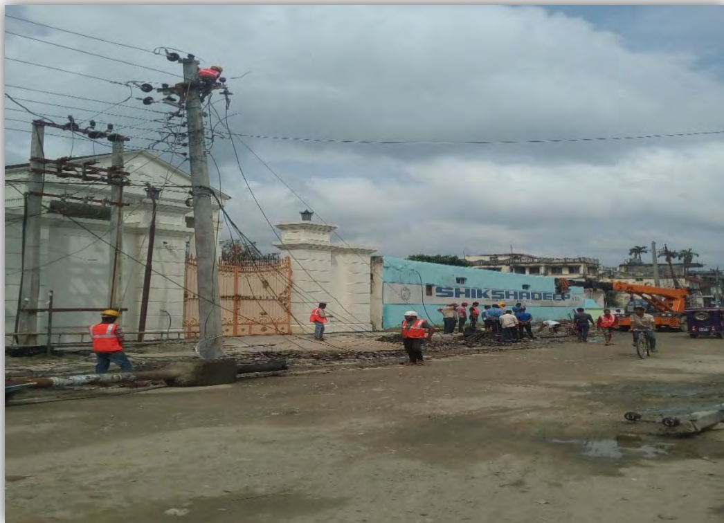
Relocation of Electric poles at R2
