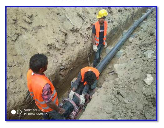
HDPE pipe 200mm dia laying at sewer line T4 Line 1
