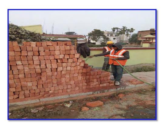
Water sprinkling on brick before laying (R18)
