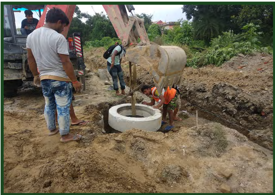
Sewer inlet works at T4 Line 1
