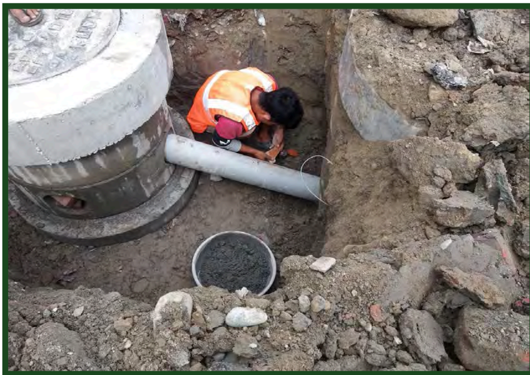
Sewer inlet works at R2
