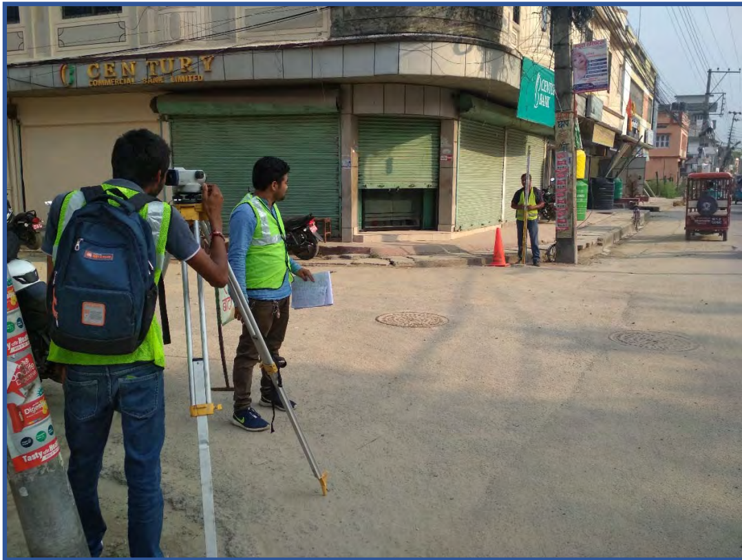
Survey works for sewer line
