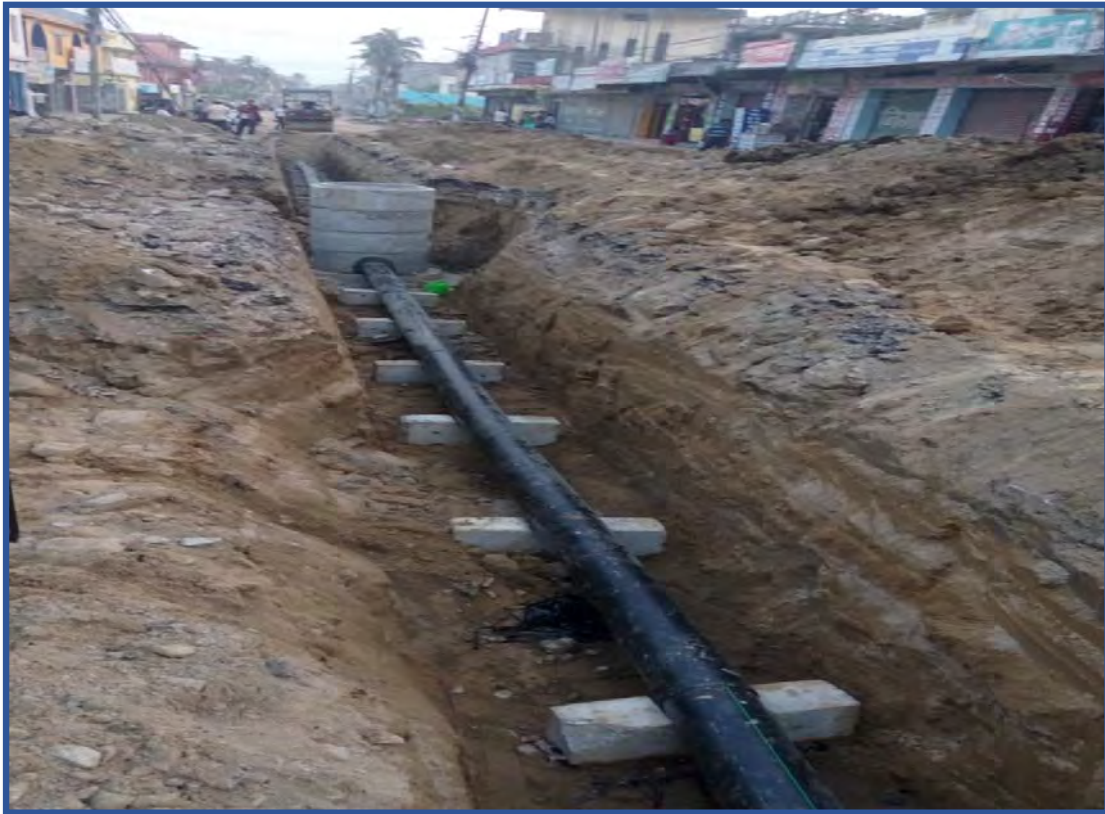
Sewer line works at T4 Line
