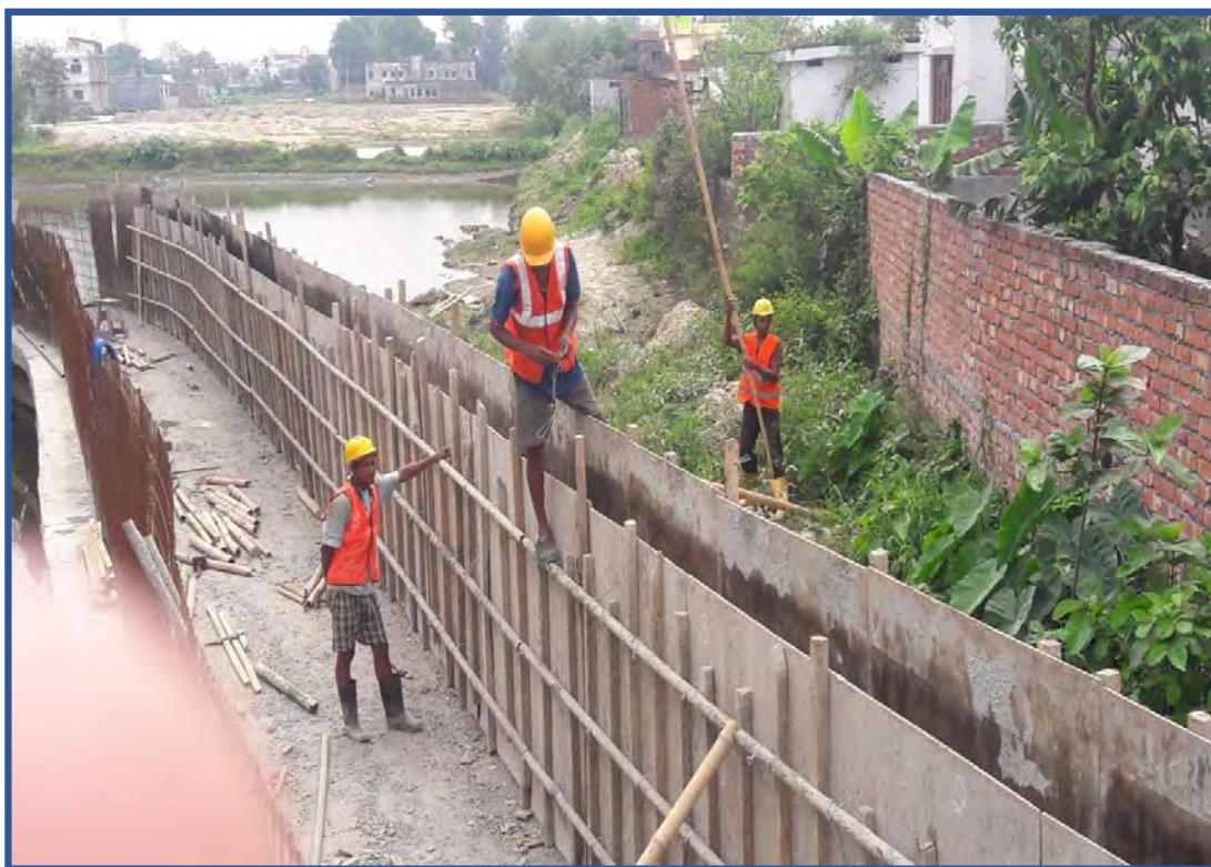
Formwork at Storm water drain (Chyangbari Nala)
