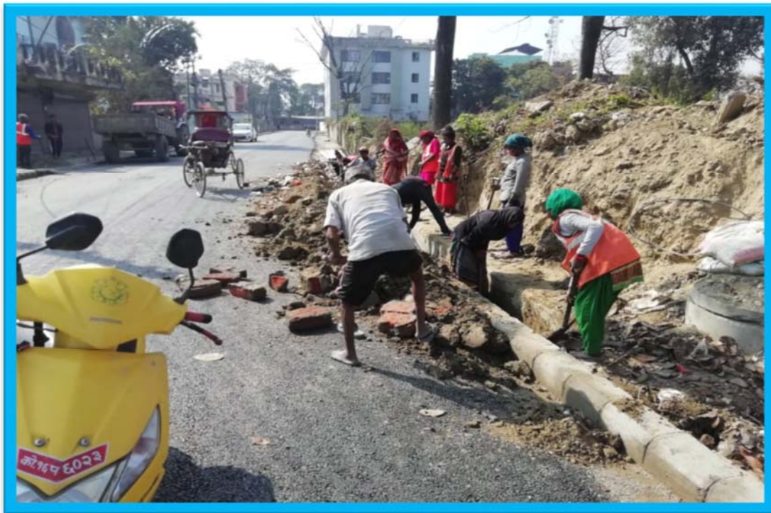
Drain Maintenance works
