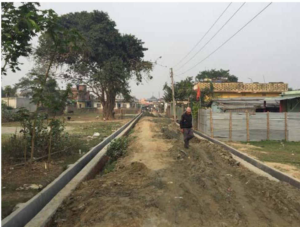
Figure 4. Lane improvement in Balgopal Tole, ward no 11, BSMC
