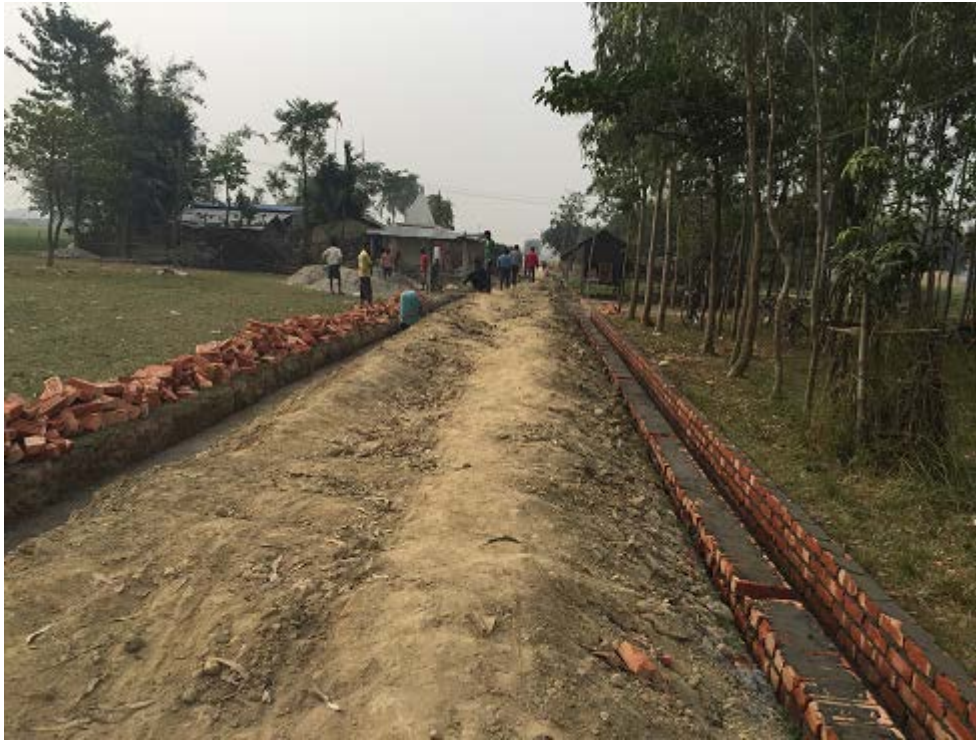
Figure 3. Lane improvement in progress, ward no 11, BSMC
