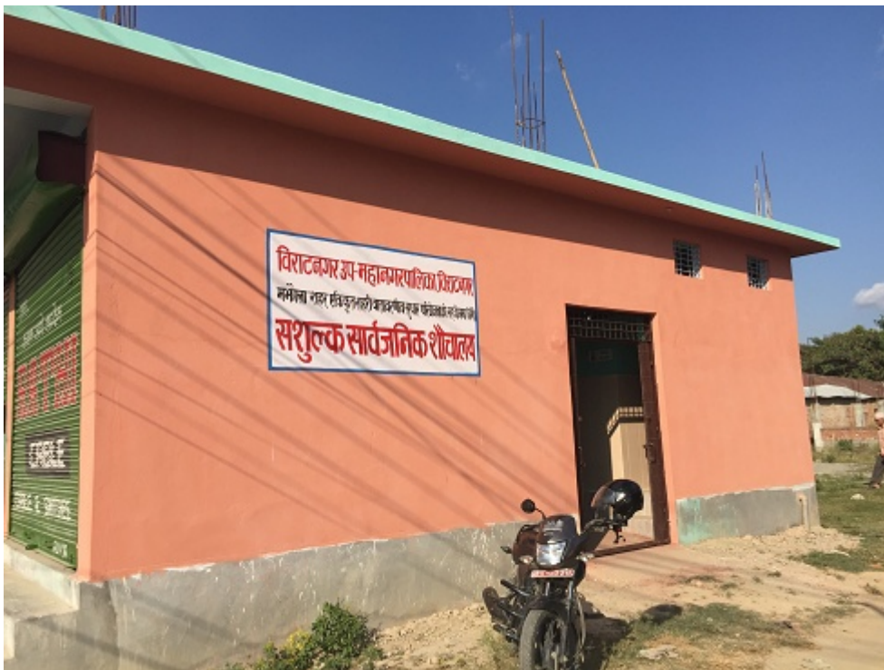
Figure 2. Completed Public Toilet
