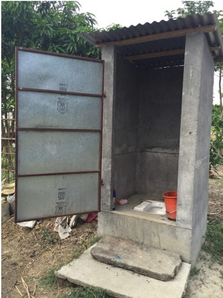
Figure 5. Completed Family Toilet
