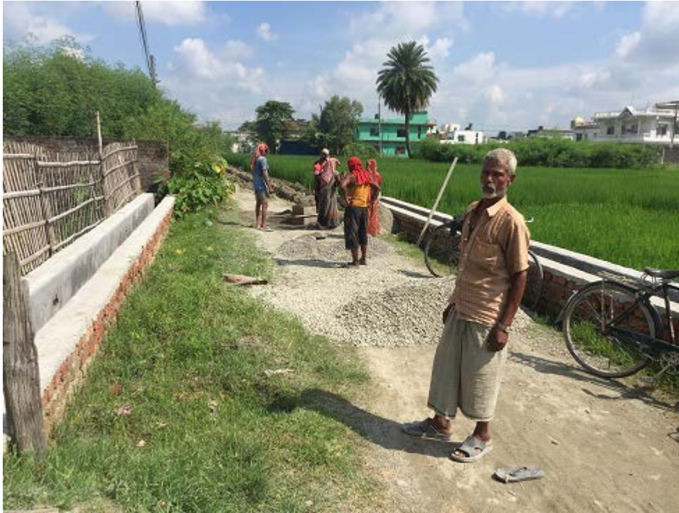
Figure 1. Lane Improvement works in Shruti Marga ward no 6
