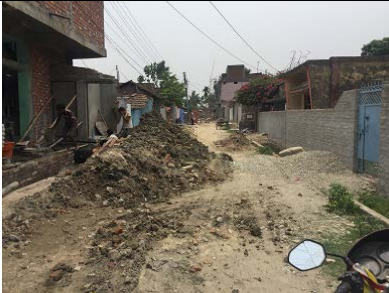
Figure 1. Lane Improvement works
