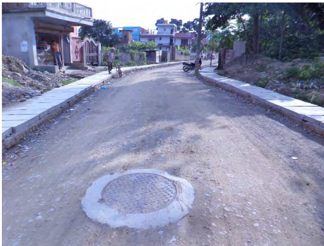
Sub-base work at R42
