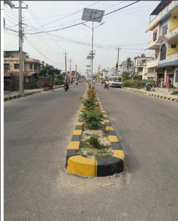
R2 Road is Ready for Taking Over
