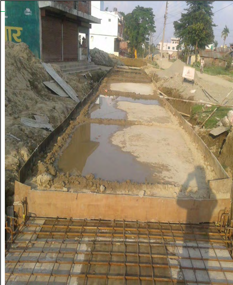
RCC Storm Drain at Line A1L2
