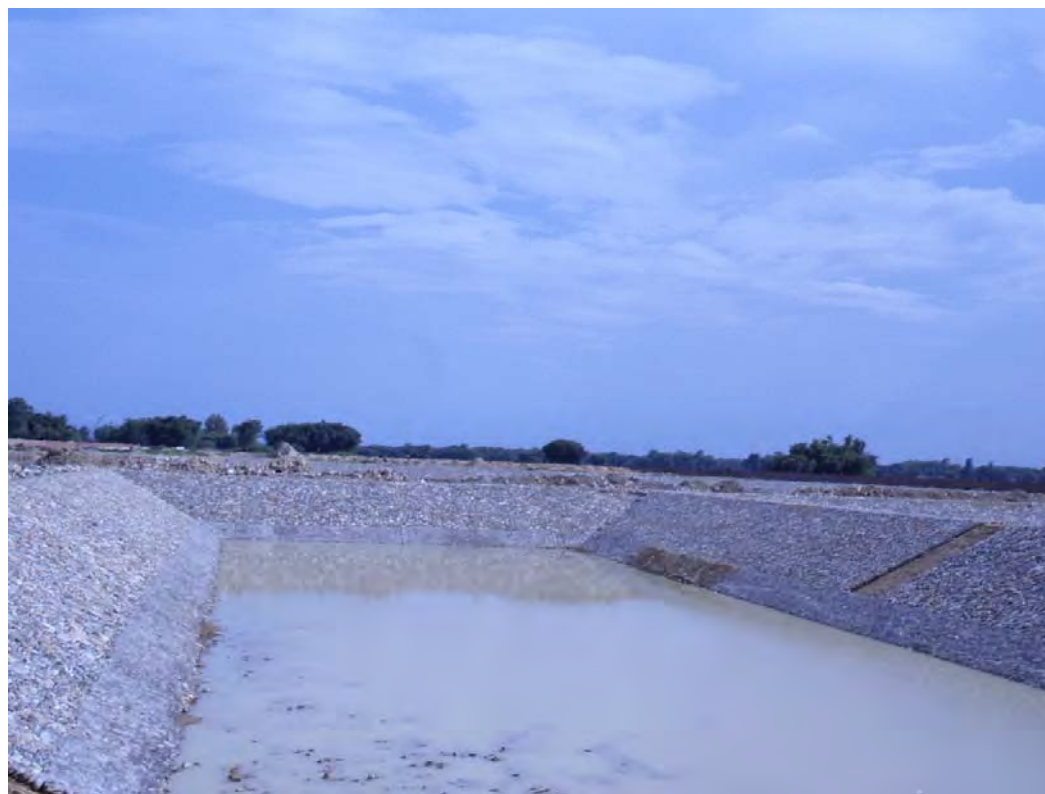
Rip-rap work in ponds at WWTP
