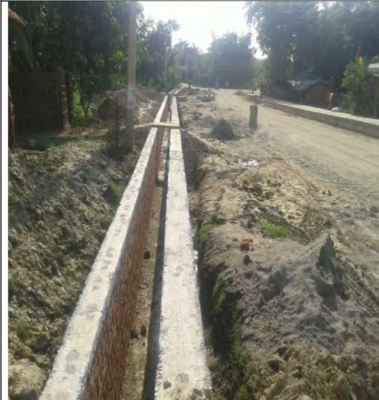
Construction of Road side Drain
