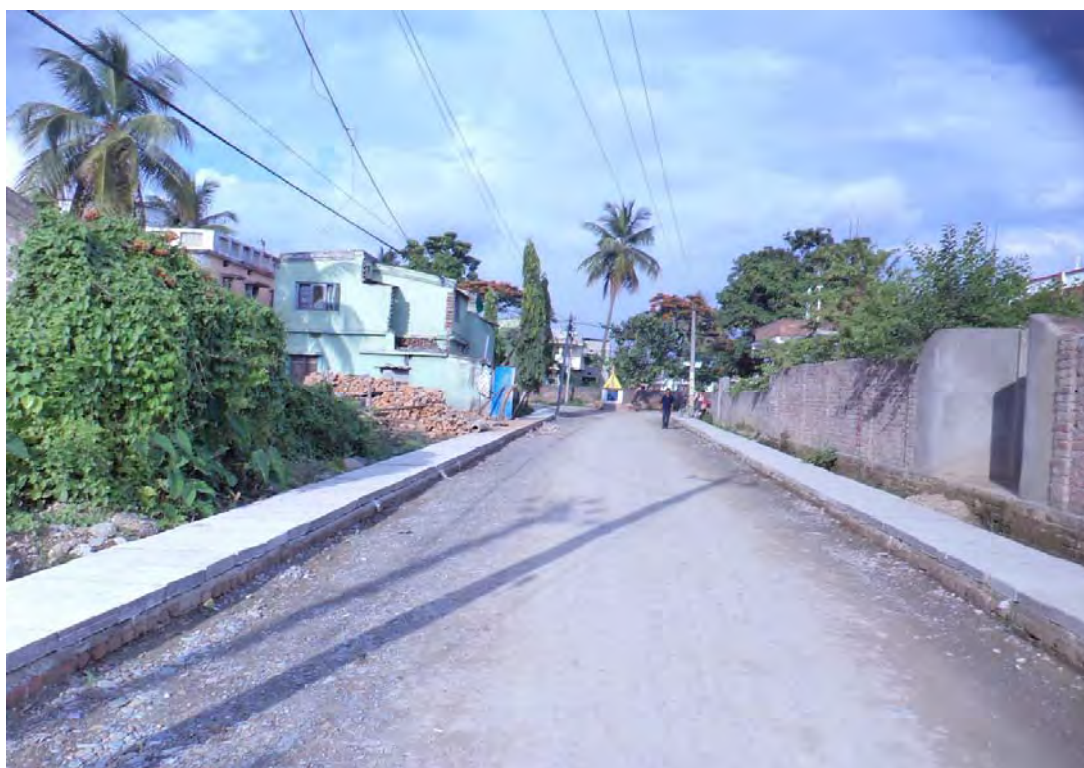
Road side drain construction at R8
