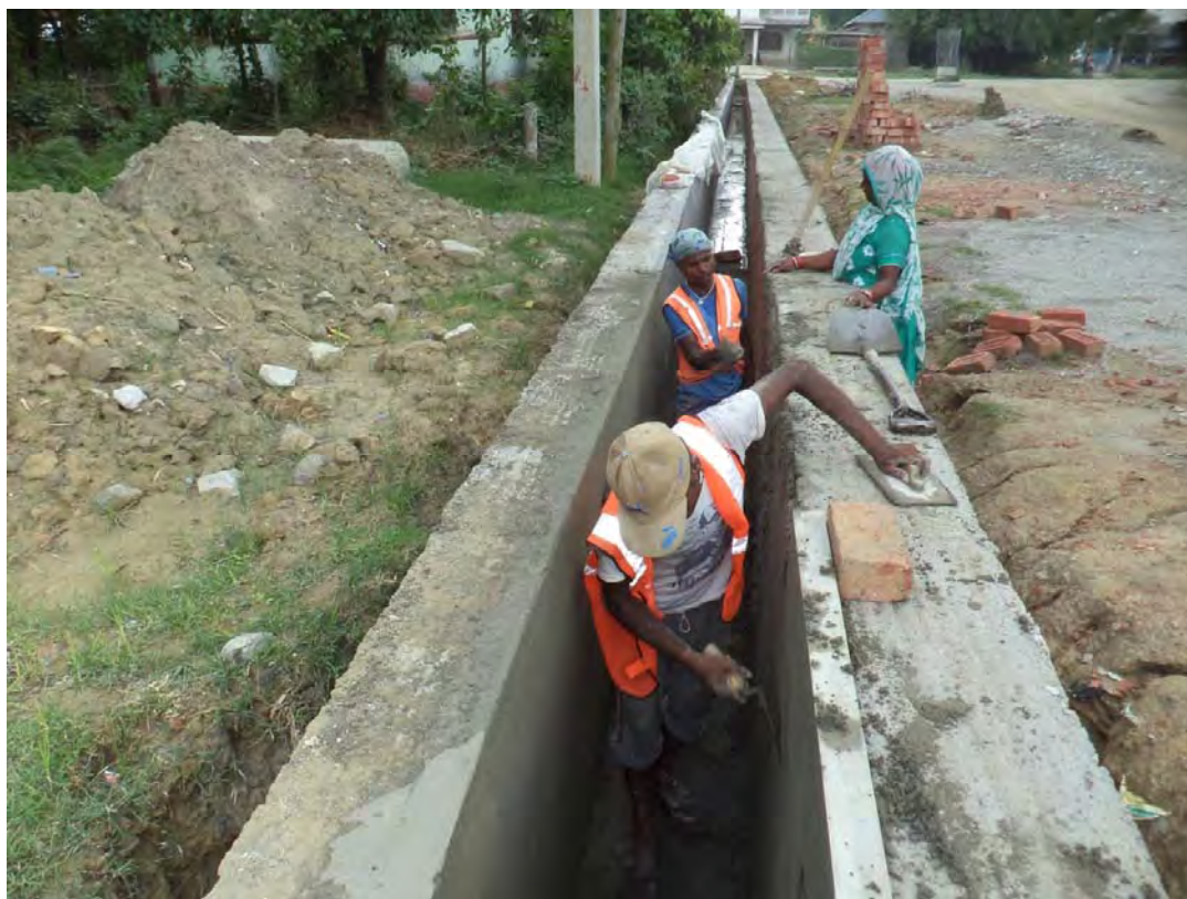
Road side drain at R4
