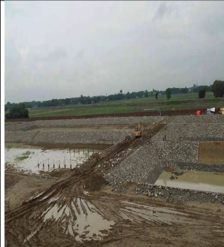
RIP-RAP Work at WWTP
