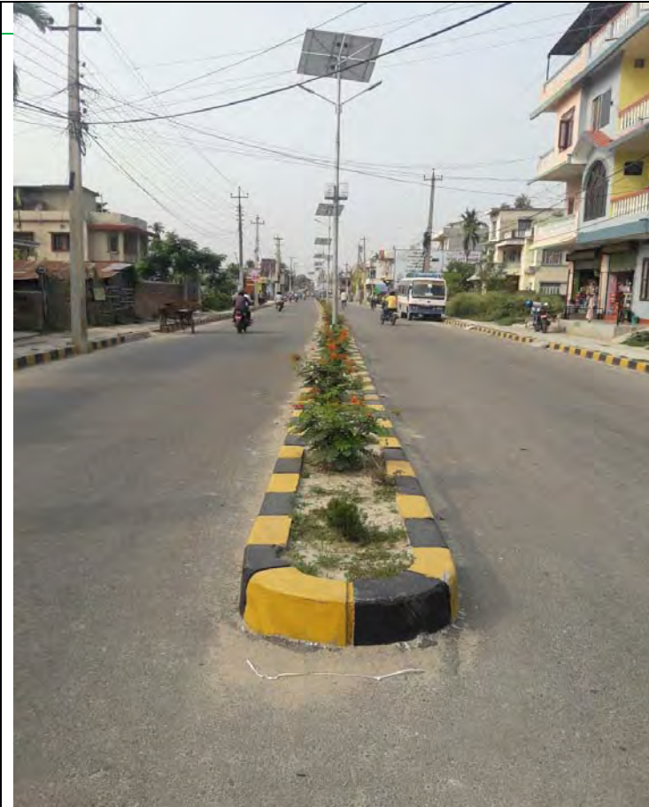
R2 Road is Ready for Taking Over
