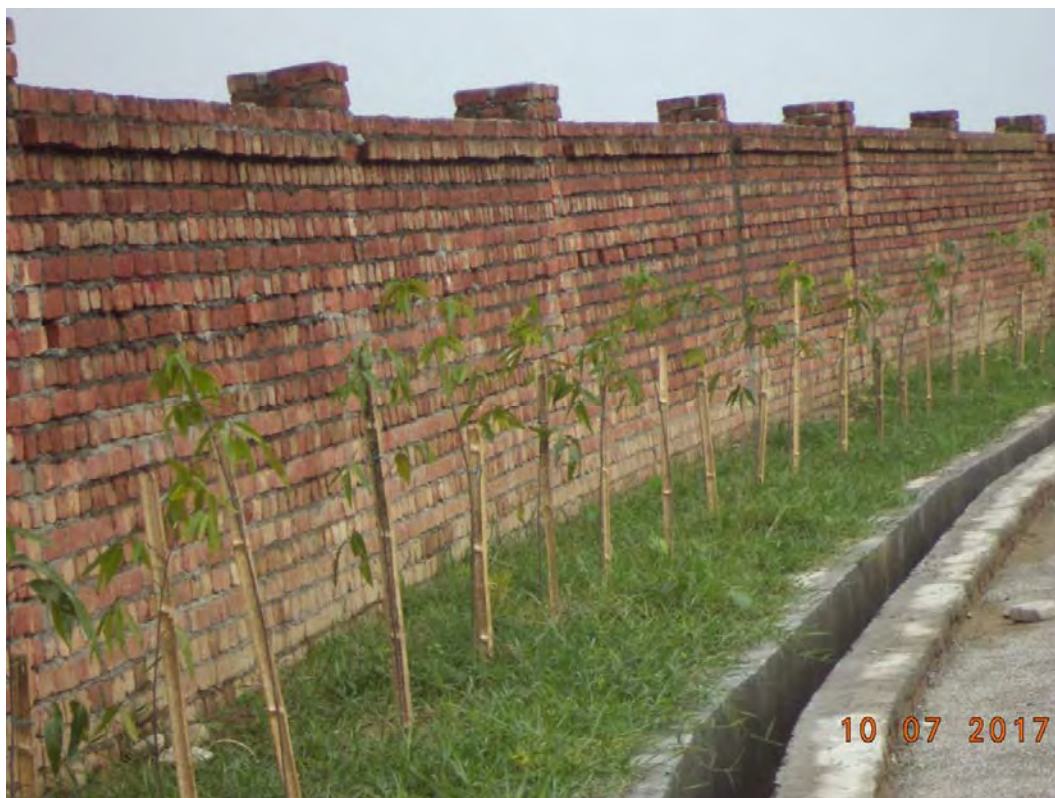
Bio- engineering at WWTP
