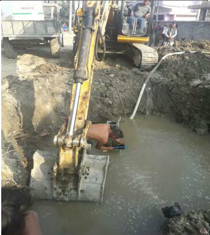
Maintenance of Drinking Water Pipe in T1 Trunc
