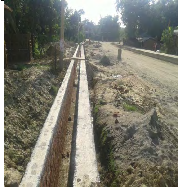
Construction of Road side Drain
