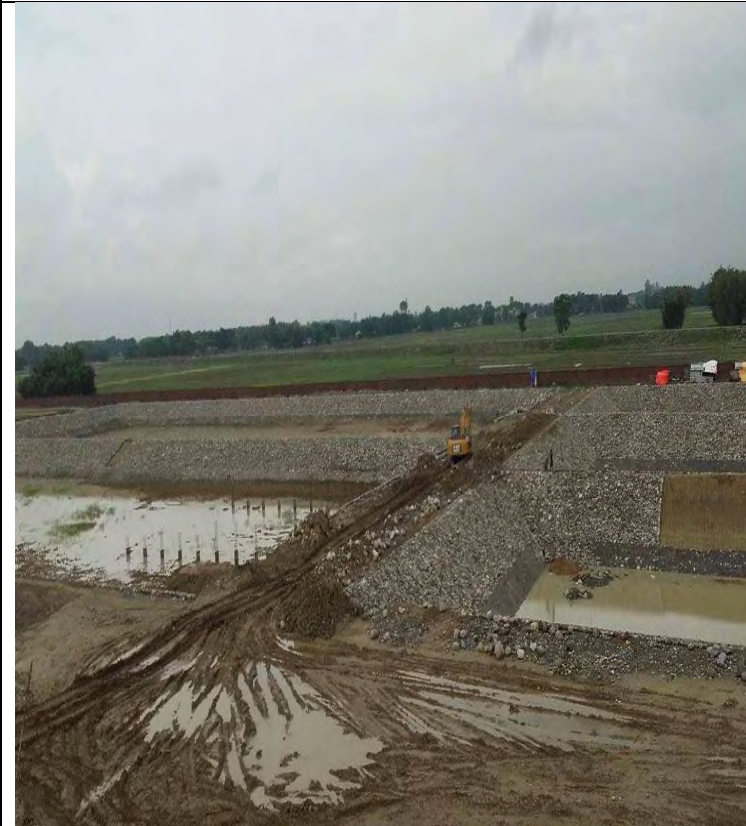
RIP-RAP Work at WWTP
