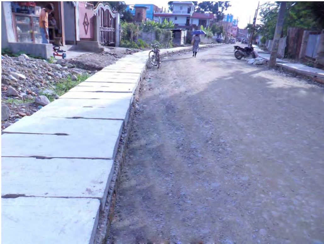
Sub-base at R42
