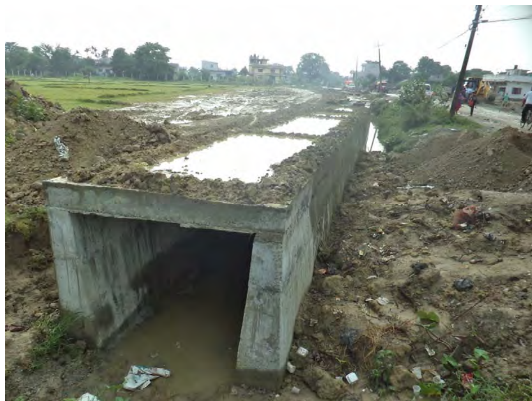
RCC drain at A1
