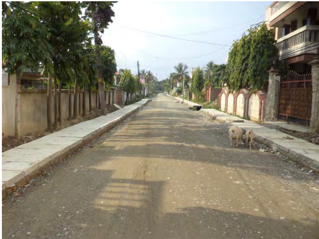
Sub-base at R104
