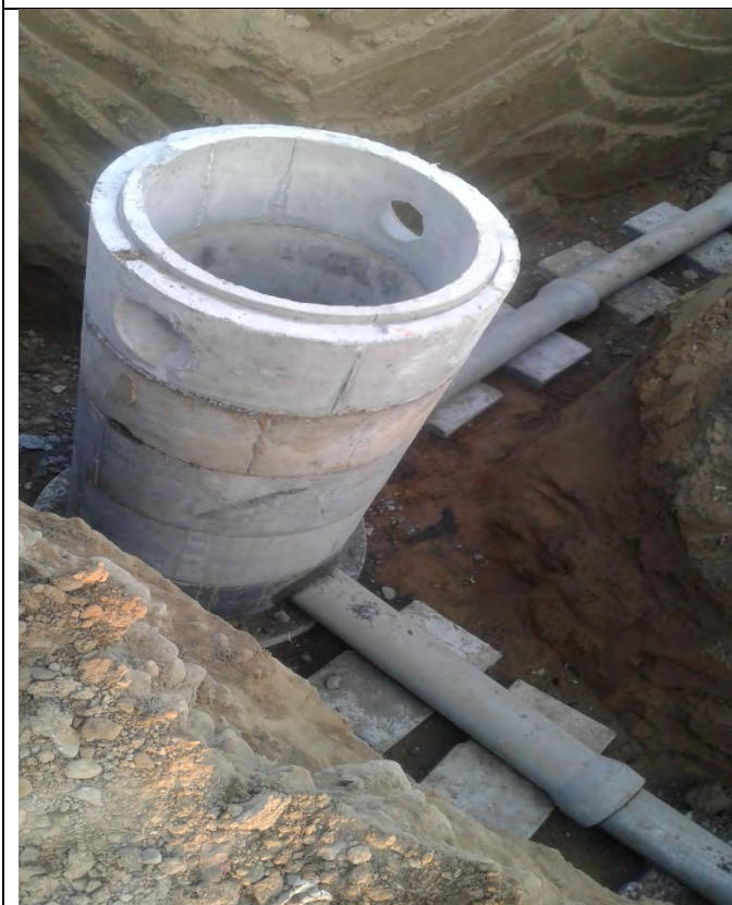
Installation of Manhole with connection of RCC Pipe
