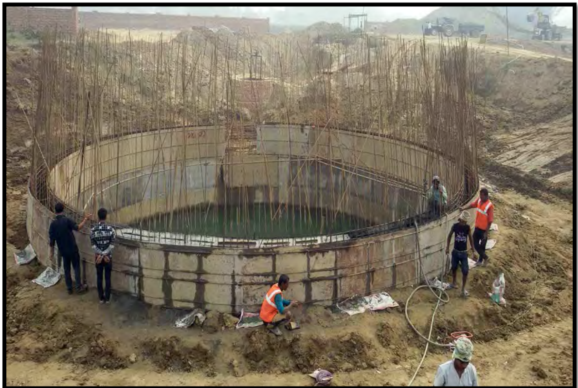
Concreting work sump well
