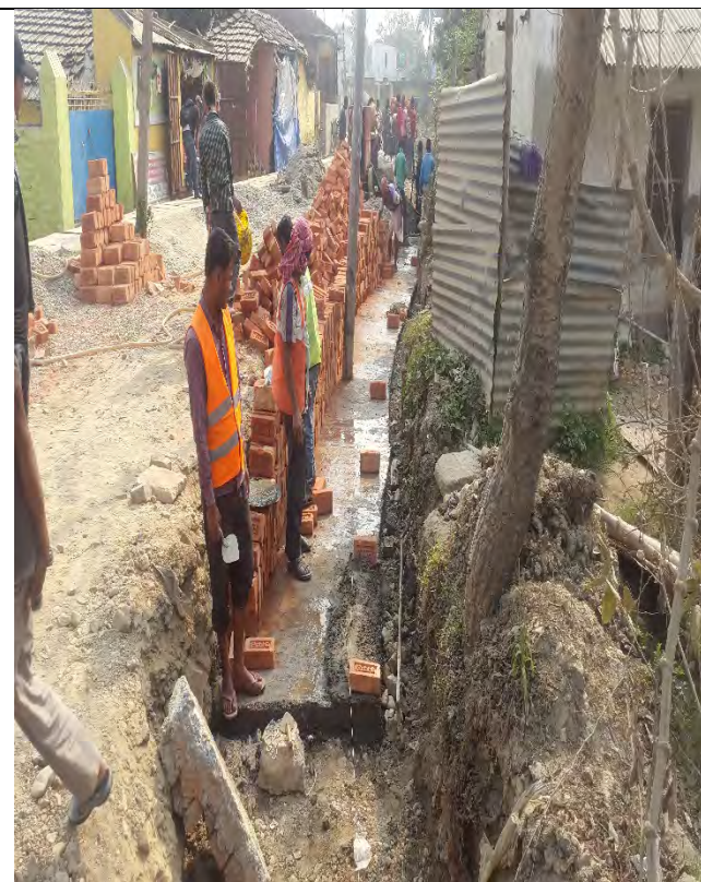
Road side drain is under construction
