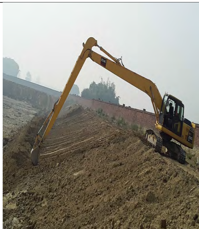
Slope Preparation of Anaerobic Pond
