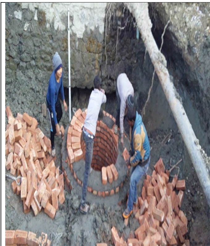
Brick masonry manhole at Koshi Highway (Trunk line)
