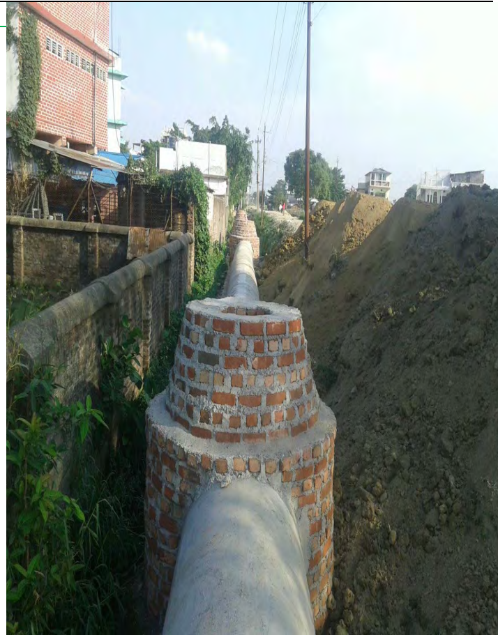
1000mm diahume pipe laying at CN3L1A
