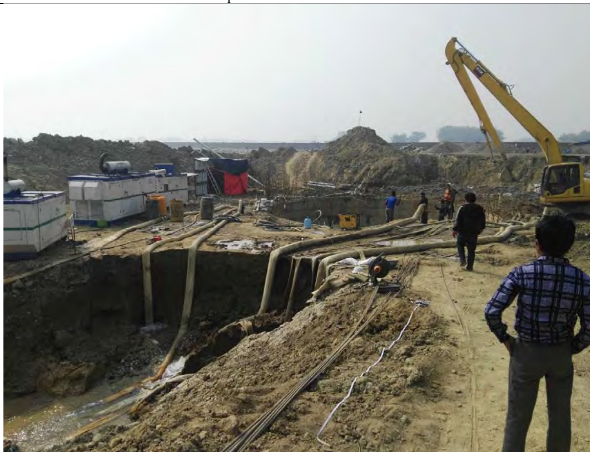
Dewatering in Sump well
