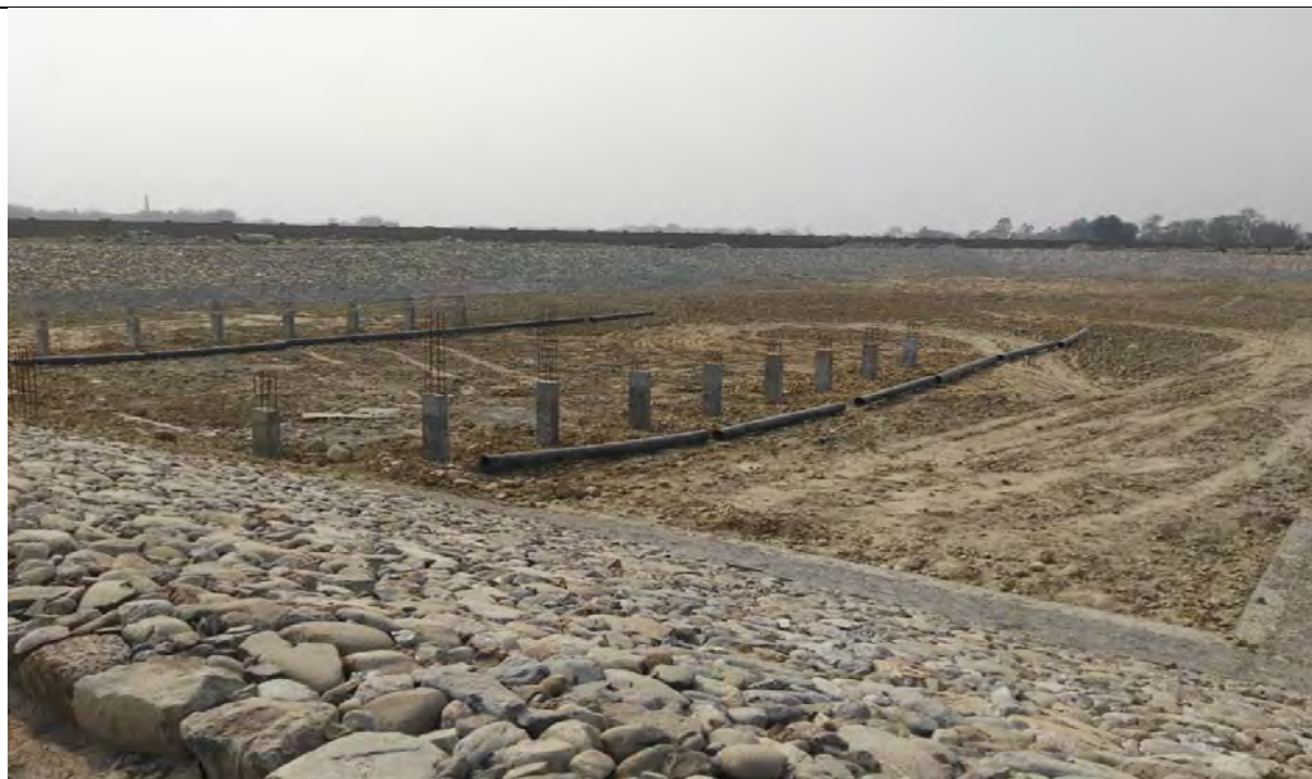
Pipe laying in the ponds
