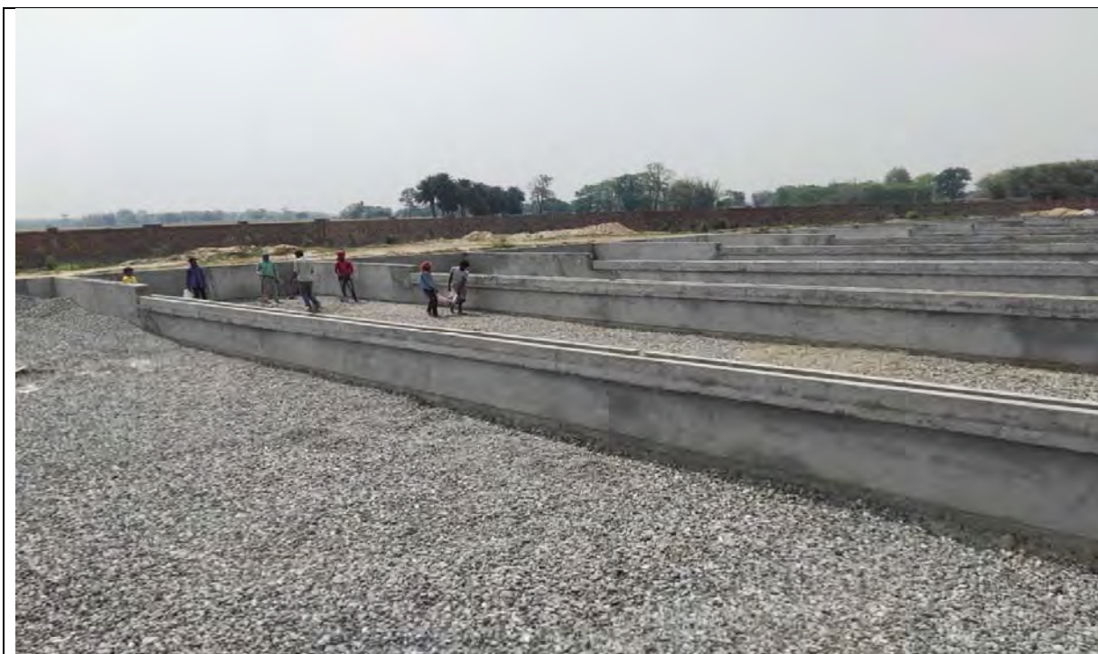
Sludge drying bed – filter materials laying
