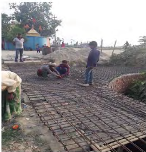
Bar bending in B2
