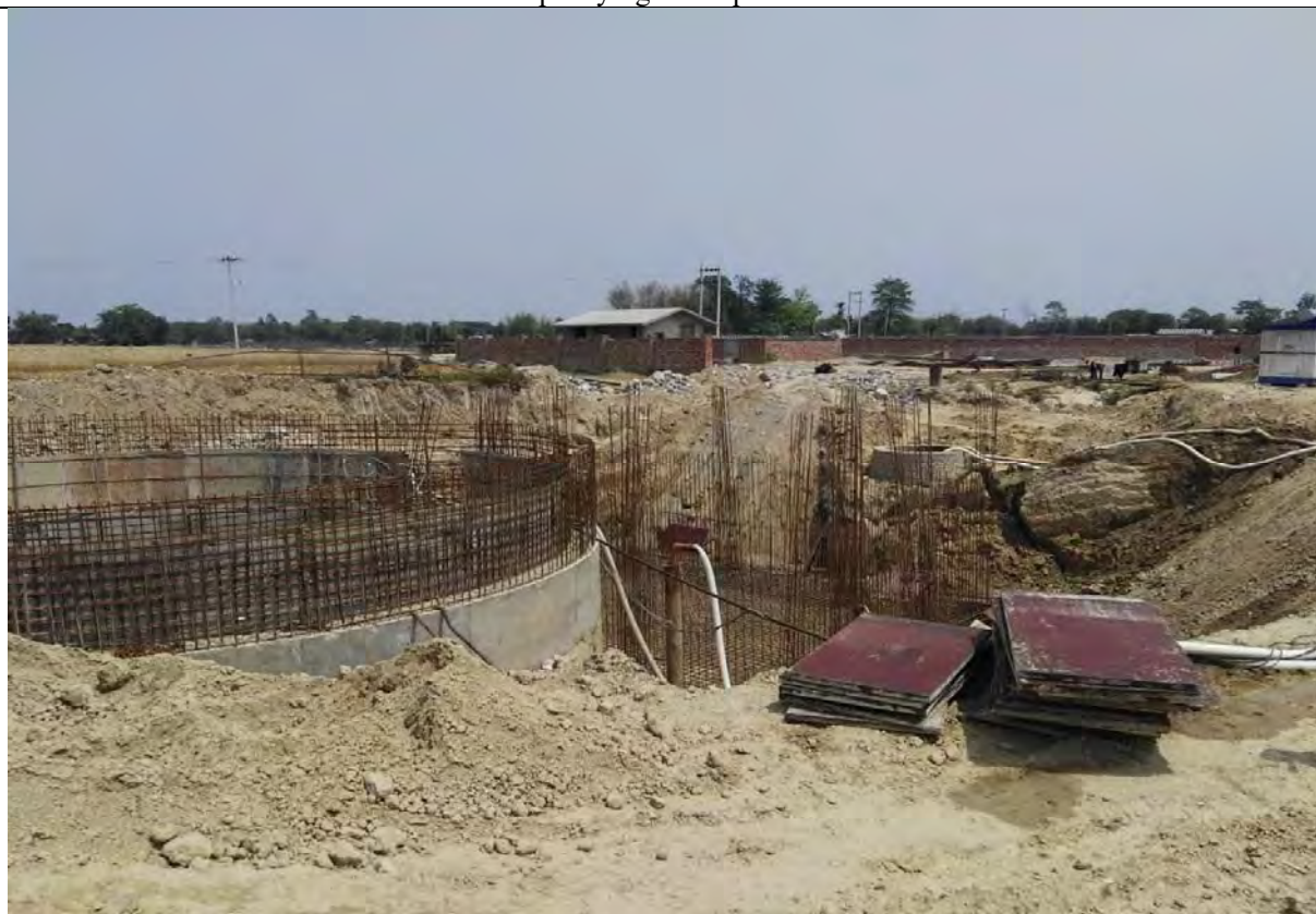
Sump well shear wall re bar
