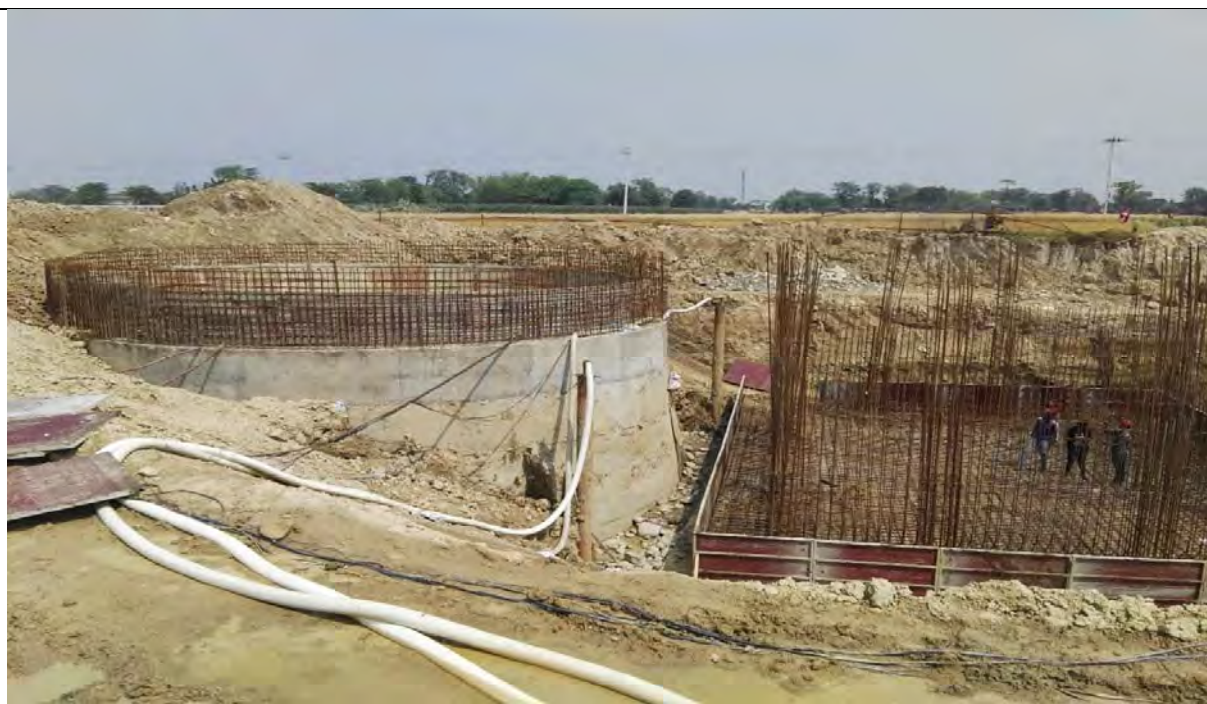
Sump well and enclosure chamber
