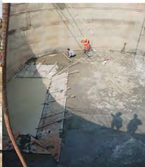
After Raft Concreting at Sump well
