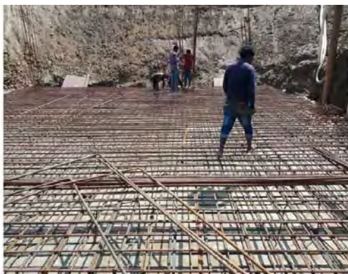
Raft in Enclosure Chamber
