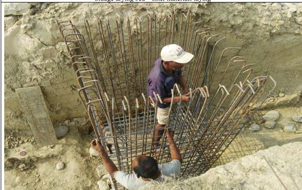
Interconnection chamber - WWTP
