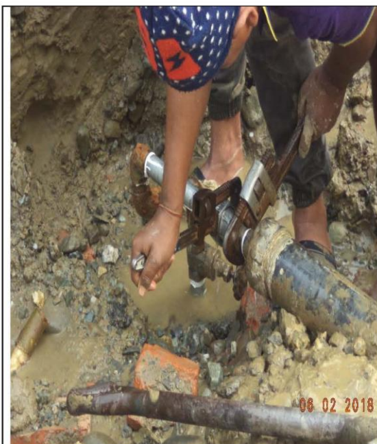
Pipe Joining for water supply
