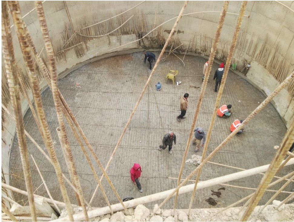
A view of Sump Well at WWTP after bottom plug sealing
