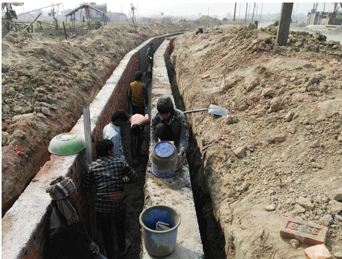
A view of B2 brick storm drain work
