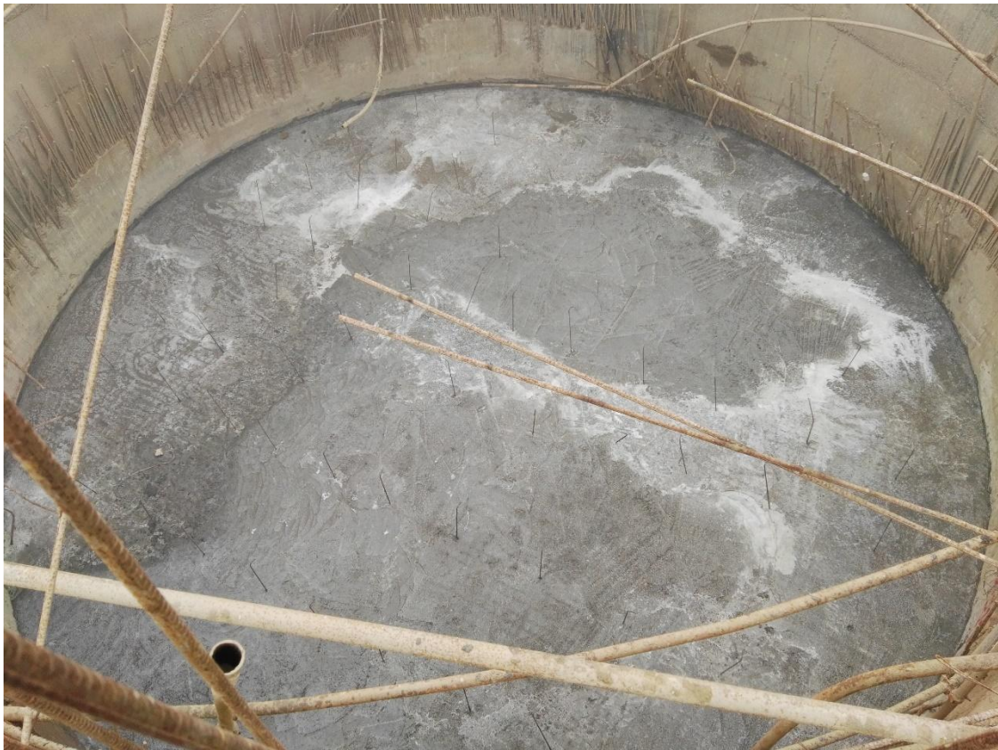
A view of WWTP after bottom plug concreting
