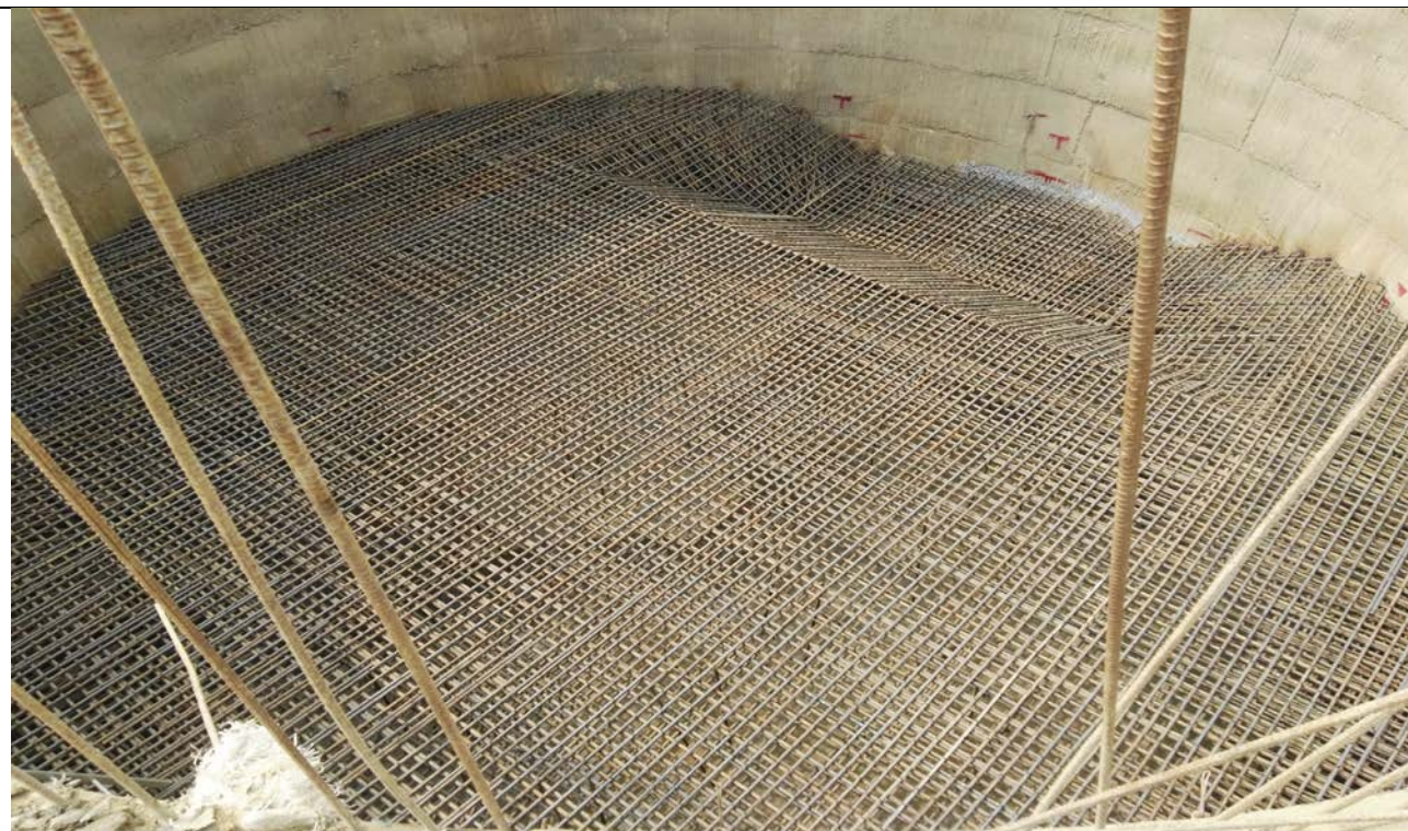
Re bar laying of raft of Sump well – WWTP, Jatuwa
