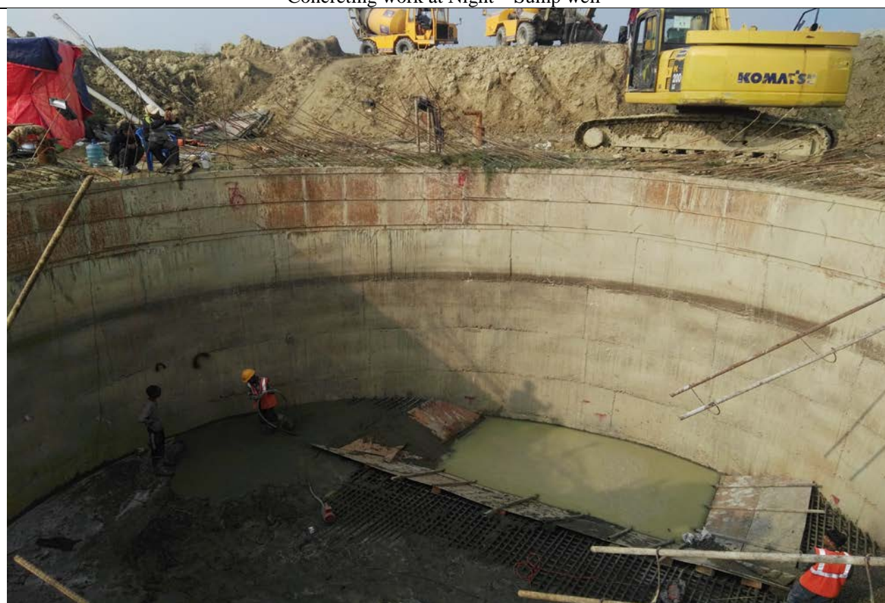
Concreting of raft at final stage – Sump well
