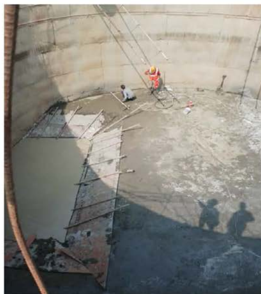
After Raft Concreting at Sump well
