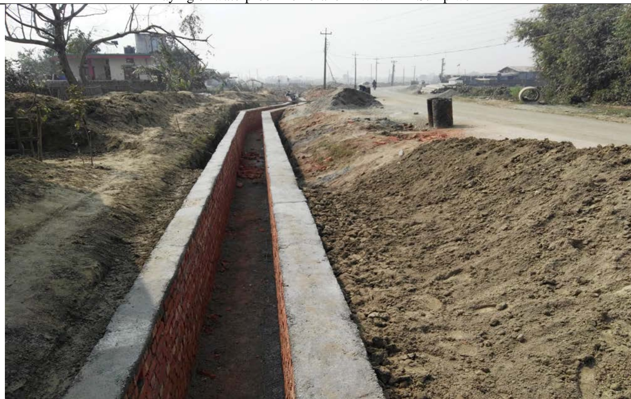
B2 – Storm water drain
