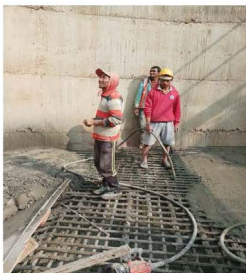
During Raft Concreting Sump Well
