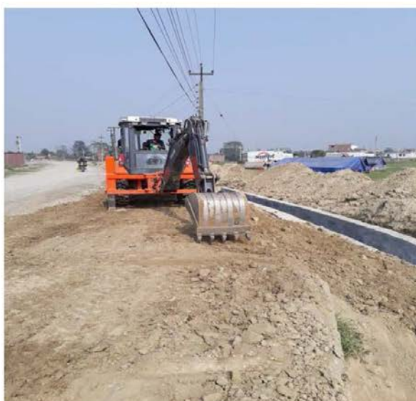
B2 – Backfilling
