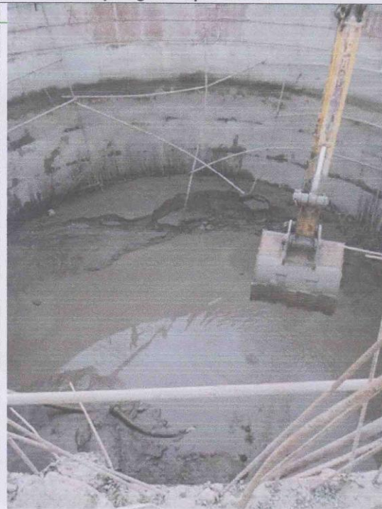
Dewatering and cleaning work at Sump well
