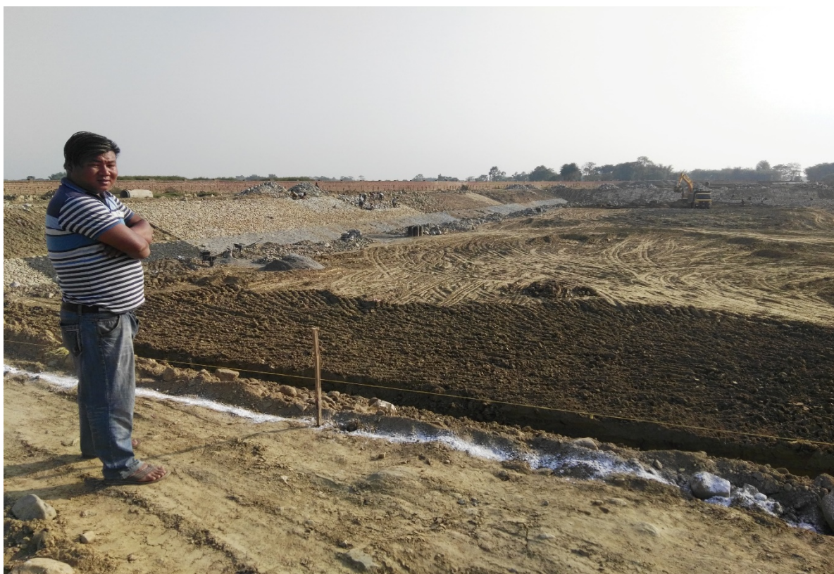
Facultative Pond: ongoing Rip Rap works
