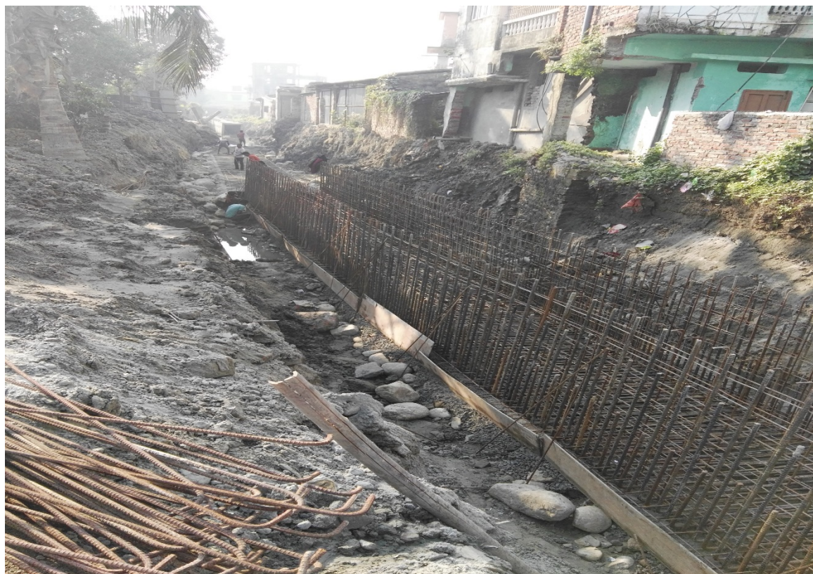
Storm water drain S9: Re bar for raft & shear wall
