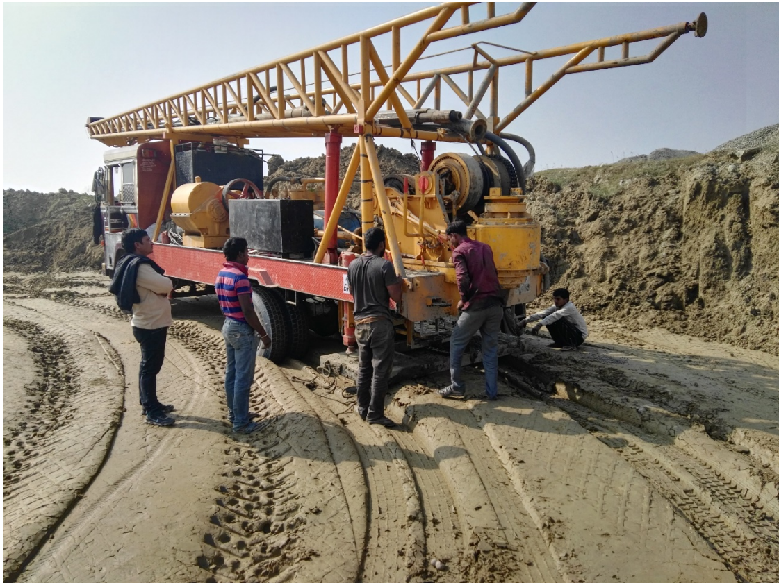
A view of Sump Well at WWTP (creation of bore holes)
