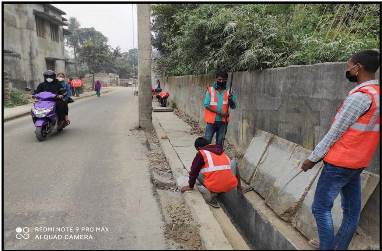
Line Level correction work at R6
