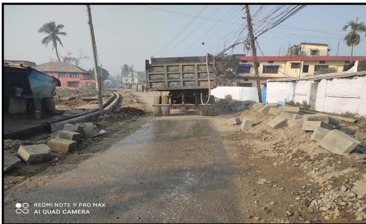
Water sprinkling for dust minimization
