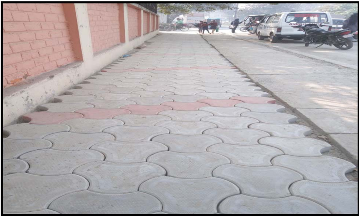
Interlocking work at R7 (near Sahid Stadium)
