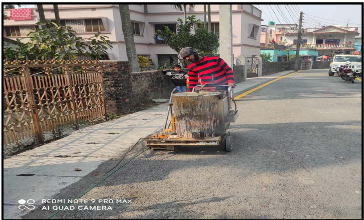
Thermoplastic work at T3Line22A
