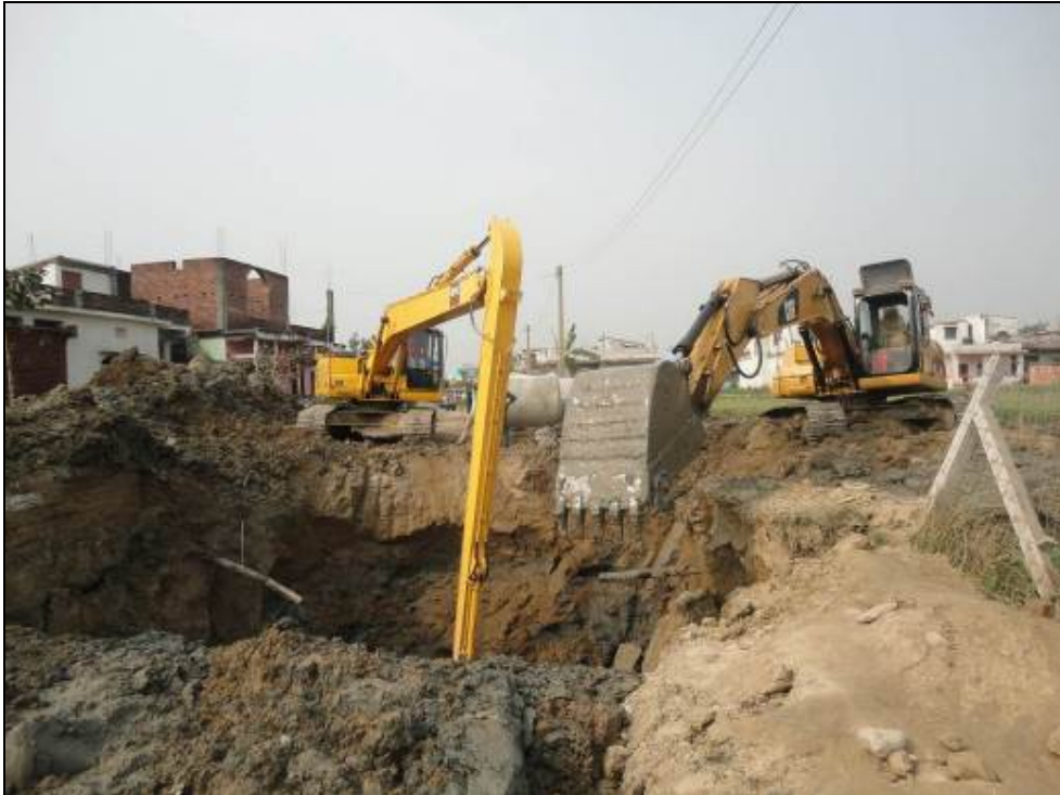
Excavation of Trench for 1,600mm Dia. RCC pipe at S13 Storm Drainage
