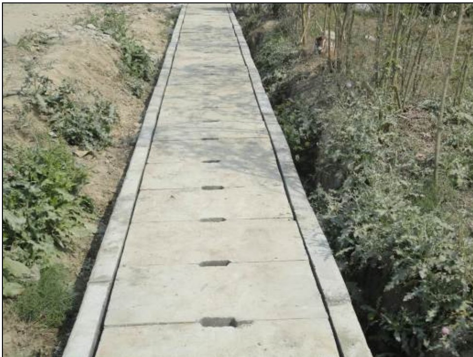
Drain Cover with Pre-cast slab guards at R2 Road(Pushpalal Road)
