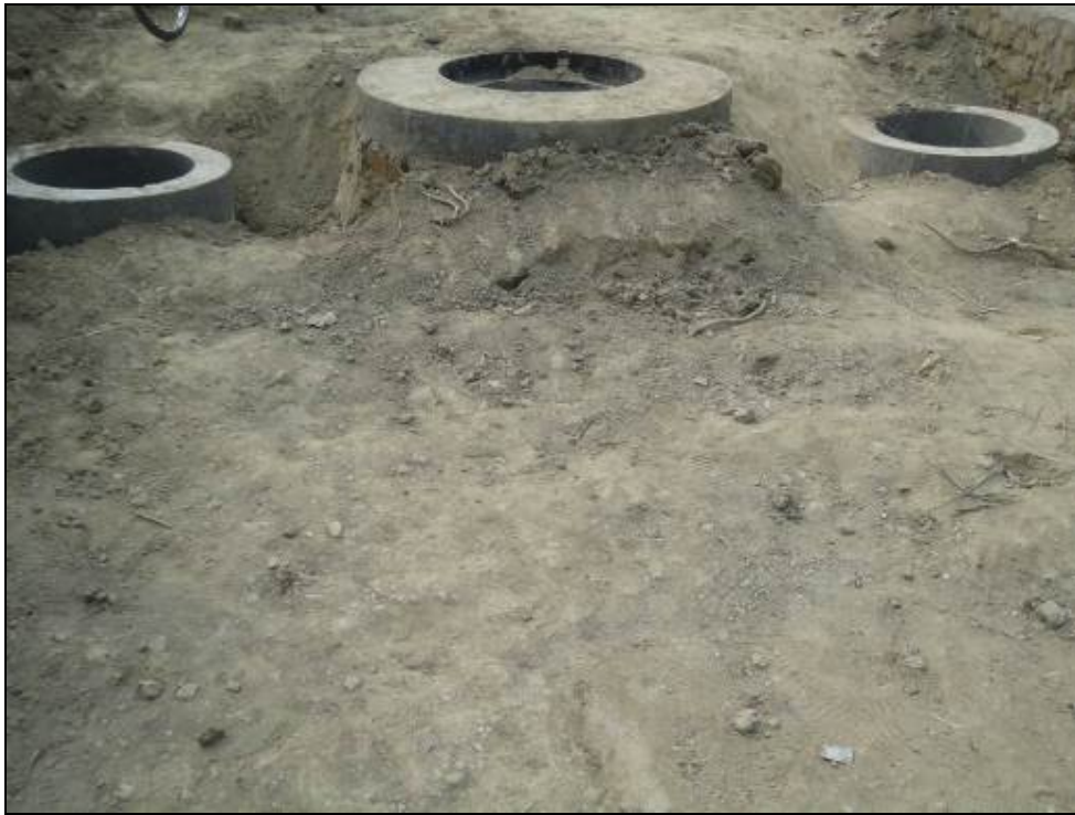
Brick Manhole at Center with Precast Sewer Inlet on Either Sides T3 Seondary Line
