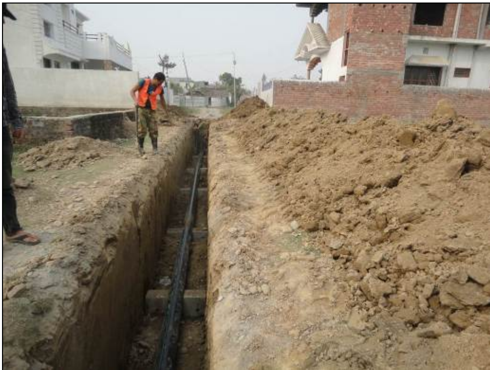
Laying of 200mm Dia. HDPE Pipes as Secondary Sewer Line
