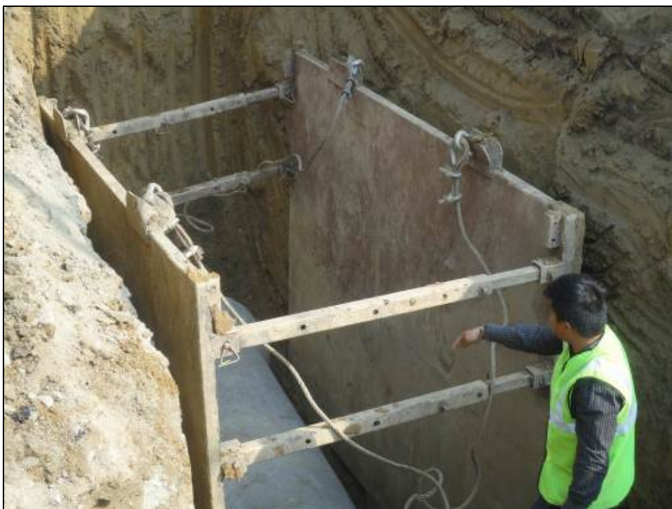
700mm dia RCC Pipe Laying with shoring at T3 (Trunk)Line ,Yadav Chowk- Devkota Chowk
