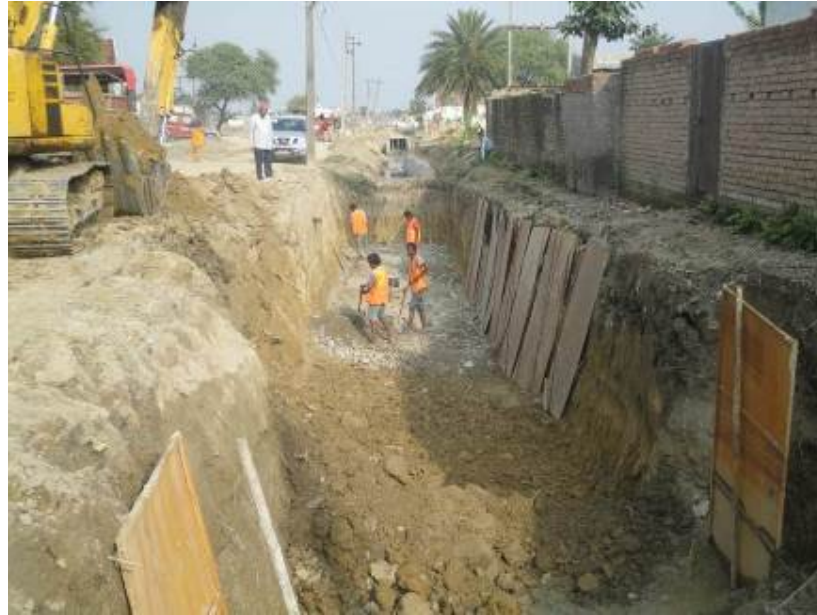
Gravel bedding in preparation near outlet of B2, DPS School
