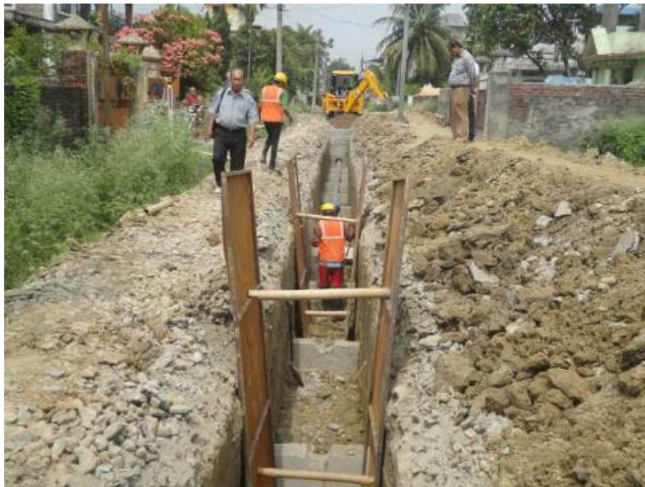
HDPE pipe of dia 200mm laying for sewer line
