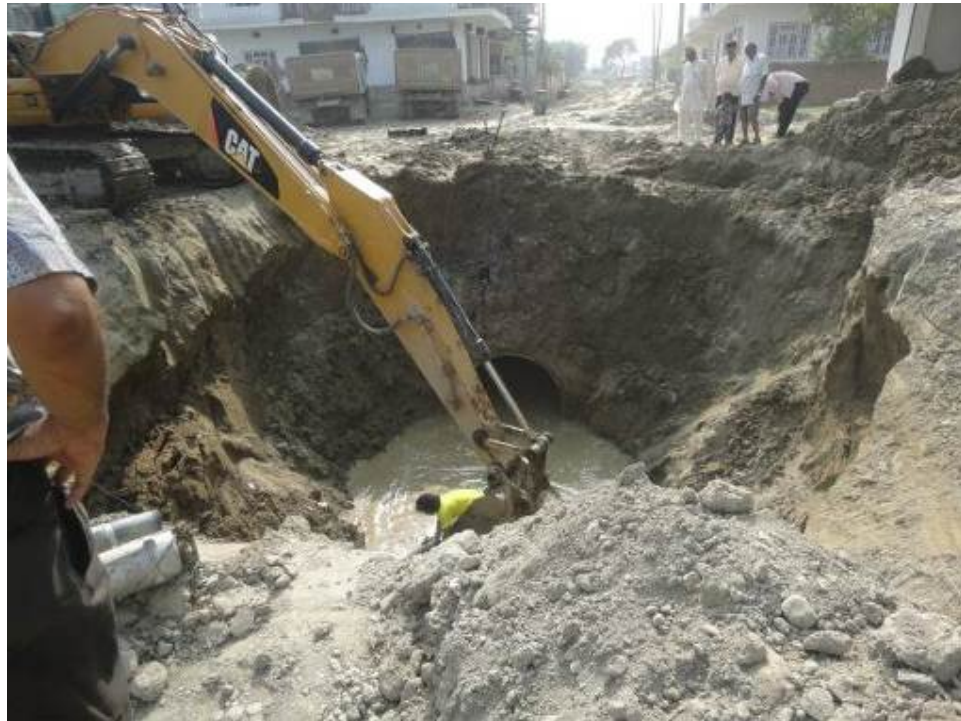
Dewatering and making ready for laying dia.1,600 mm RCC Pipe at S13 near R2 road crossing
