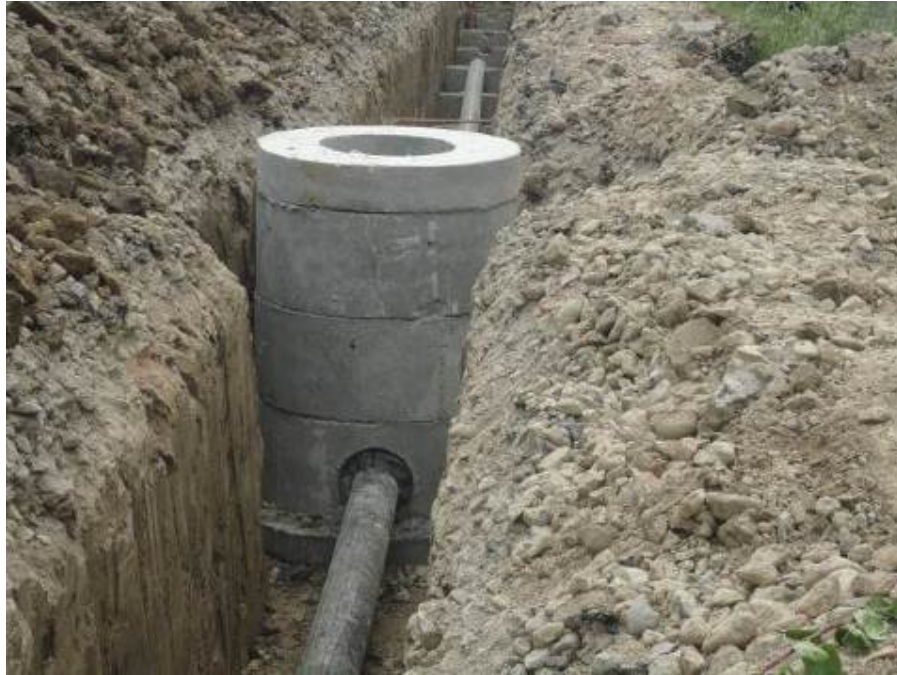
Pre-cast manhole installed at site
