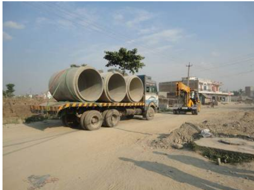
Unloading Dia.1,600mm RCC pipes near road crossing of Storm drain S13 at R2 Road
