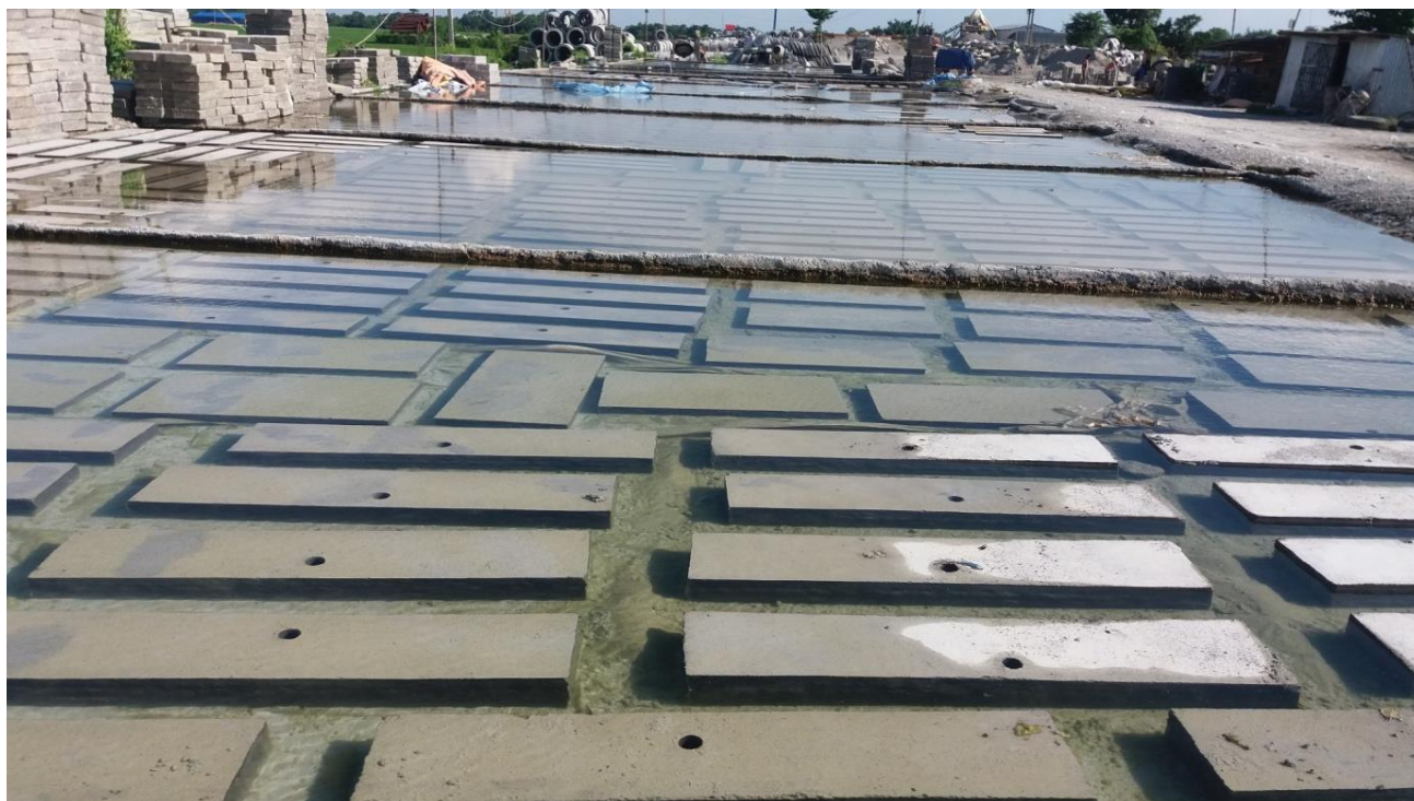
Picture 1 Curing of casted Cover slab at Contractor's yard
