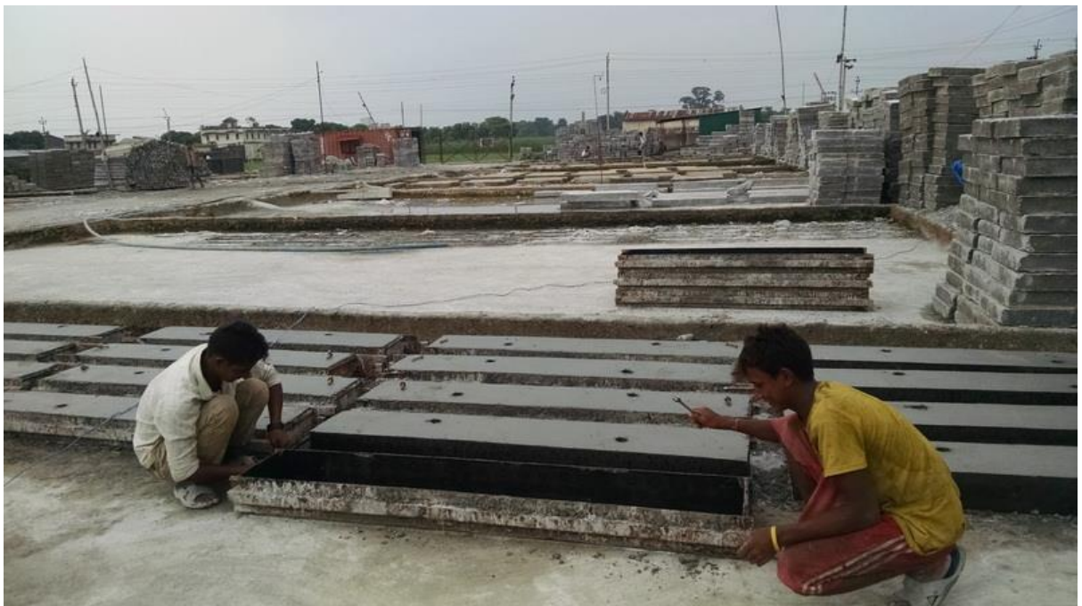
Figure 8 Precast Slab casting at Yard
