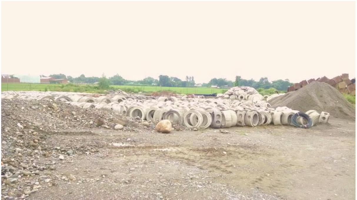
Figure 3 Precast Sewer Inlet Chambers casted and stocked at Yard
