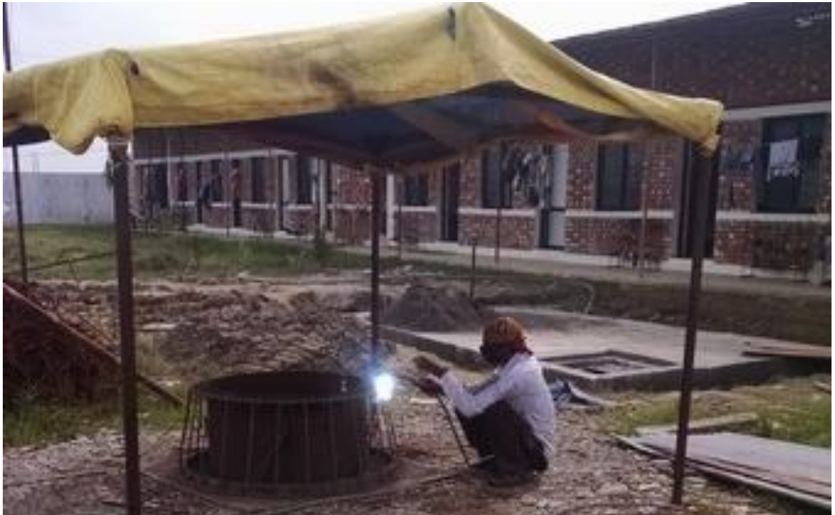
Figure 7 Welding of Precast Chamber Reinforcement
