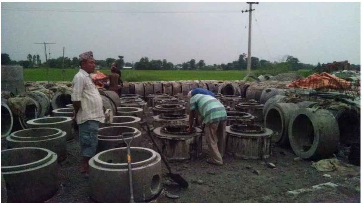
Figure 4 Precast Manhole Chamber Casting at Yard
