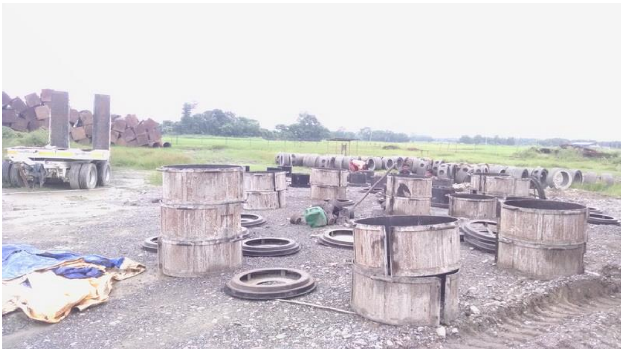
Figure 2 Formwork preparation before casting of precast chambers
