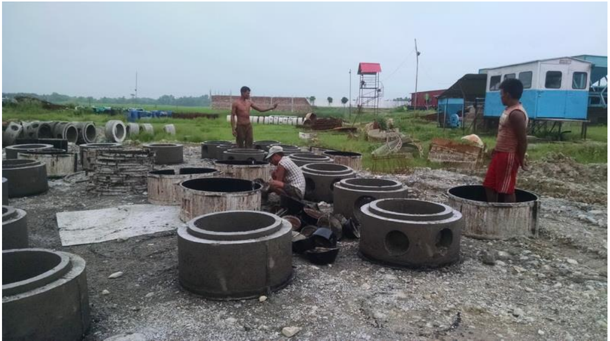
Figure 5 Precast Sewer Inlet Chamber casting at Yard
