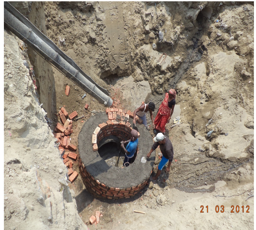
Manhole construction T1 trunk
