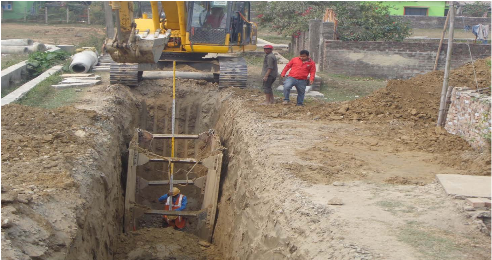
Pipe Laying work at T2 L19
