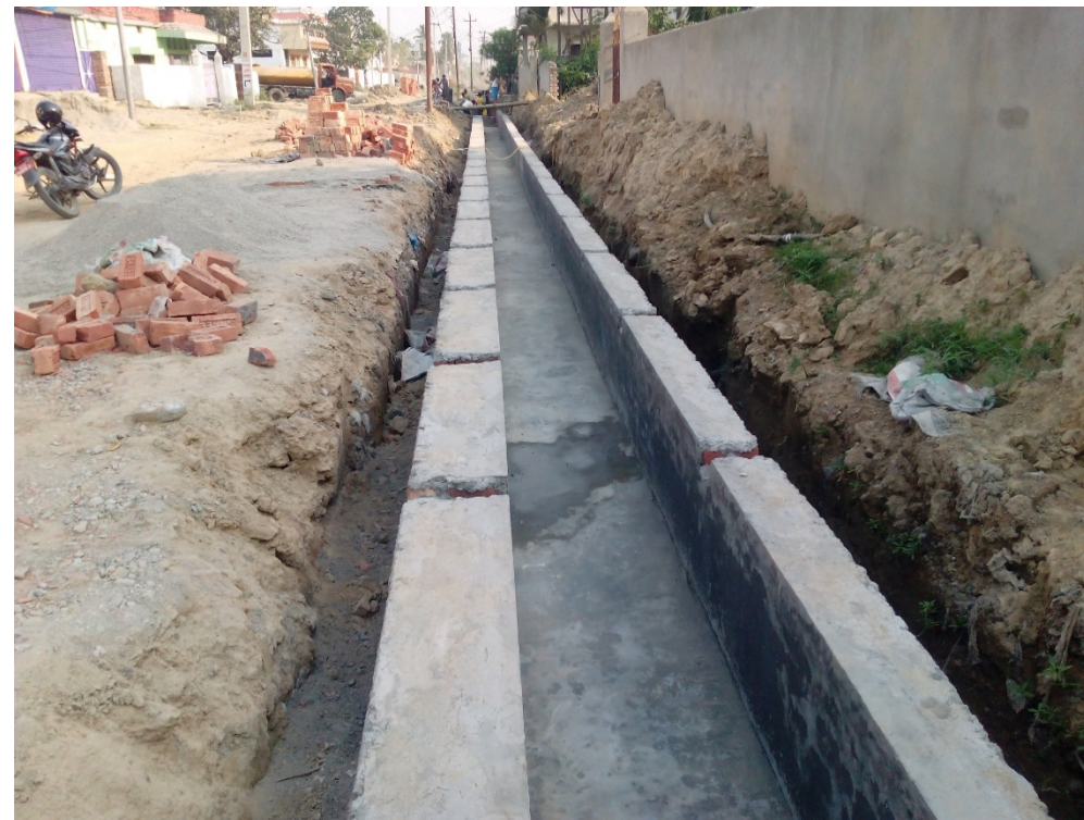
Road side Brick drain at R3 Dharambandh
