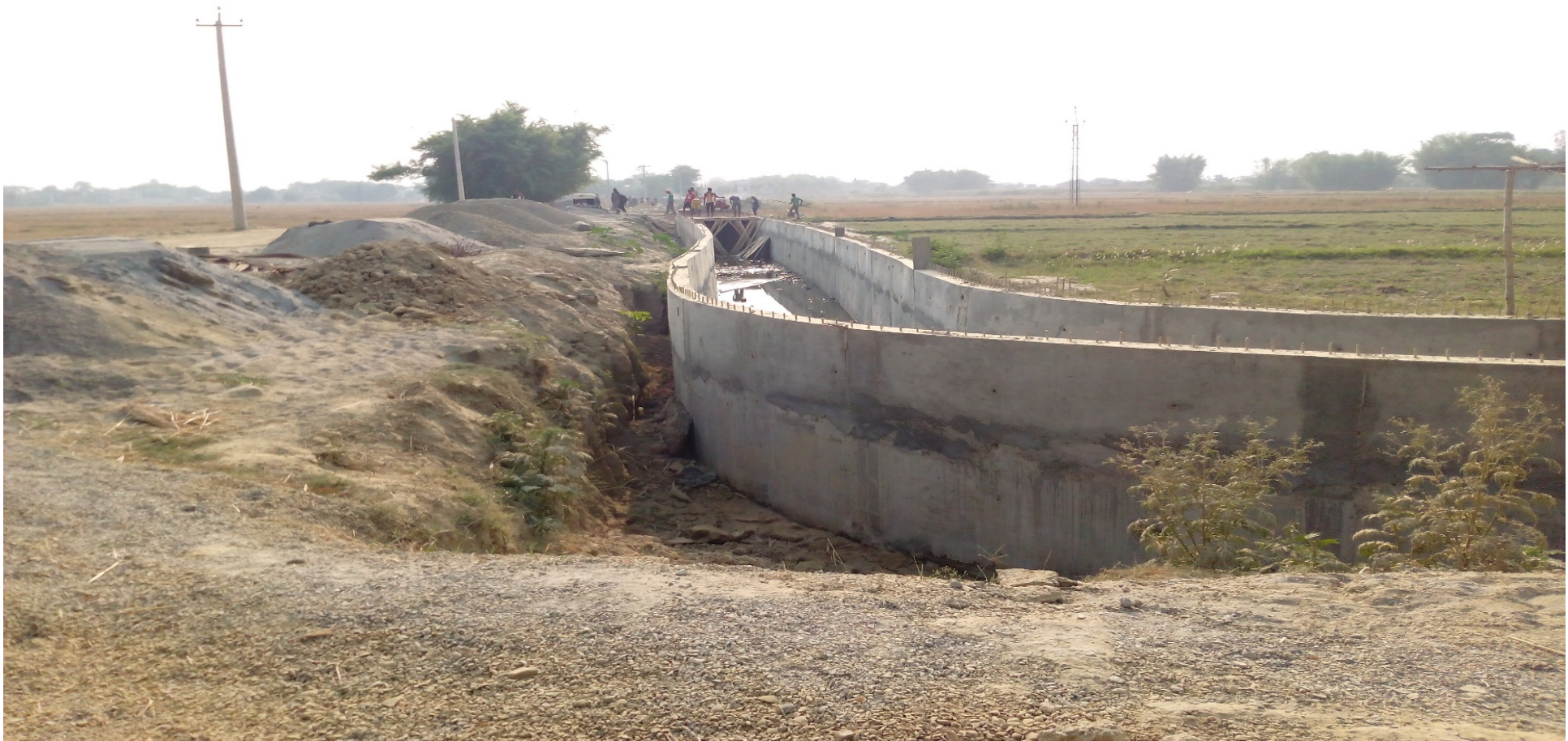
RCC Storm water drain at S5
