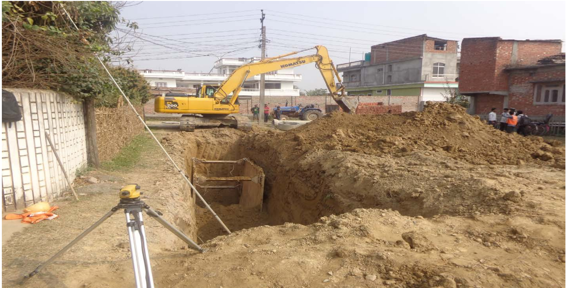
Pipe Laying work at T3 trunk
