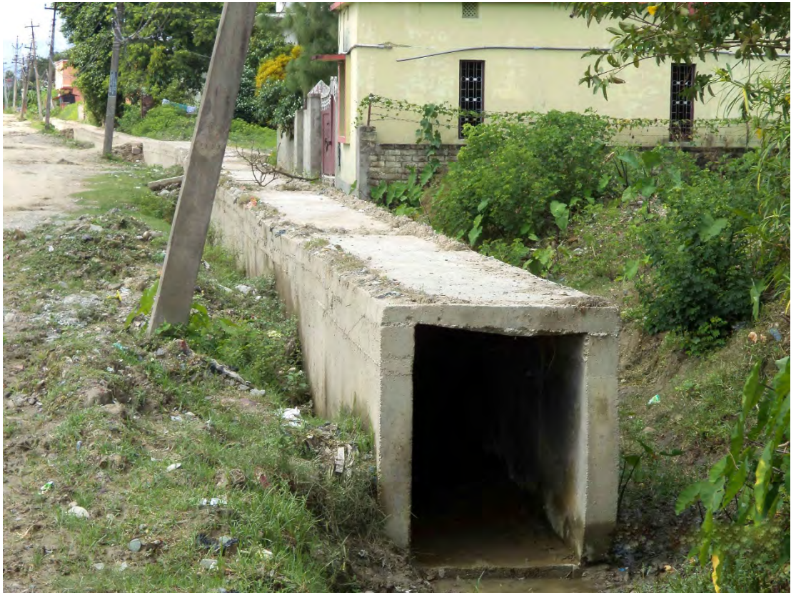
RCC Road Side Drain at R3
