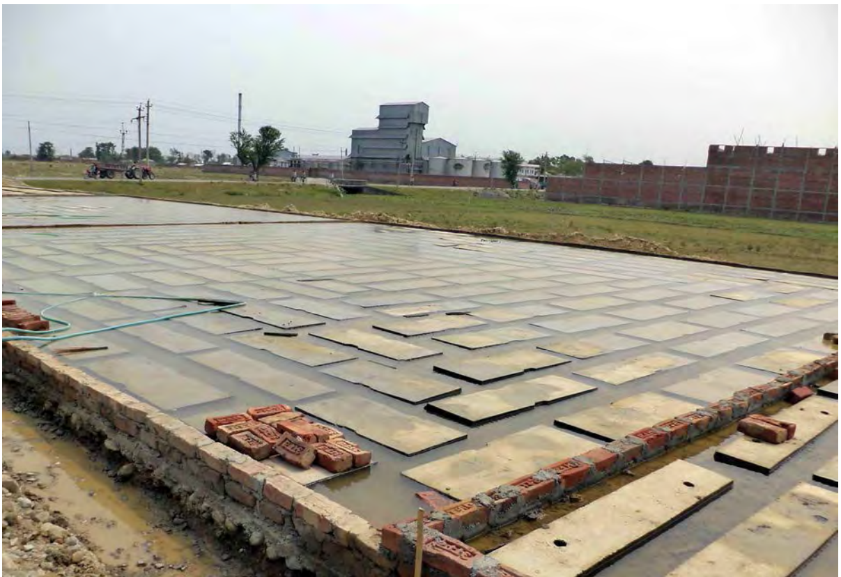
Precast Drain Cover Slab production at Contractor's yard
