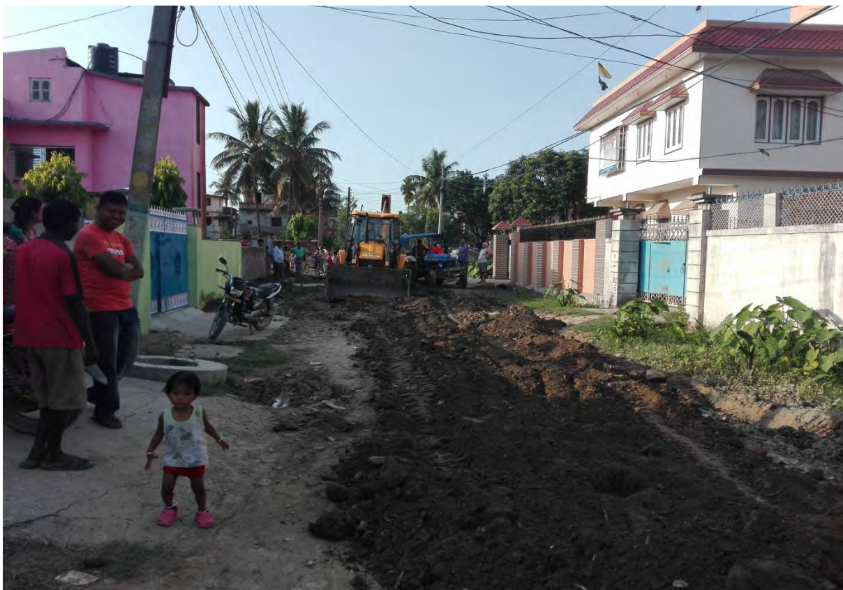
Picture 2 Road Maintenance work
