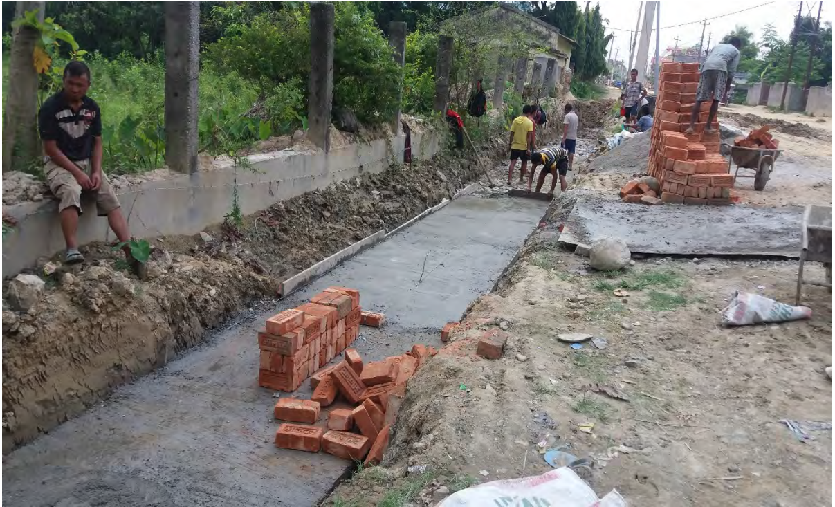
Road Side Drain at R3 (Dharambandh)
