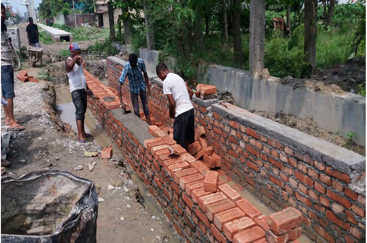
Road Side Drain at R3 (Dharambandh)
