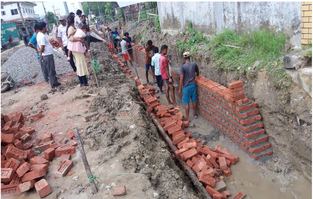
Road Side Drain at R3 (Dharambandh)
