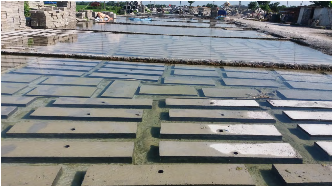
Picture 1 Curing of casted Cover slab at Contractor's yard
