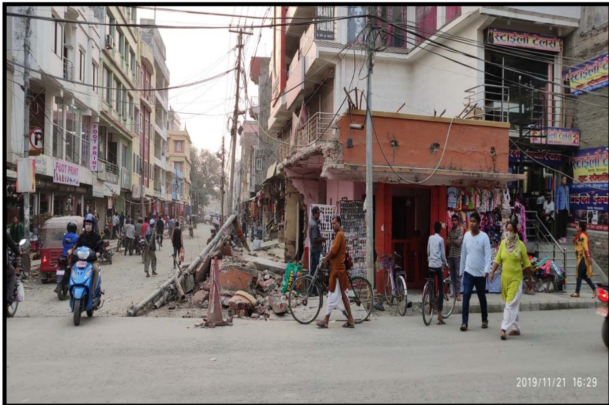
House owner's self-clearing voluntarily road width and footpath as per ROW approved by the BMC
