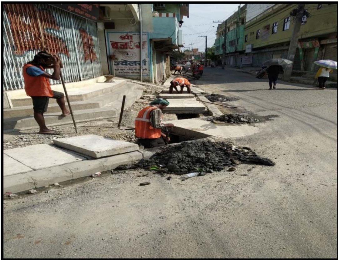
Drain cleansing at Sri Hospital road – at Junction of T3Line9 & T3Line10
