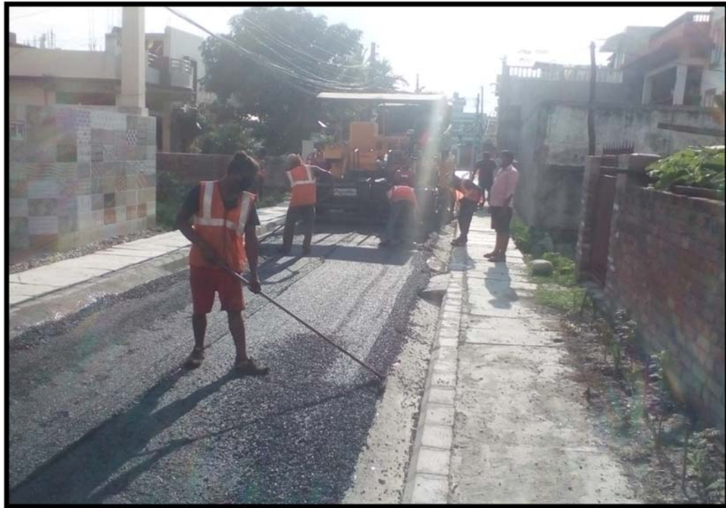
Asphalt laying at T2L18A
