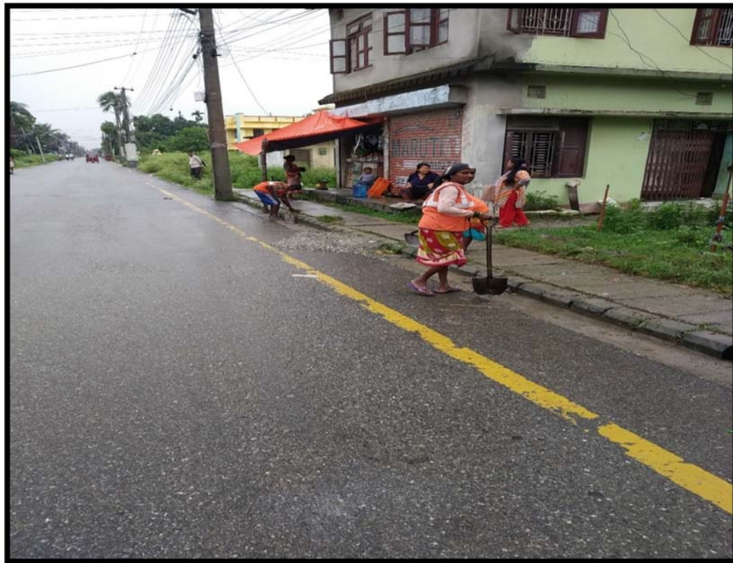
Gutter / Teak drain cleansing work at R114
