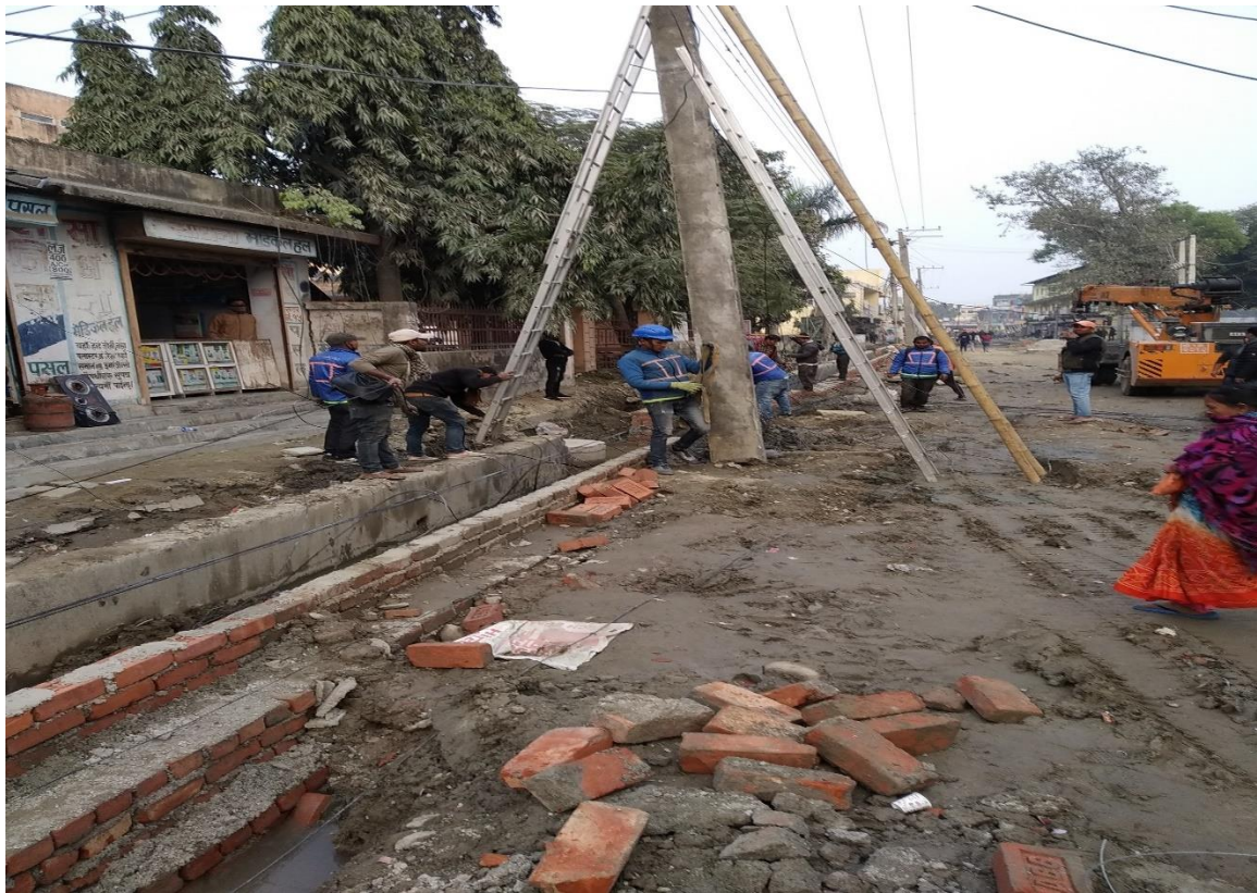
Relocation of electric poles at Hospital chowk in Rangeli road
