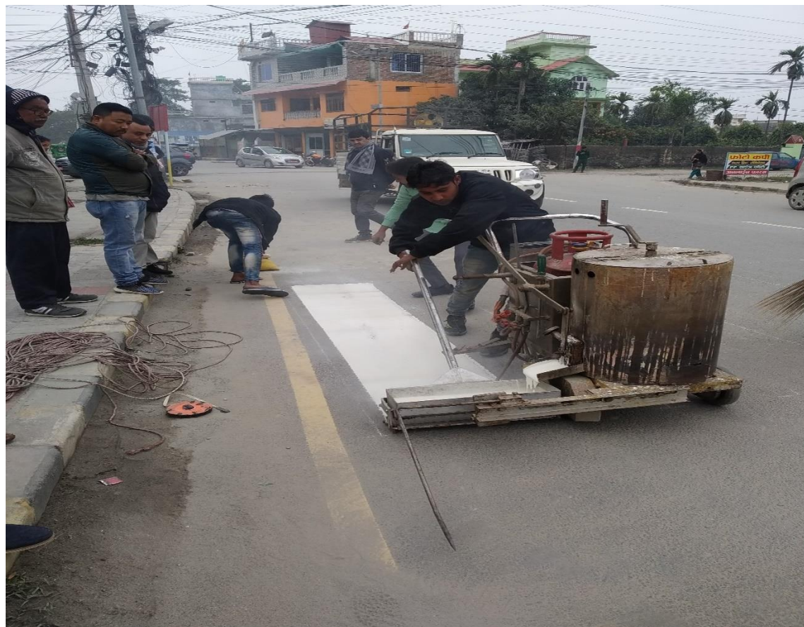
Road painting at R2
