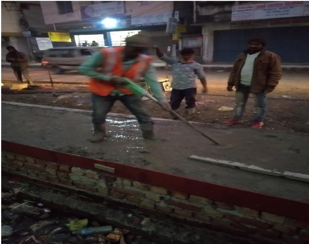
In situ drain cover casting at Rangeli road
