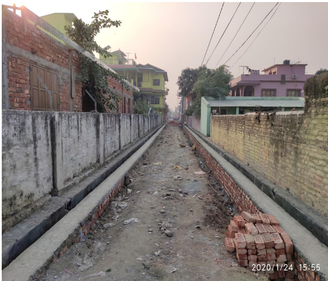
Brick drain at T1L8B (School Marga)
