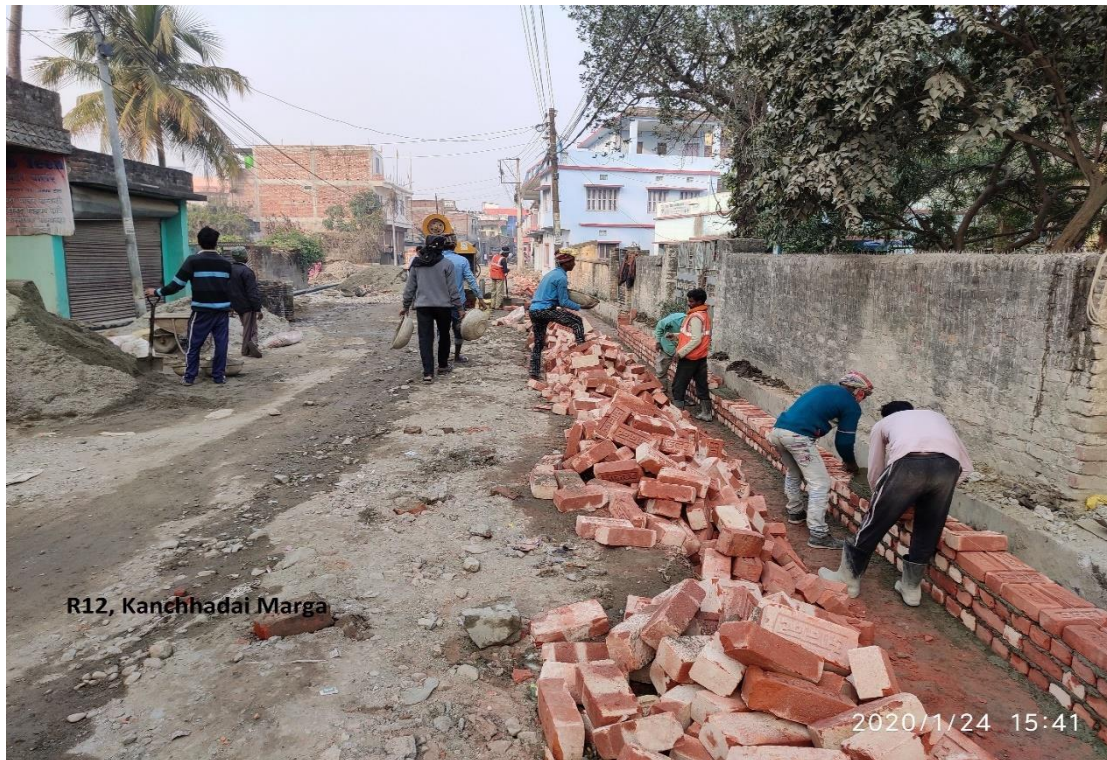
Brick drain at Kanchha dai Marga
