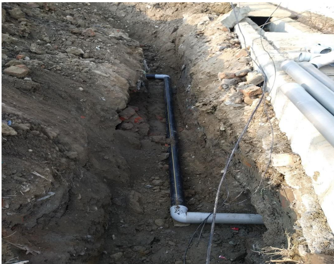
Pipe laying for HCC at R110
