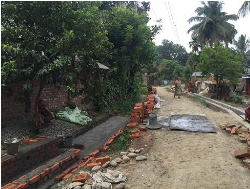
Figure 3. Work in Progress
