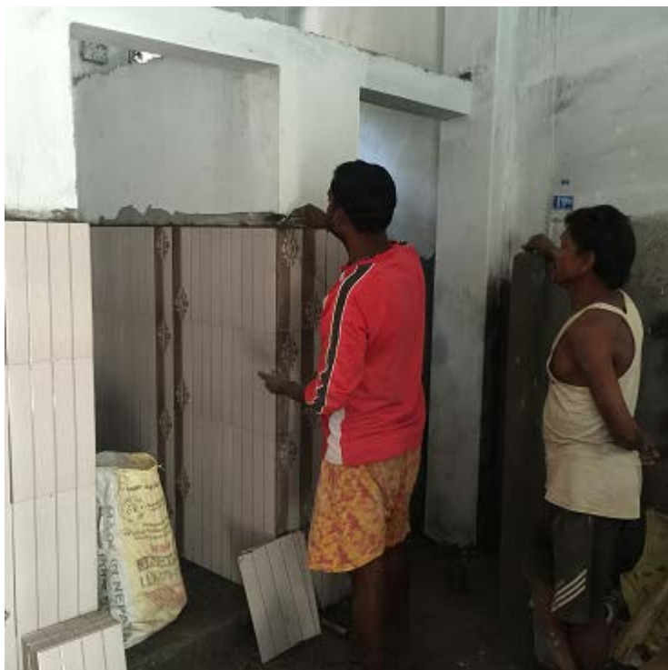
Figure 4. Public Toilet in Koshi Hospital in progress
