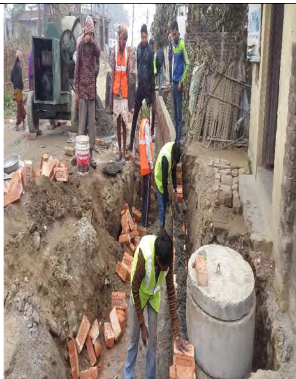
Under Construction of Road side Drain
