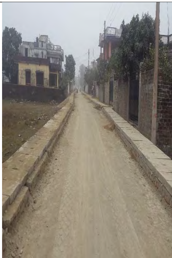
Laying of sub base course for road improvement
