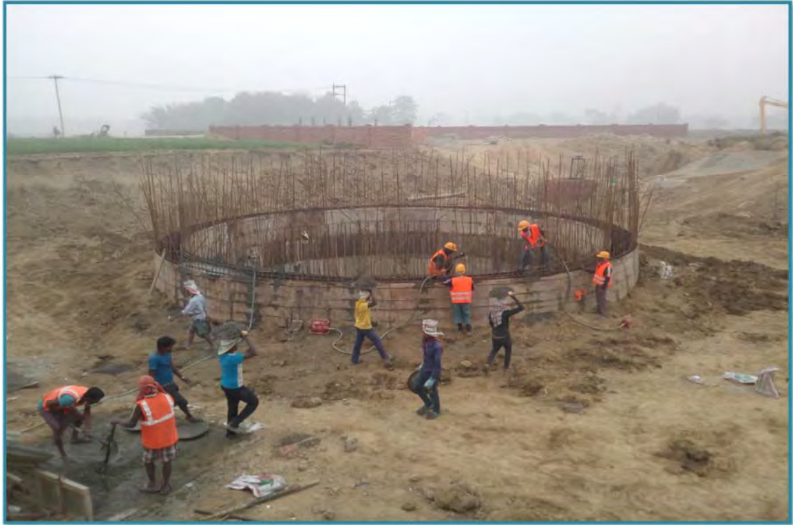
Concreting work sump well
