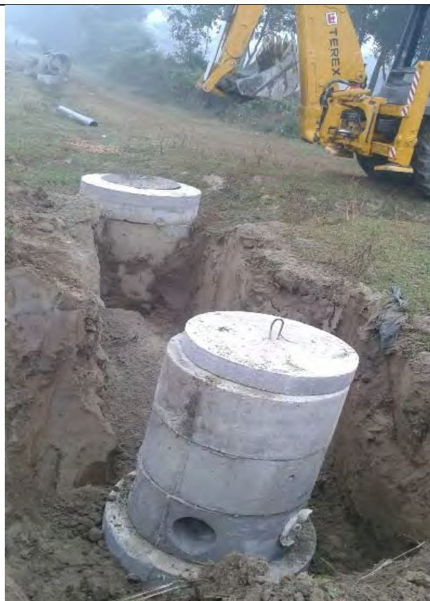
Connection of Manhole and Sewer inlet by uPVC Pipe
