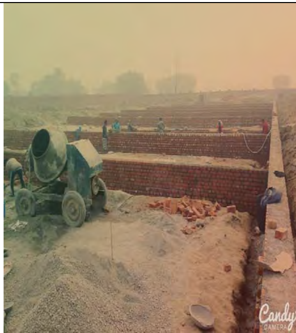
Sludge Drying Bed of WWTP
