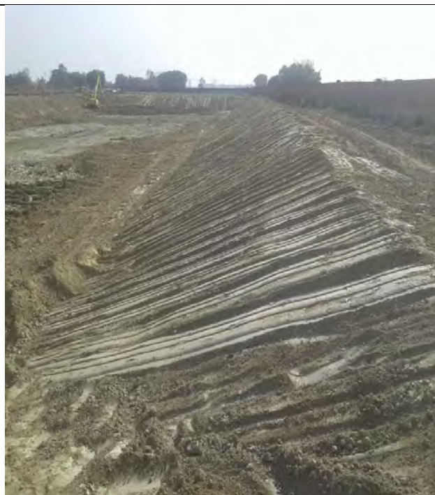
Slope Preparation of Facultative Pond
