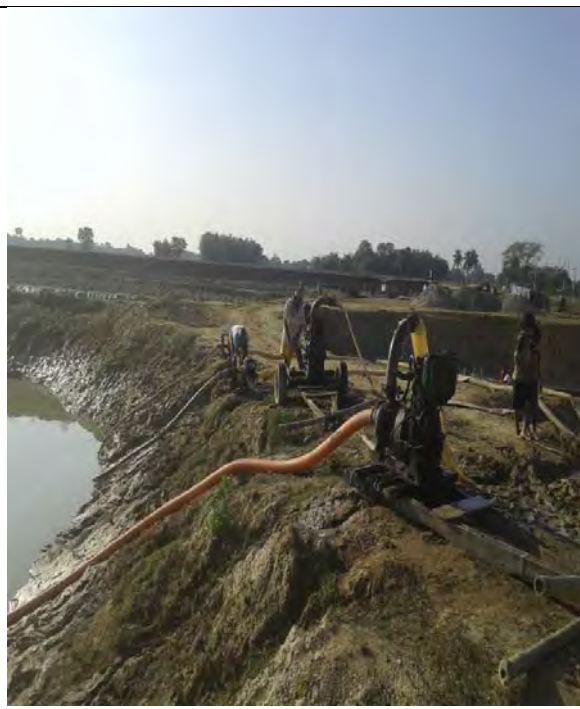
Dewatering of Anaerobic Pond
