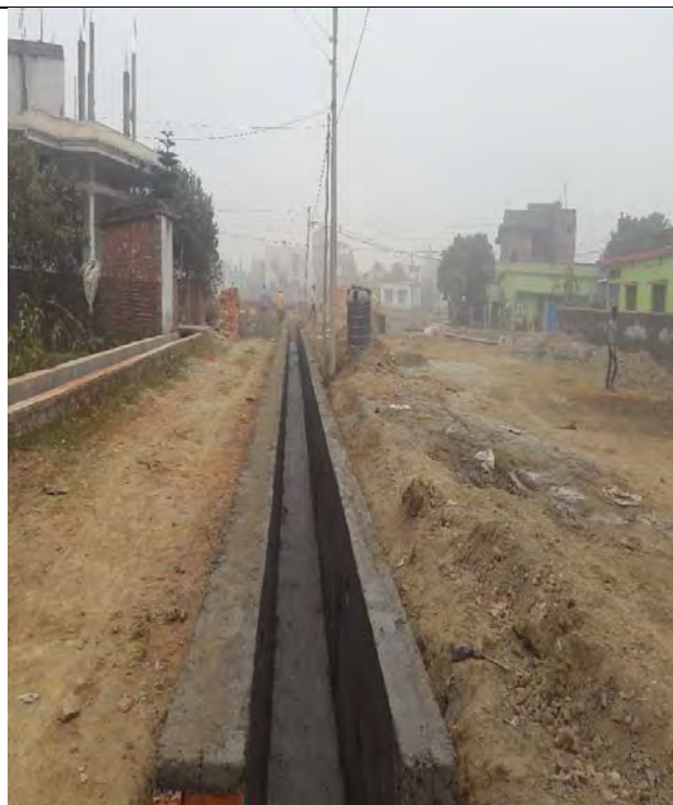
Road side drain with with plaster and punning
