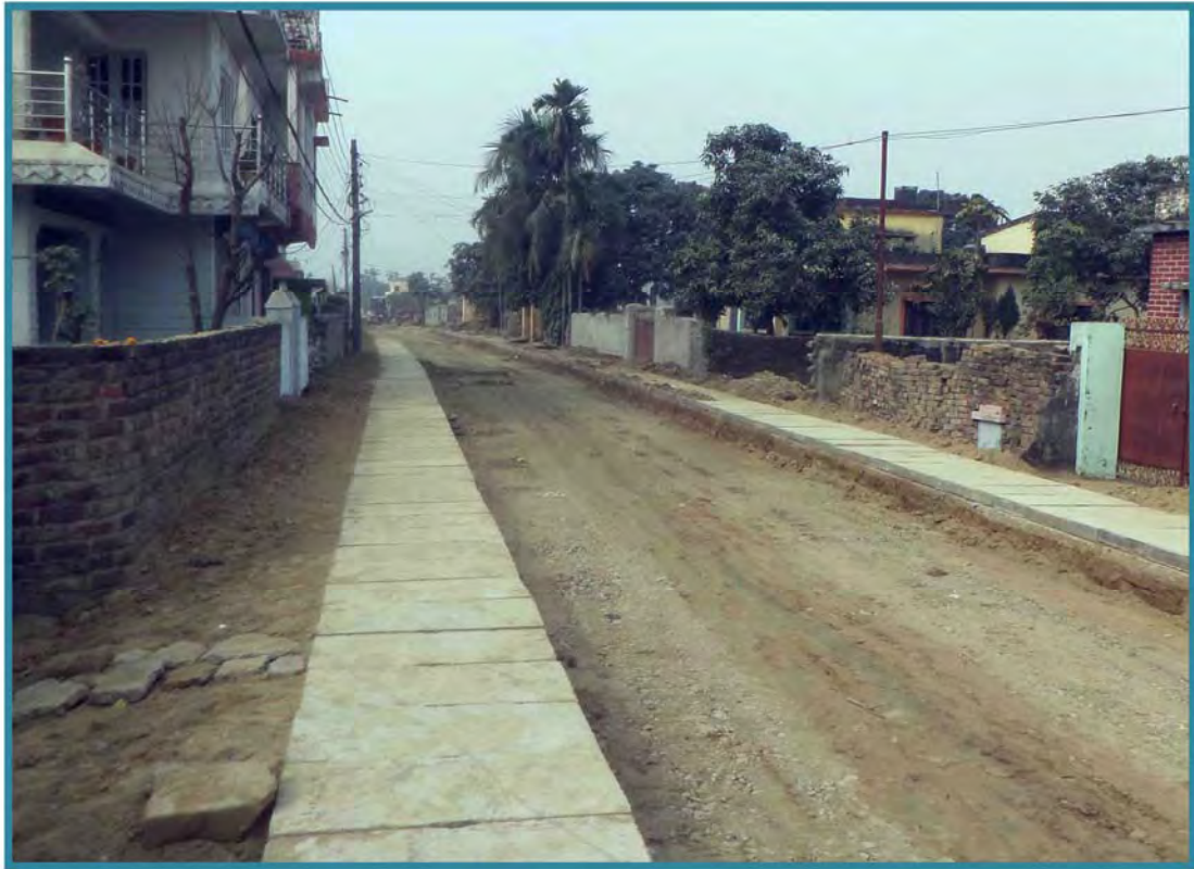
Placing Cover Slabs and Preparation for Sub-Base at R25
