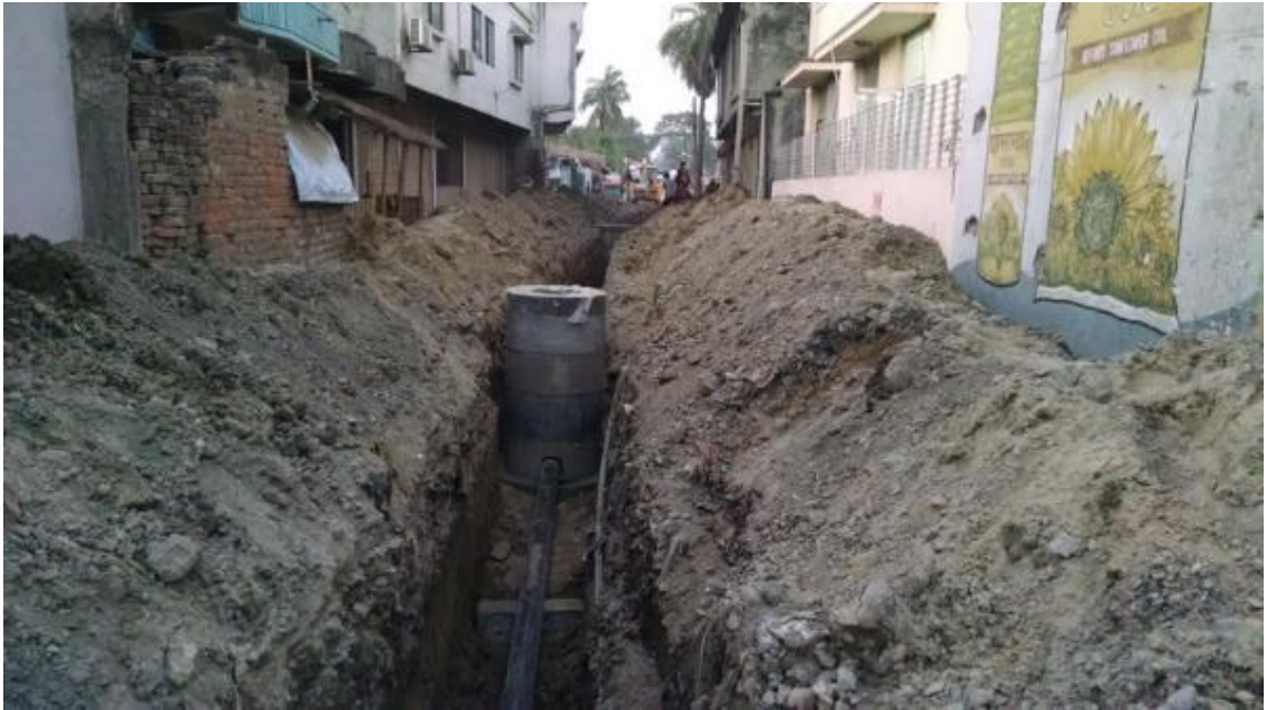
Figure 15 Installation of precast manhole at line 23 (Satghumti)
