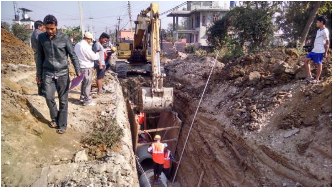
Figure 17 Installation of 700 dia Hume pipe at line T3, Yadhav Chowk
