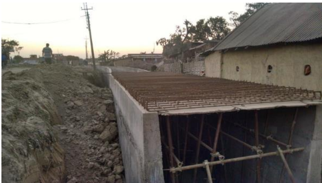
20. Reinforcement laying for RCC slab at line B3
