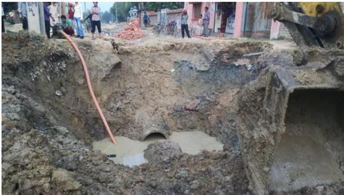
Figure 3 Dewatering of manholes
