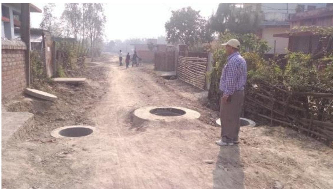
Figure 14 Observing precast sewer inlet and manholes at line 33
