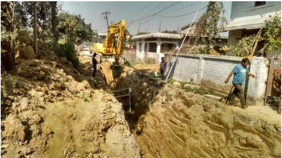
Figure 16 400 dia Hume Pipe laying at secondary line T2L19
