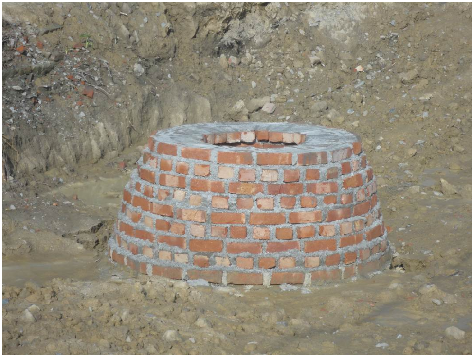
Complete Brick Masonry Manhole at T2 (Near National Trading Office)
