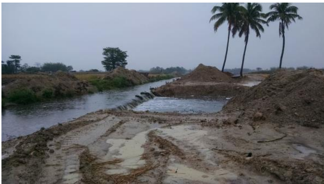
Figure 8 Heavy rainfall cause raise of water level at Dharamband Nala causing overflow to manhole pit
