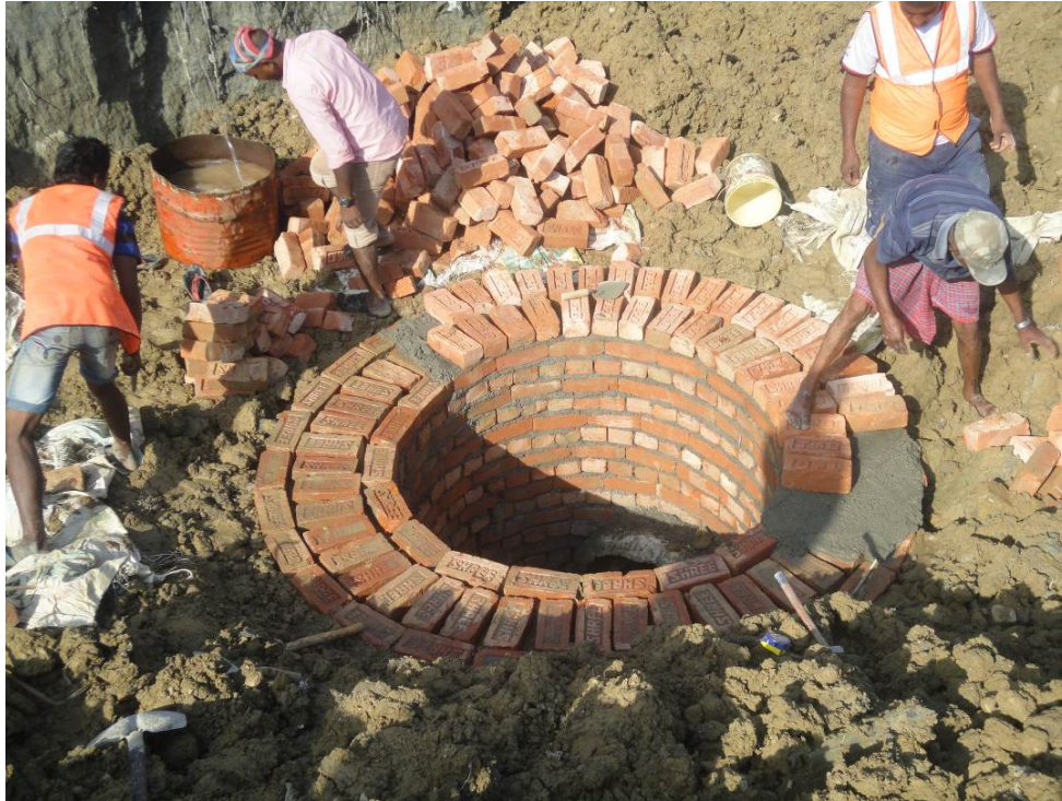
Brick Manhole under construction at T2 (Near National Trading Office)
