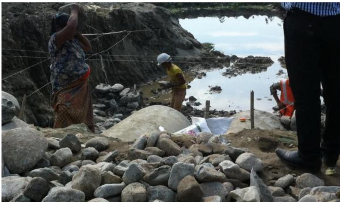
Figure 25 Outfall Structure construction at S11
