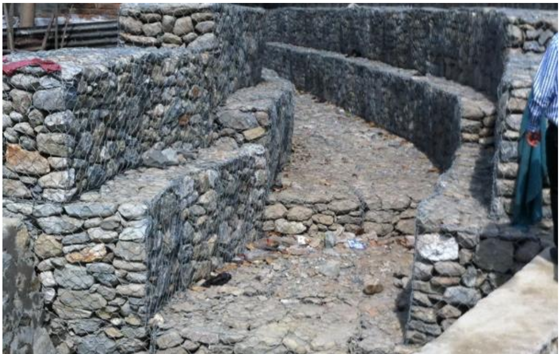
Figure 24 Outfall structure at S11
