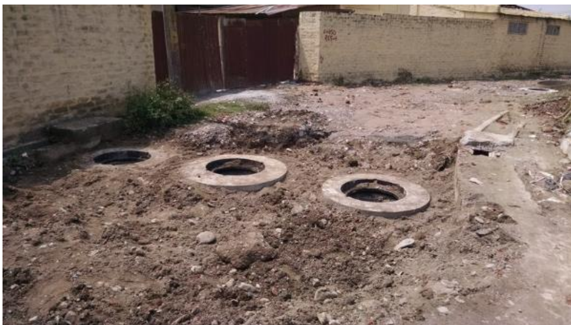
Figure 6 Manhole and Sewer Inlet at line T2L24A( Satghumti)
