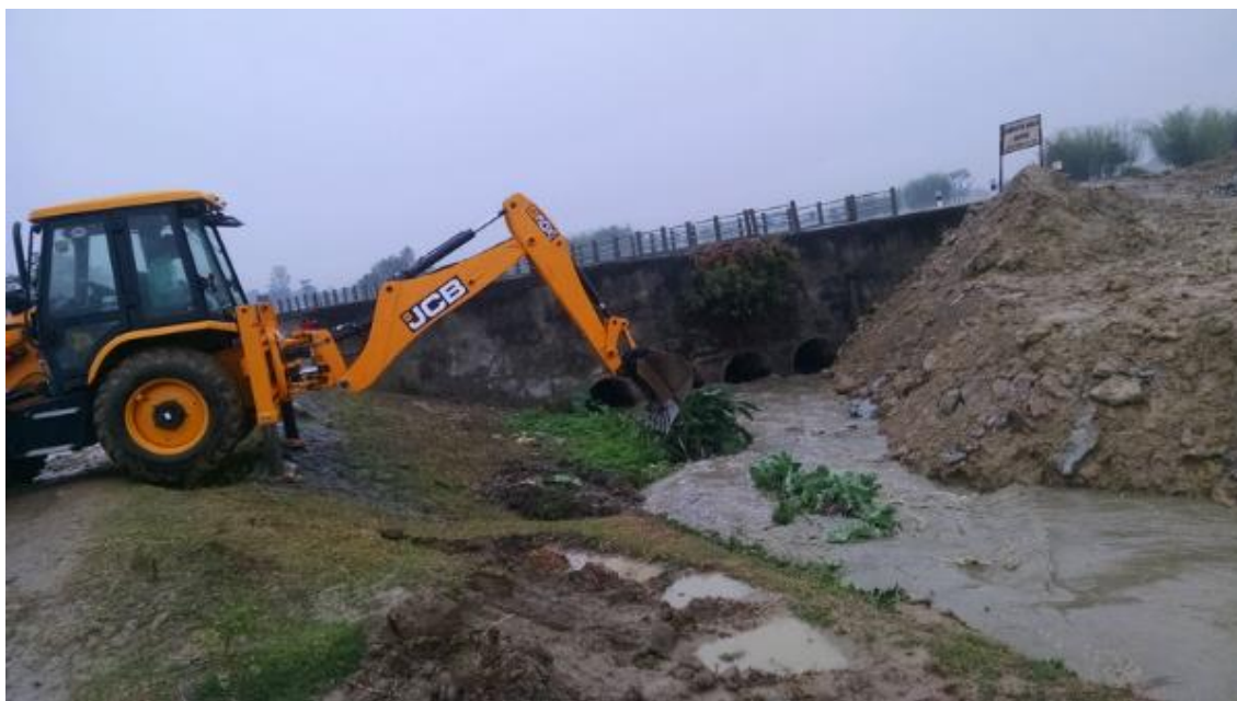
Figure 7 Diversion of existing canal
