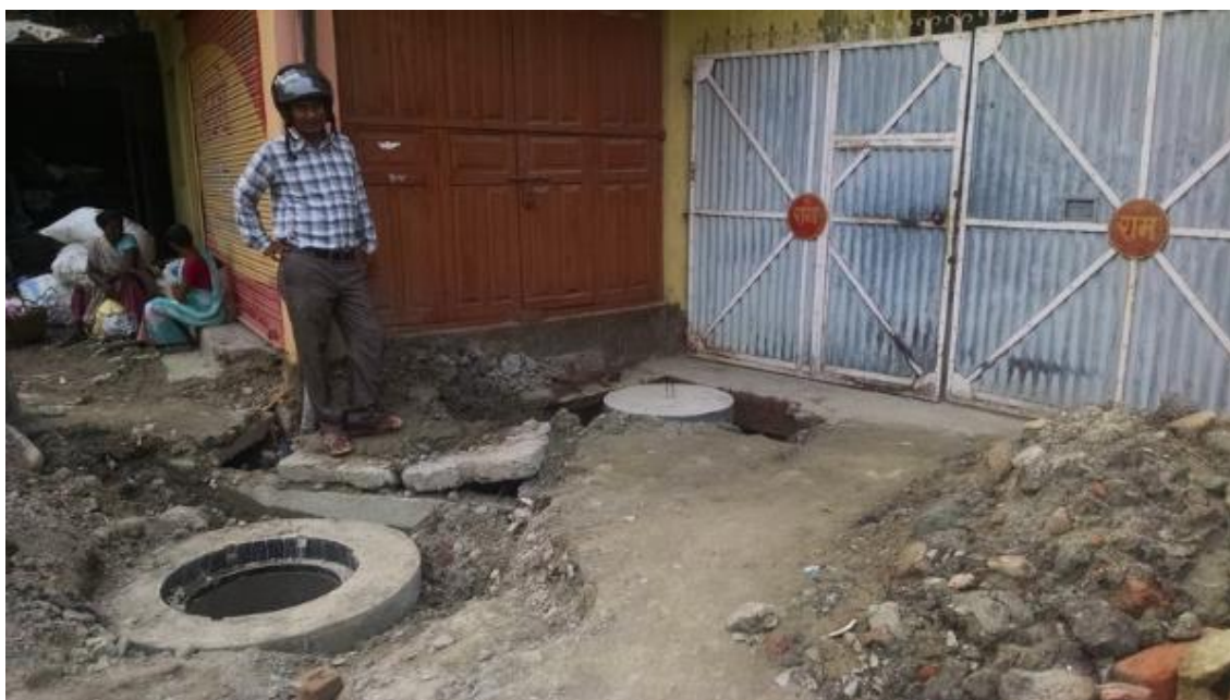
Figure 4 House Connection Chamber and Sewer Inlet at Line T2L24A (Satghumti)
