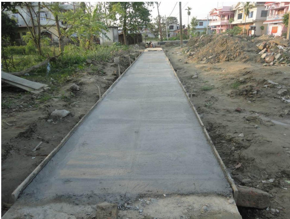
RCC Cover Slabs for storm drain S11 at West side of Pushpalal Chowk
