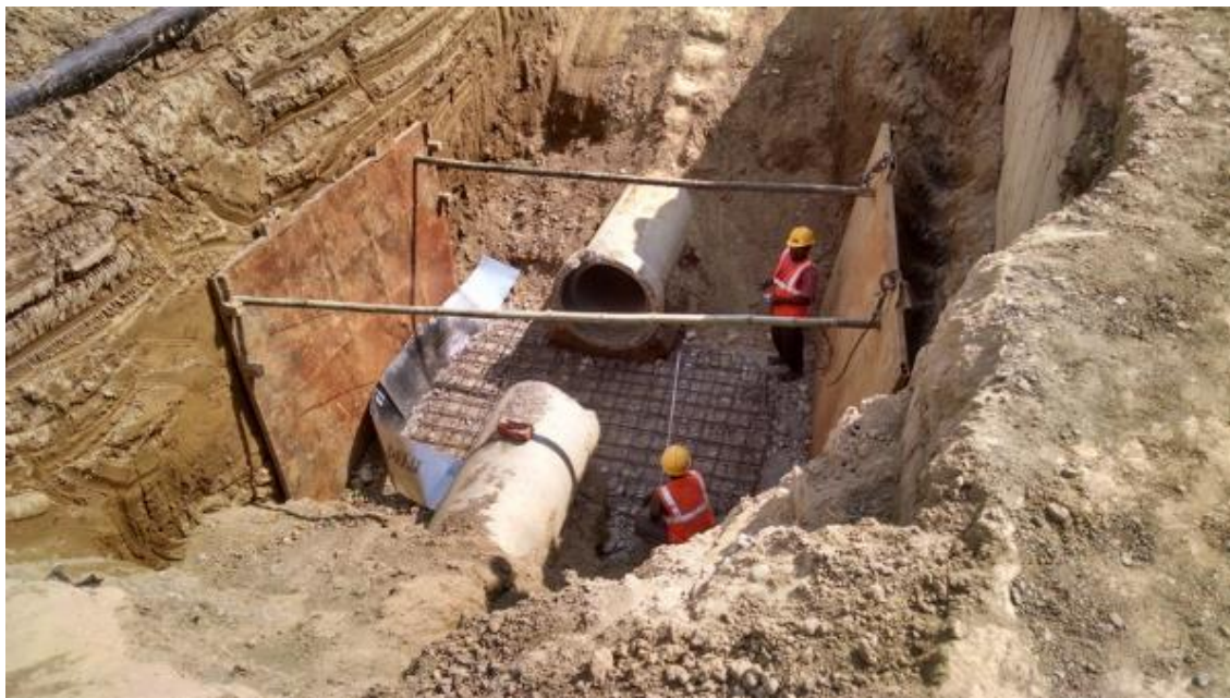
Figure 11 Manhole bottom RCC at Line T2, Jatuwa
