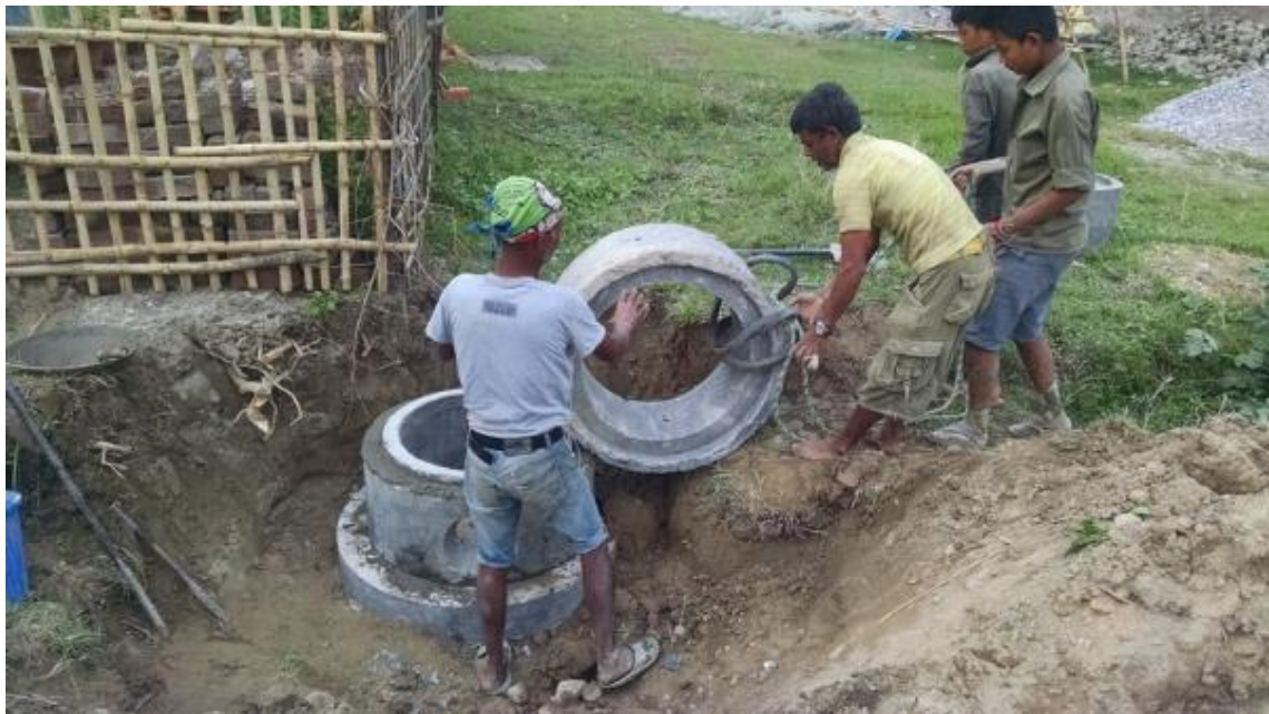
Figure 1 Installation of Precast Sewer Inlet Chamber
