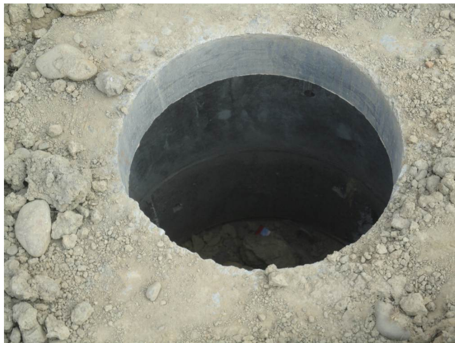
Precast manhole installed at site
