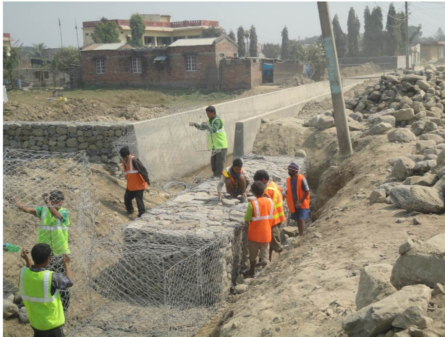
Outfall structure at B3 in progress
