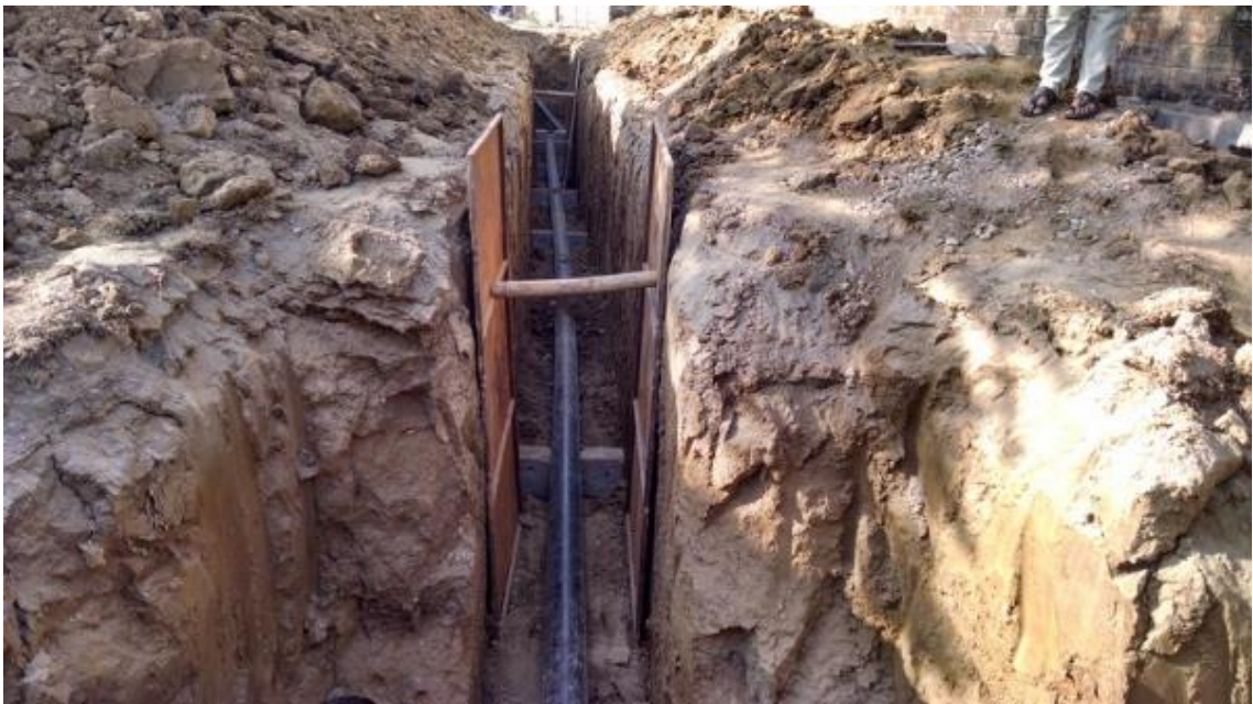
Figure 18 HDPE pipe laying at line T3L26
