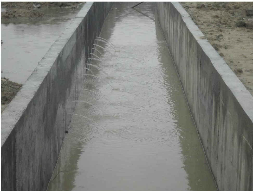
Well function of weep holes observed during rain on 26-27 March 2015, completed Storm drain at B2
