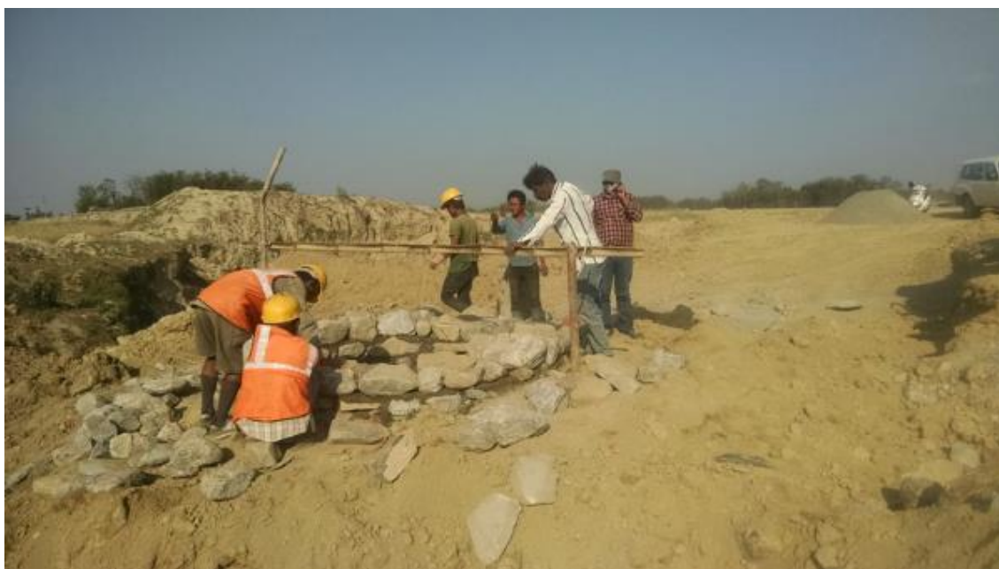
Figure 12 Stone masonry works at line T2, Jatuwa
