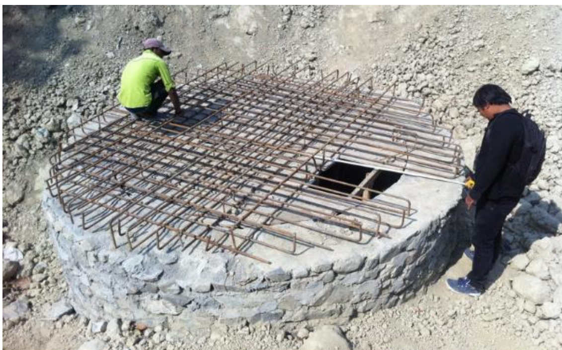
Figure 26 RCC Slab construction for manhole at S13
