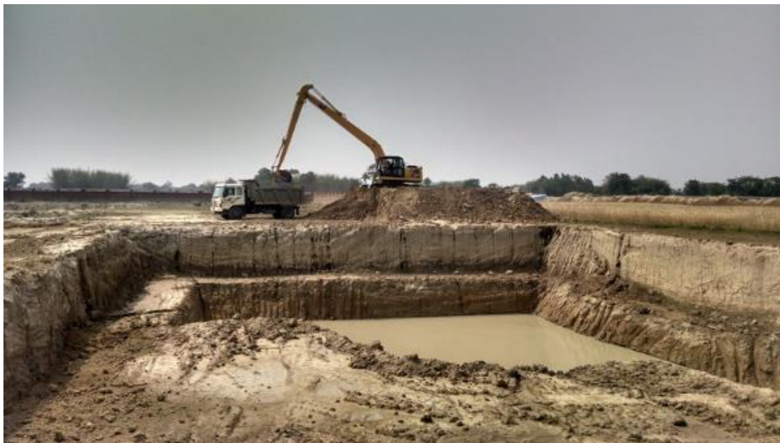
Figure 5 Excavation of Sump well
