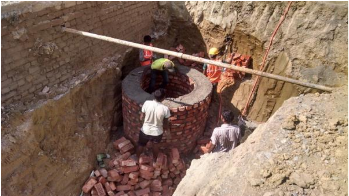
Figure 10 Manhole construction at line T2L19
