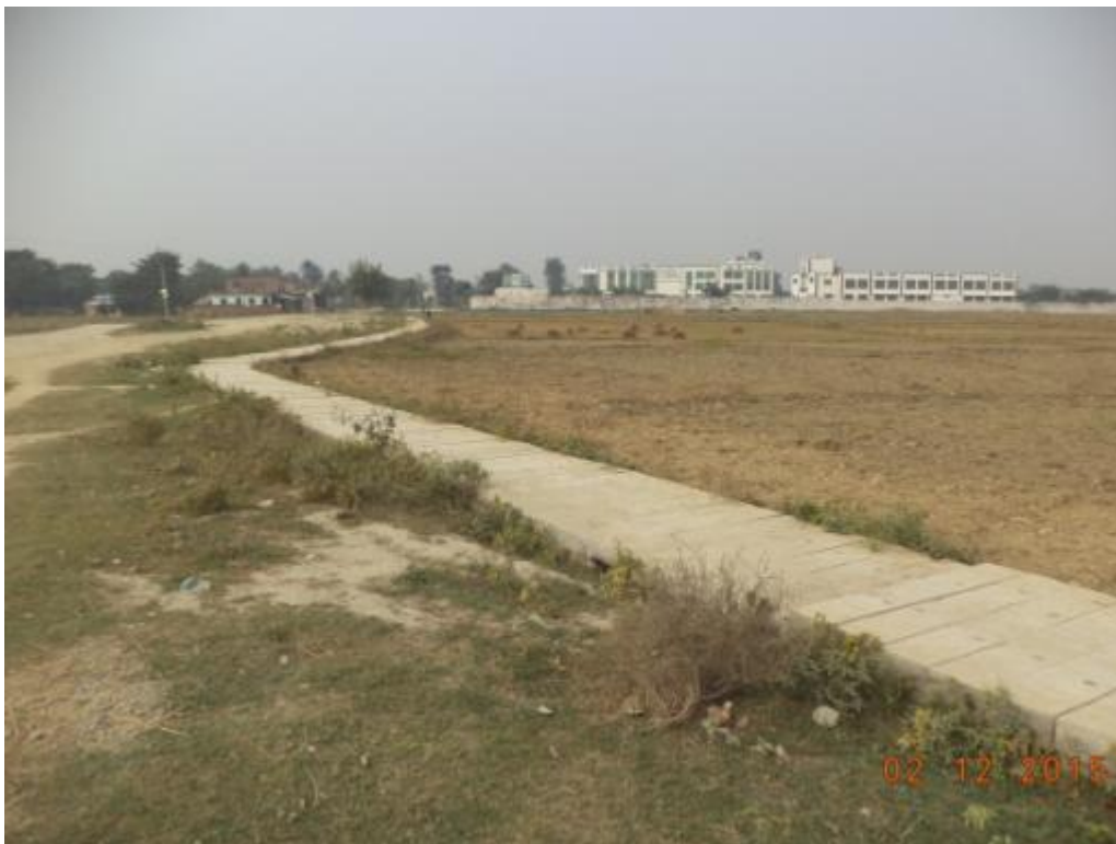
Condition of Storm drain at B2 L1 after monsoon and festival
