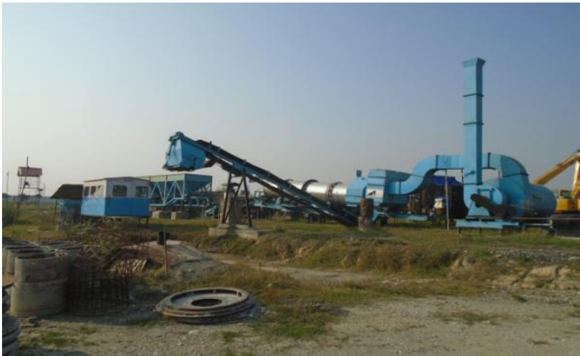
Figure 2 Asphalt plant and other equipment remain idle due to strike
