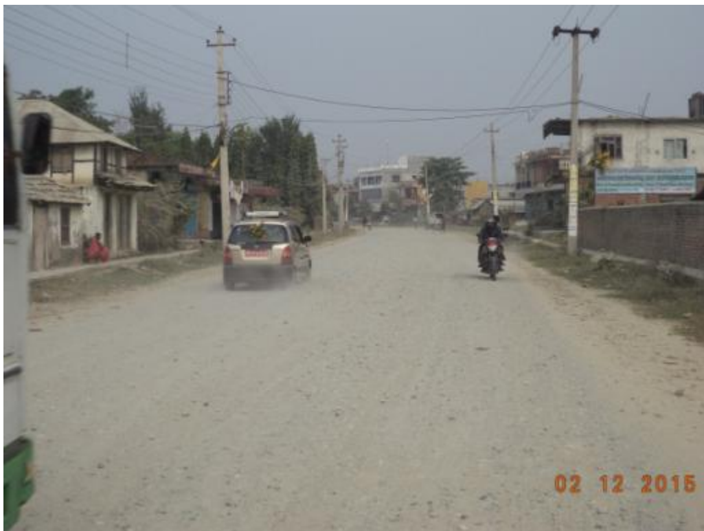
Good condition of gravel road surface after monsoon and festival at Pushpalal Road ( A part of R2 Road)
