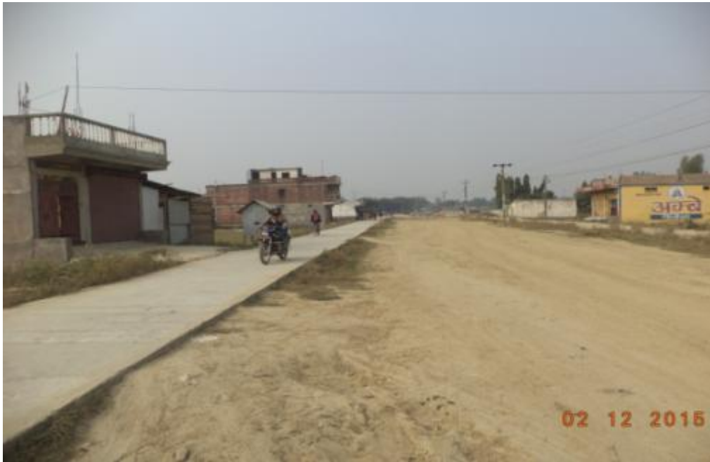
Condition of Storm Drain after monsoon and festivals at B3 L2
