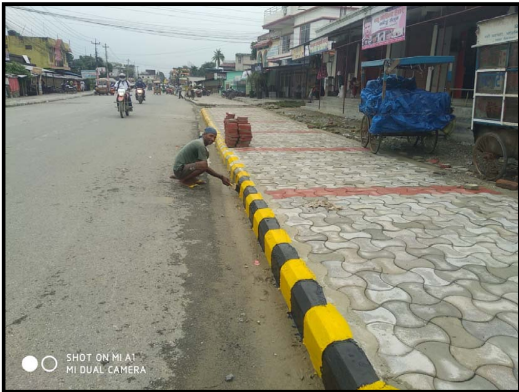
Footpath finishing works at B2
