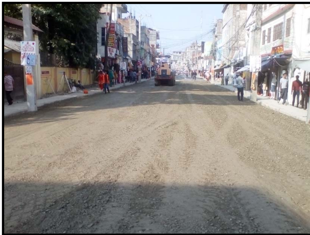
R2 Lane – Base laying
