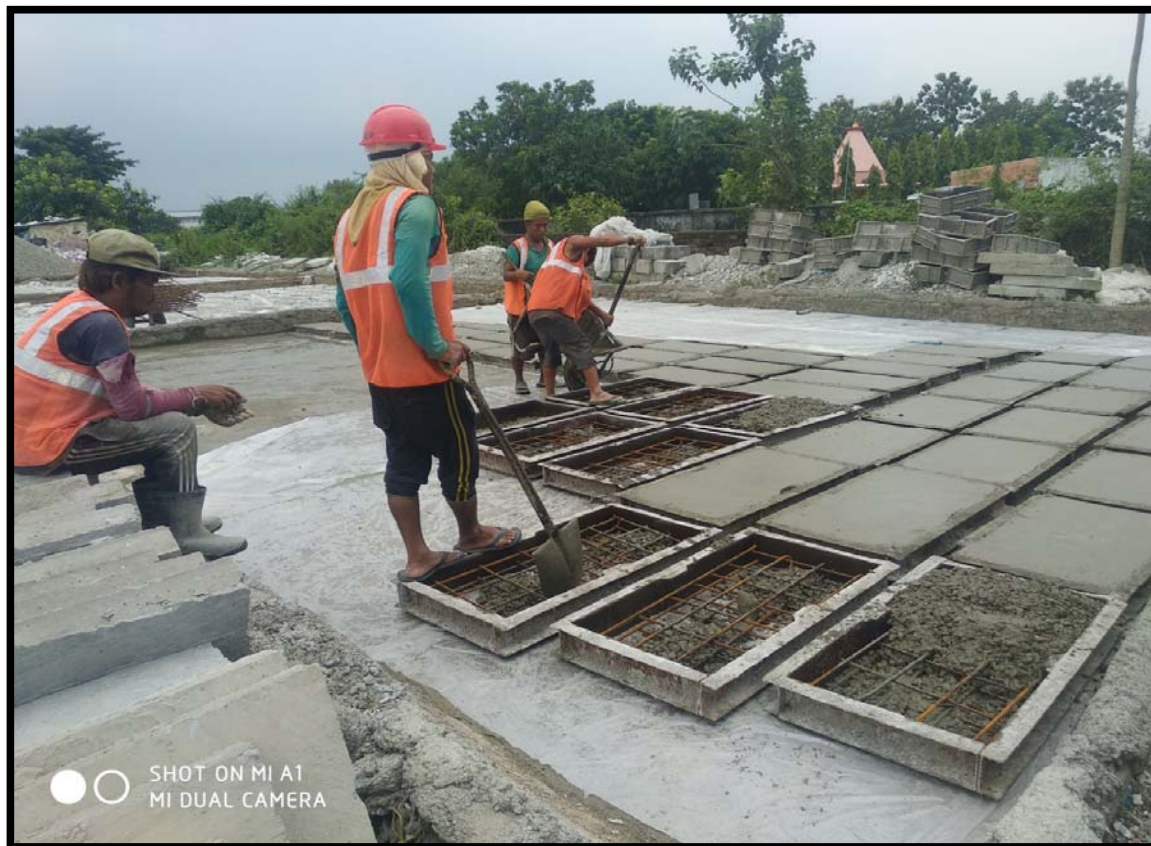
Precast element's casting at Contractor's yard
