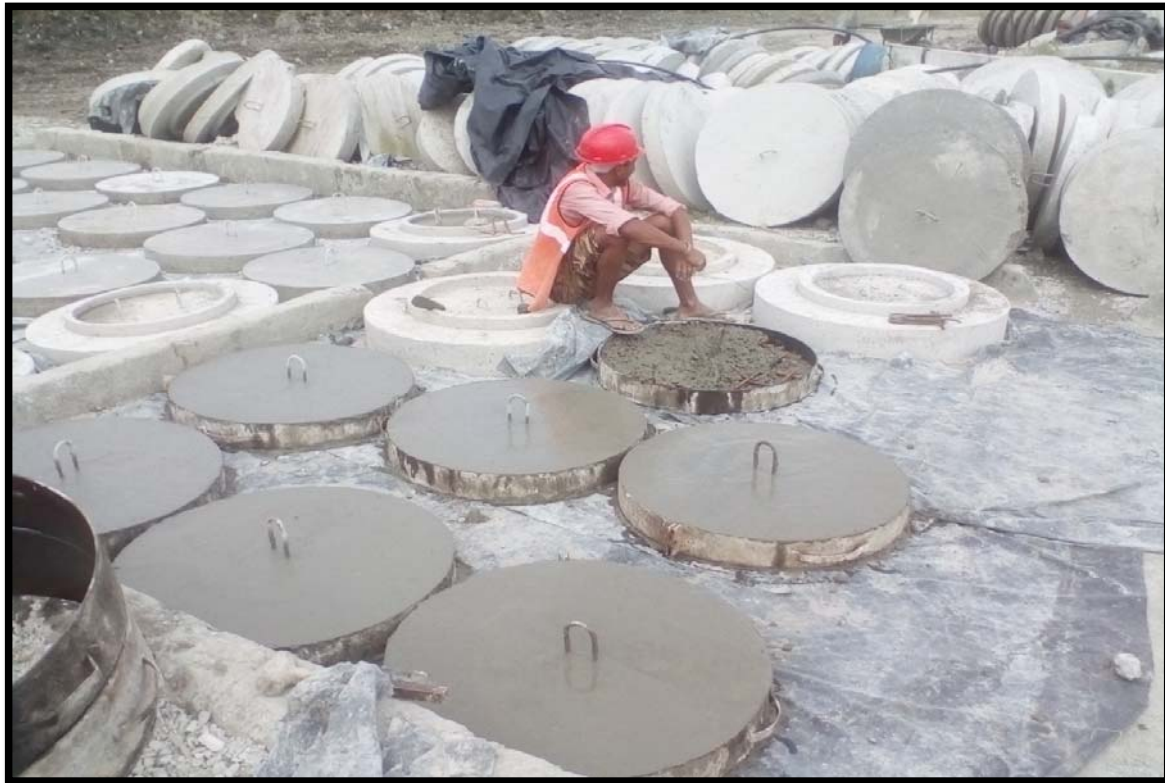
Precast element's casting at contractor's yard
