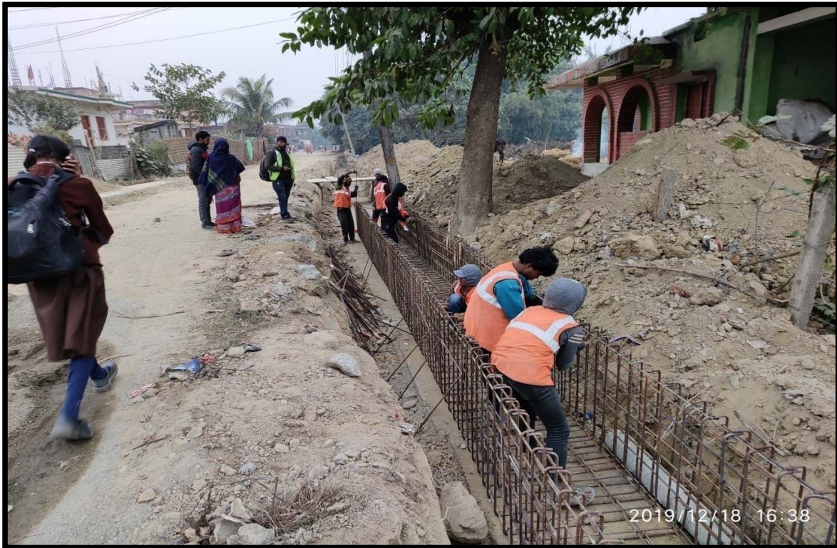
RCC Drain at R4 near N2 Junction
